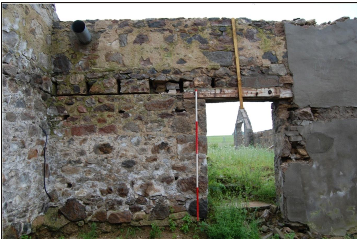
Illus 12 North end east wall Room 2 with D10 showing beam slots
