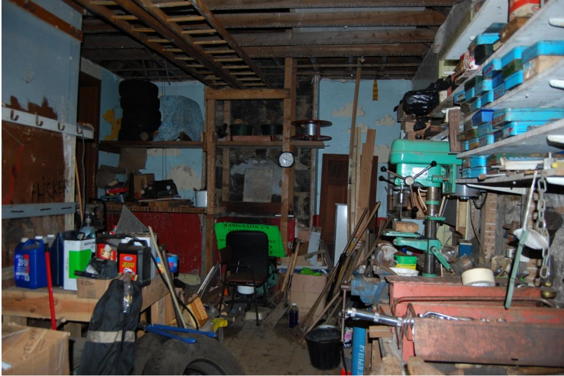
Illus 7 Building 4 facing NE showing original chimney breast and fireplace (centre)
