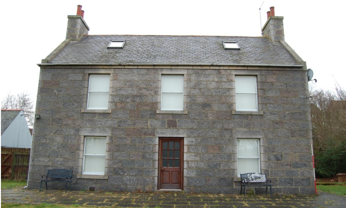
Illus 4 Building 1 the farmhouse; facing NE
