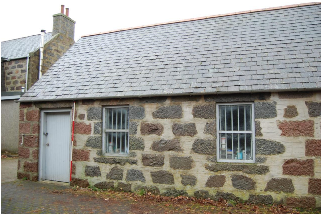
Illus 5 Building 2; facing SW
