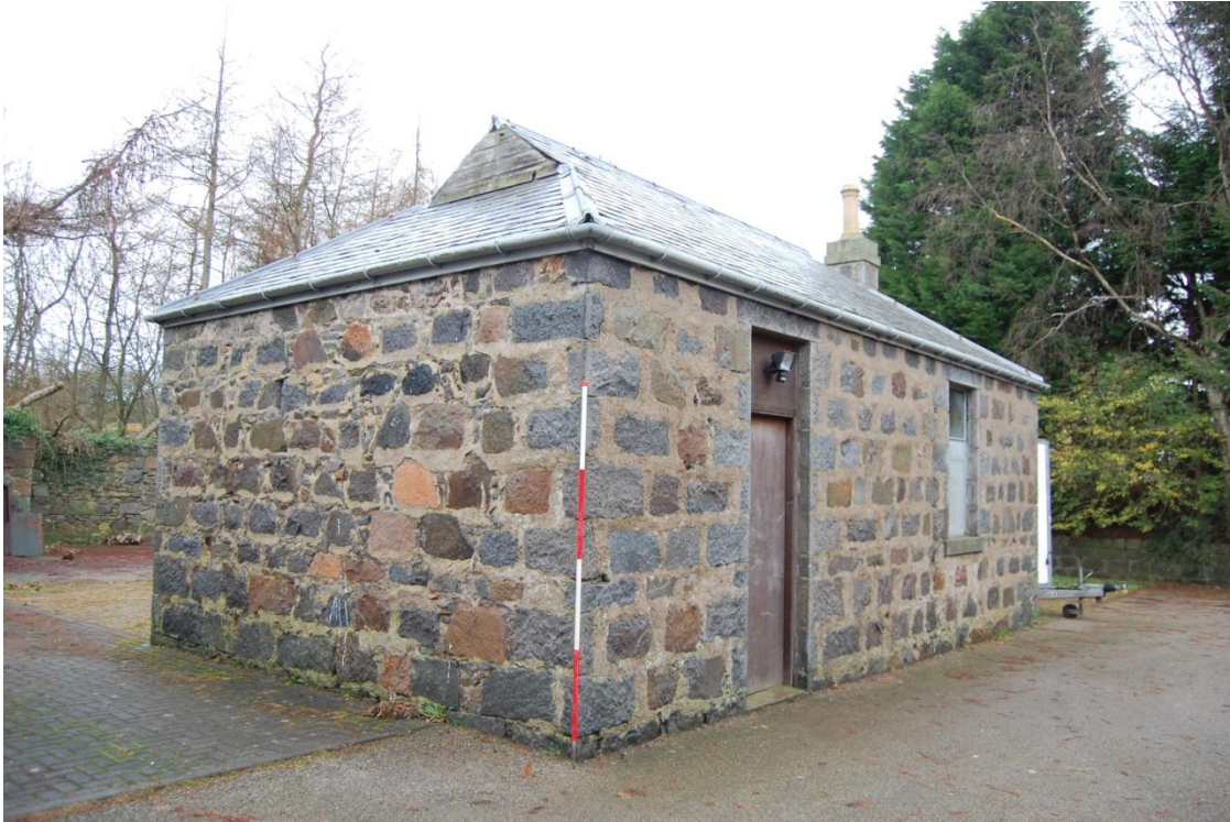
Illus 6 Building 4; facing NNE
