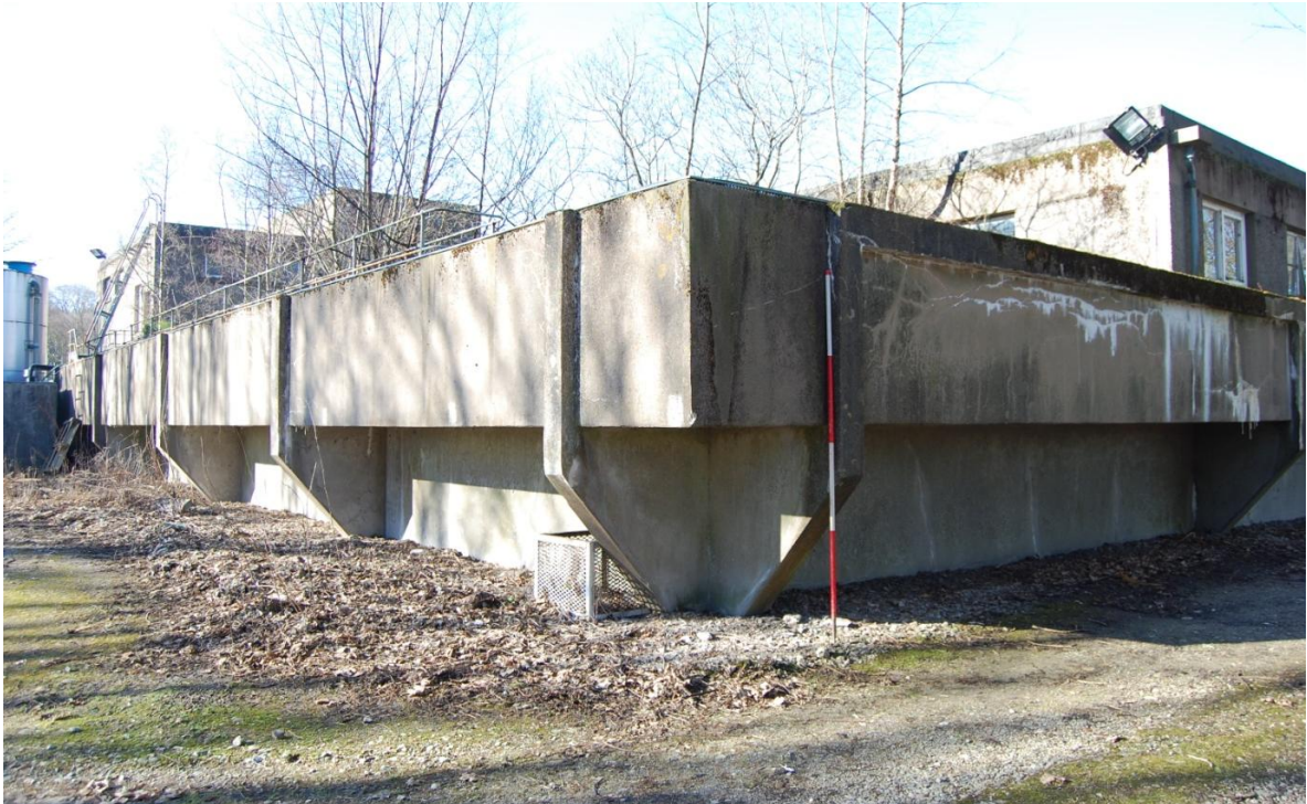
Illus 18 Building 30A section to be demolished facing W
