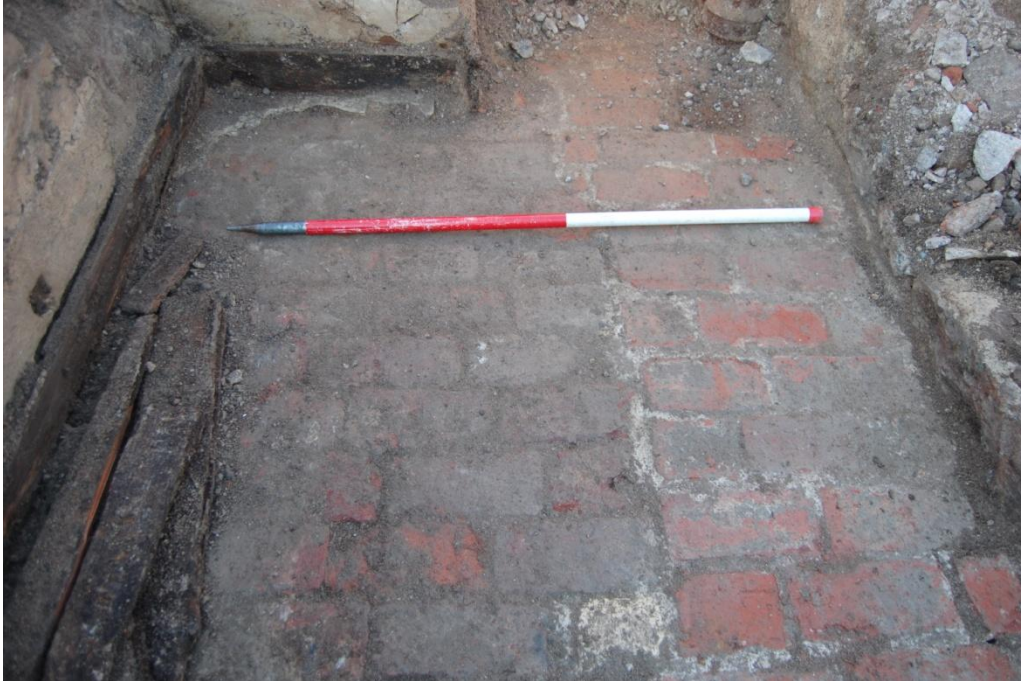
Illus 8 Duct or inspection pit F10 was originally constructed in stone and mortar with a brick floor; it was altered in the late 19th-century and a poured shuttered concrete wall added (left)
