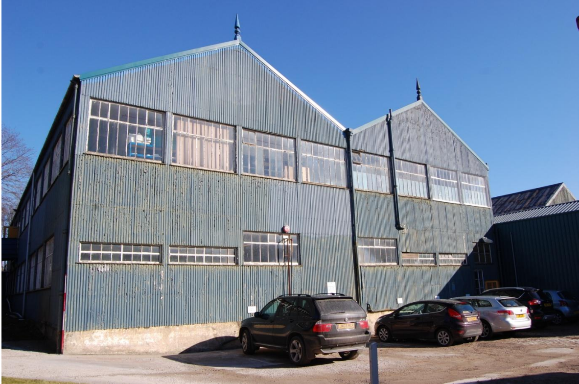
Illus 17 Building 30 SW facade
