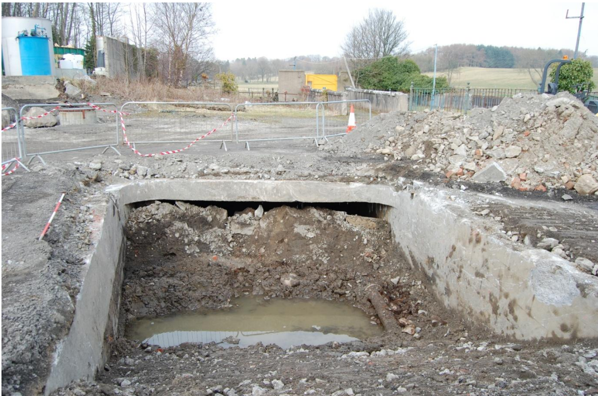
Illus 12 concrete lade intake F55 facing NE
