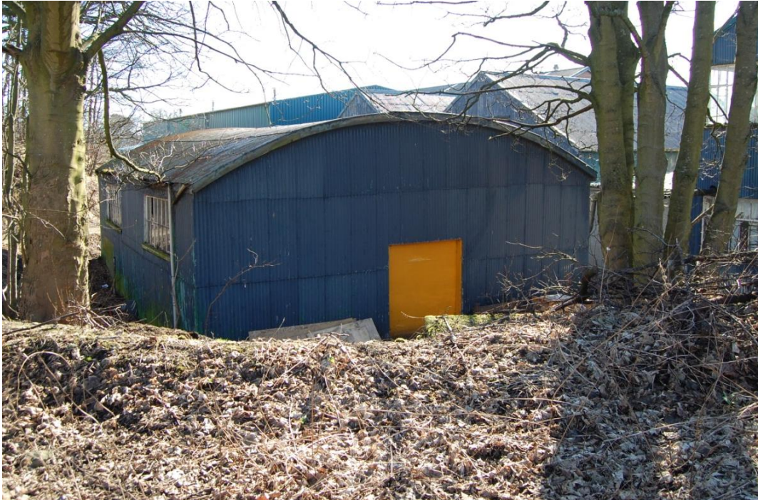
Illus 19 Building 31A facing SE
