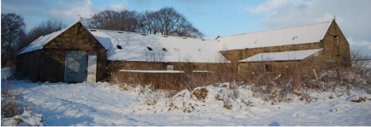
Illus 13 Building 3 (left and centre) Building 2 (right); facing NW
