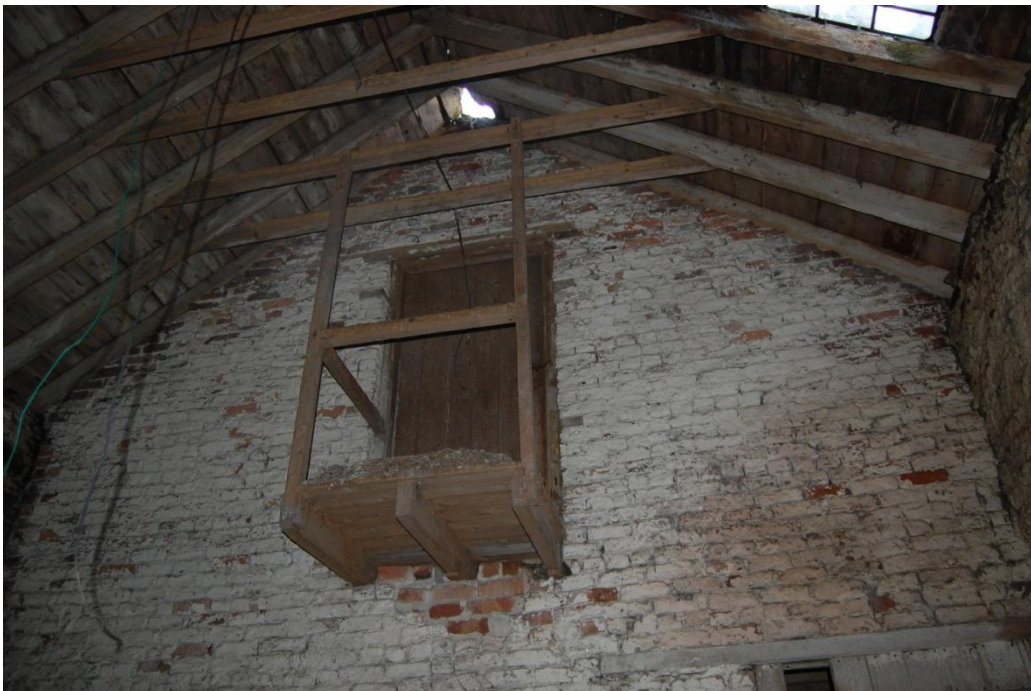
Illus 16 East wall of cartshed showing first floor door and wooden balcony facing E
