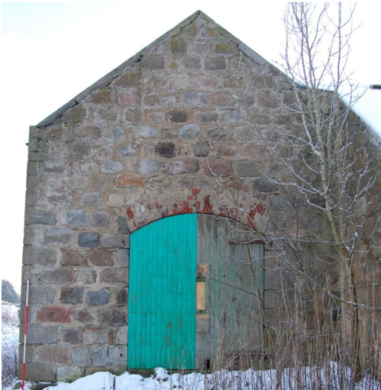
Illus 14 Building 2 Door 15 exterior; facing E
