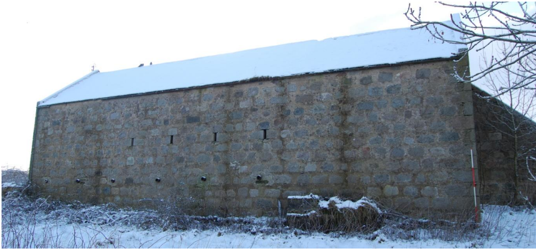
Illus 17 Building 2 north wall with ventilation holes; facing SSE
