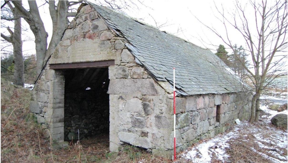
Illus 8 Building 1 south gable showing Door 2 a modern insertion; facing NNW
