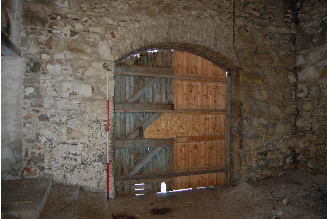
Illus 15 Building 2 Door 15 interior; facing W
