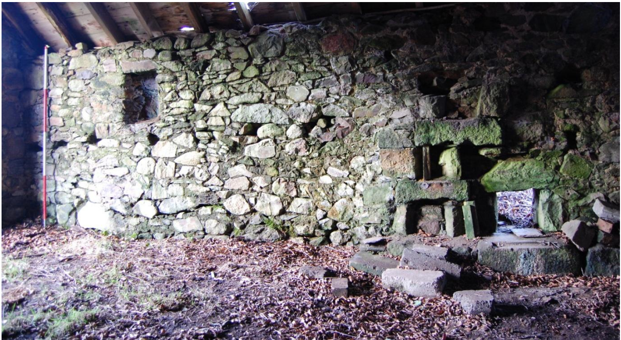
Illus 9 Building 1 interior of west wall showing sockets F108 (left) and apertures for mill mechanisms (F102, F103, F111, F112 right); facing SW
