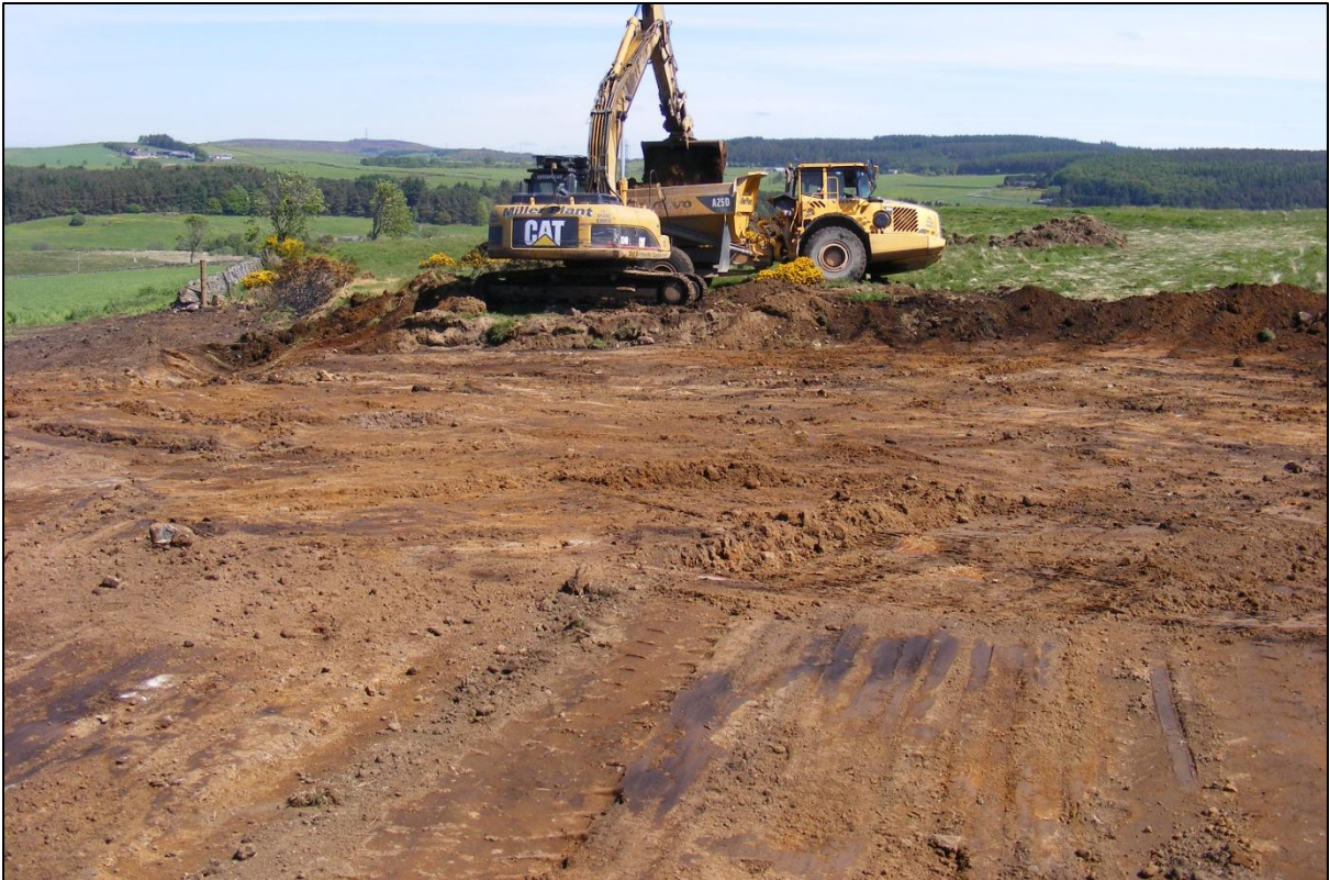
Plate 3 – View of turbine base during excavation facing N.
