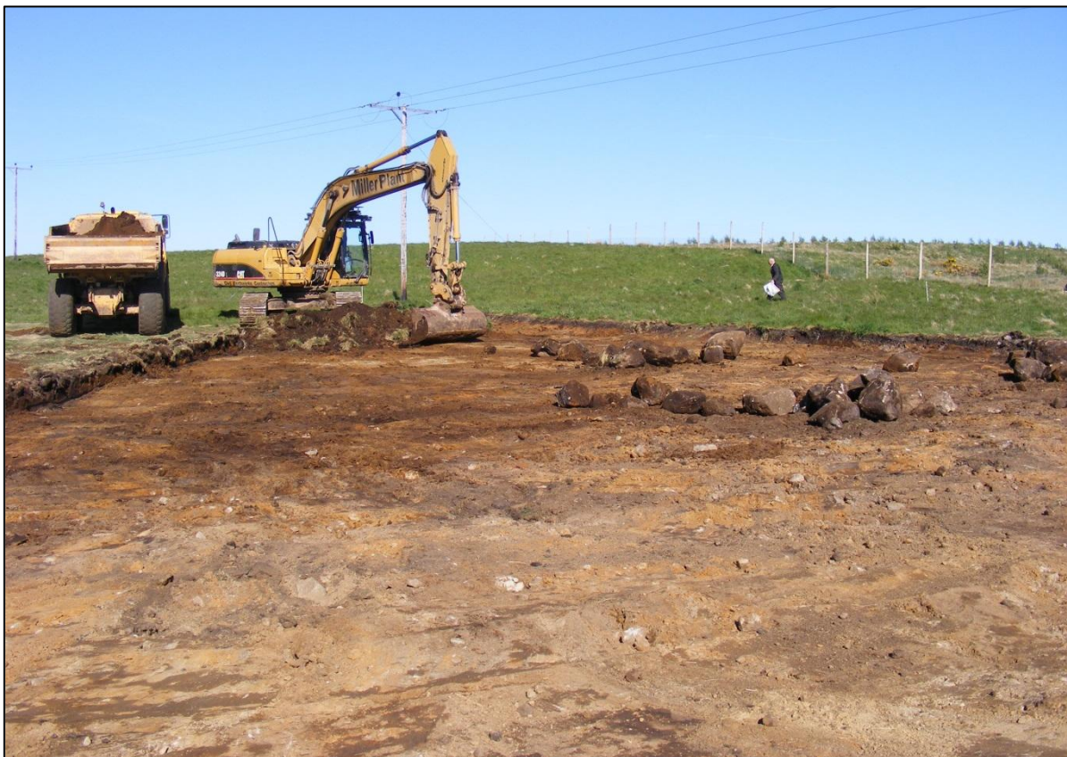
Plate 4 – View of crane pad during excavation facing NE.
