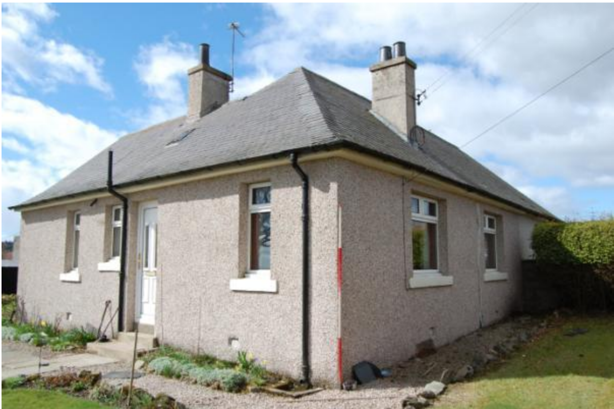
Illus 7 Building 1 No 7 Whitemyres Holdings facing NW
