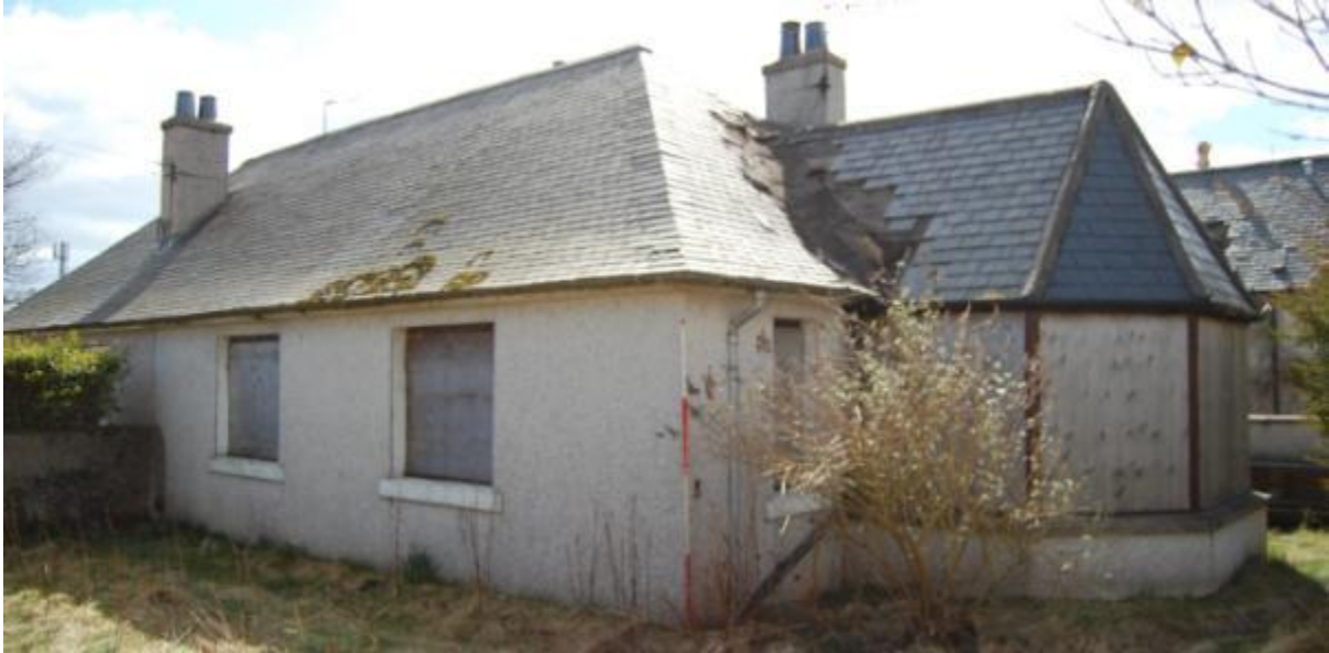
Illus 11 Building 4, 8 Whitemyres Holdings facing SE
