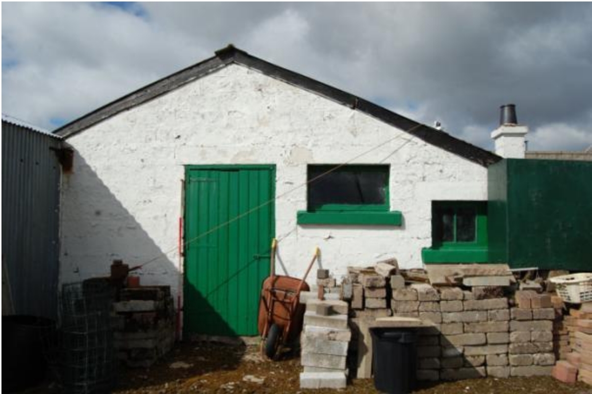
Illus 8 Building 2 shed of 7 Whitemyres Holdings, facing W
