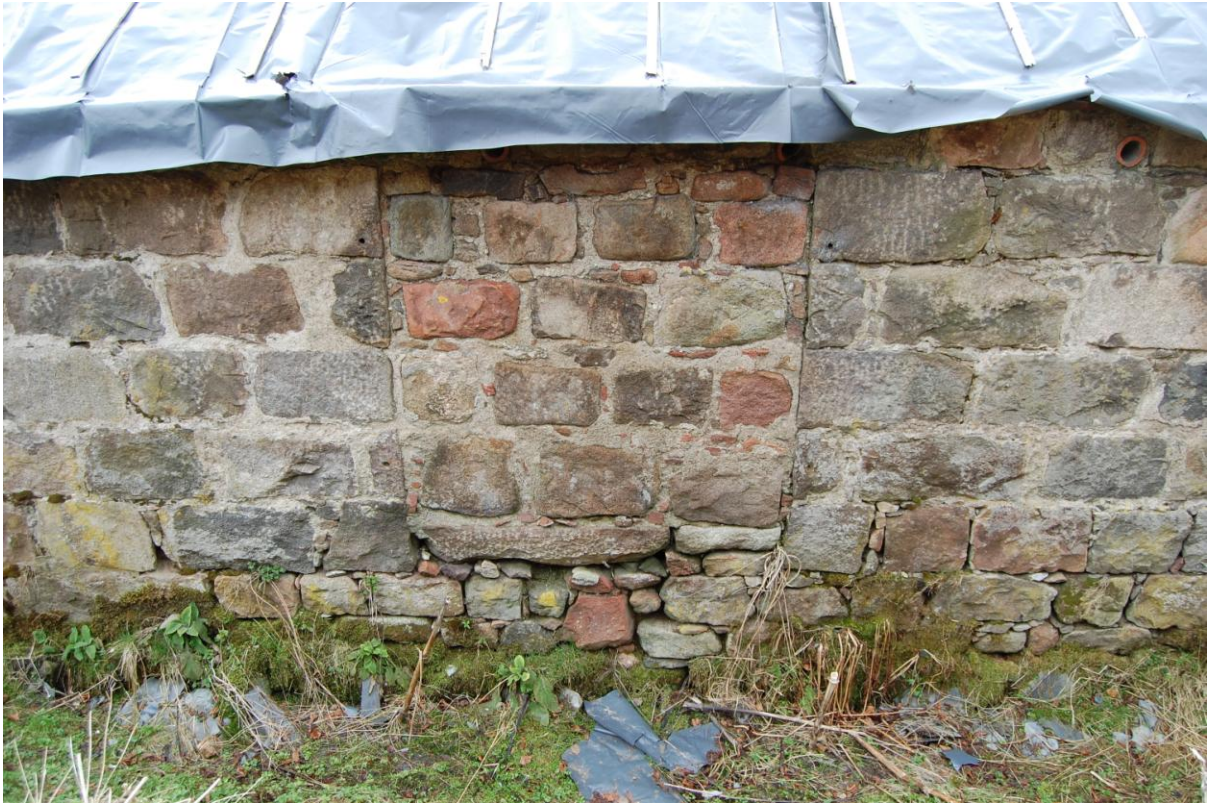
Illus 8 Room 2 north wall showing blocked door; facing south.
