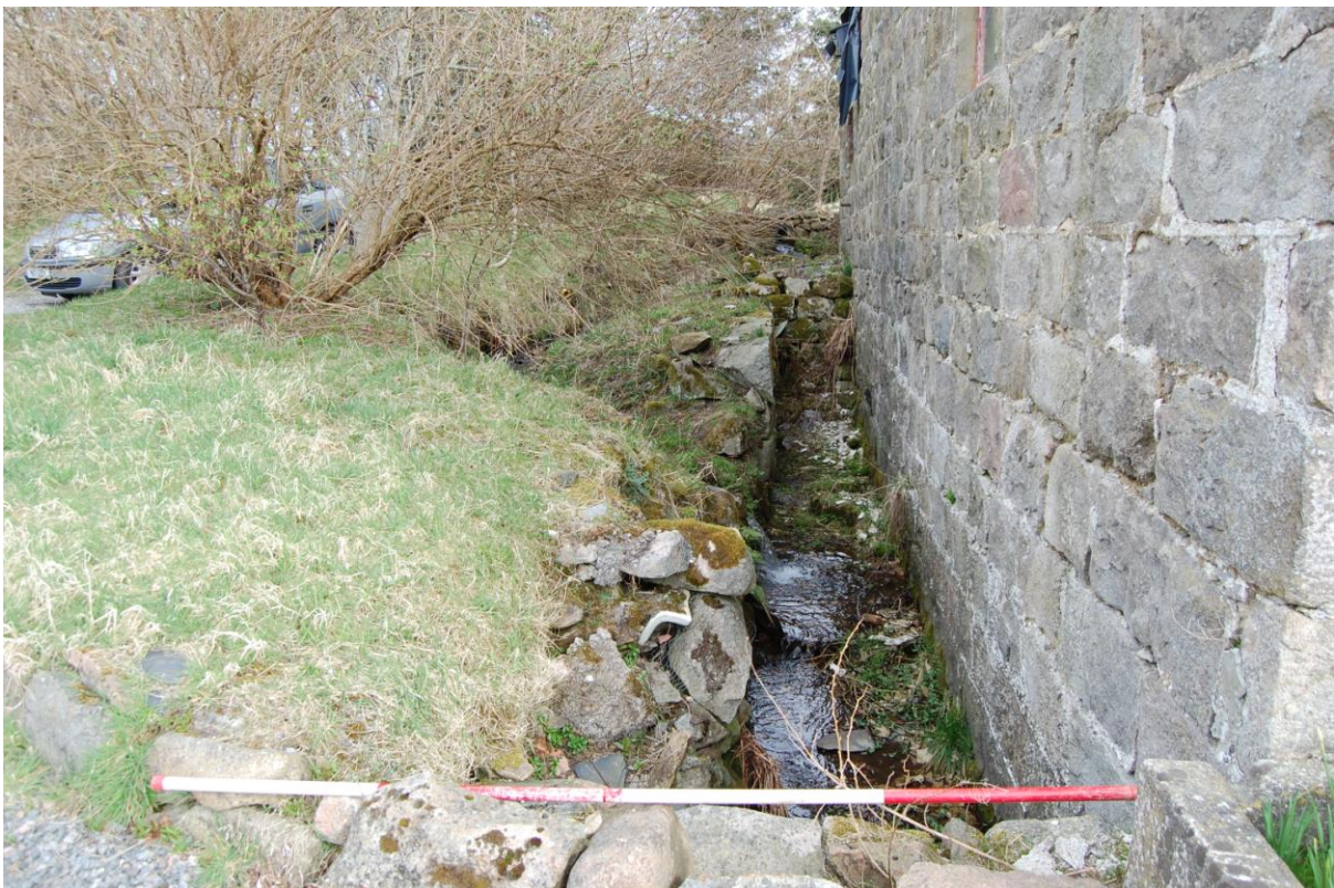
Illus 7 Room 3 west wall showing mill race and stream; facing north
