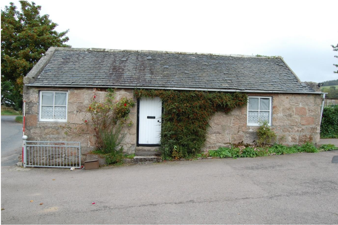
Illus 5 South-facing facade
