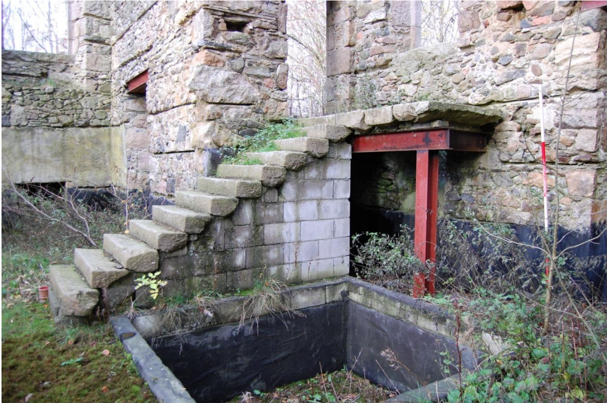
Illus 9 Stairs to lower ground floor basement; facing NW.
