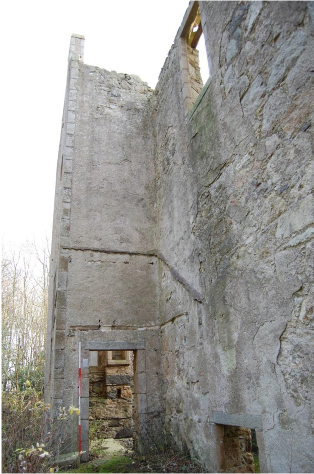
Illus 12 Extension to exterior of north wall with rear back door and scars showing lean-to extension above'; facing east
