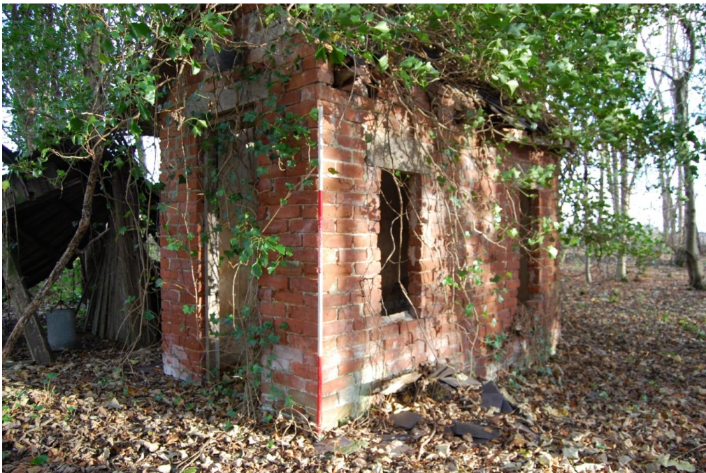
Illus 17 Building 3 facing NE.
