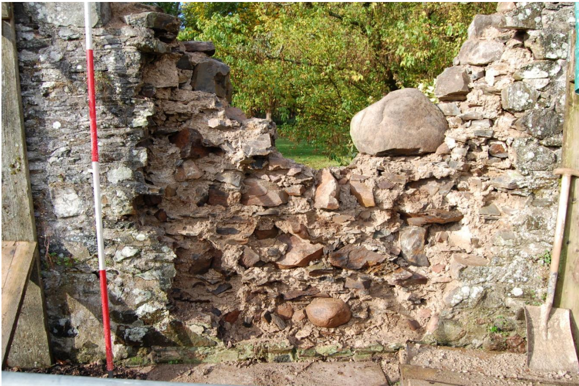
Illus 4 The wall showing laminated slaty stone and large and medium granite fieldstone construction; facing west
