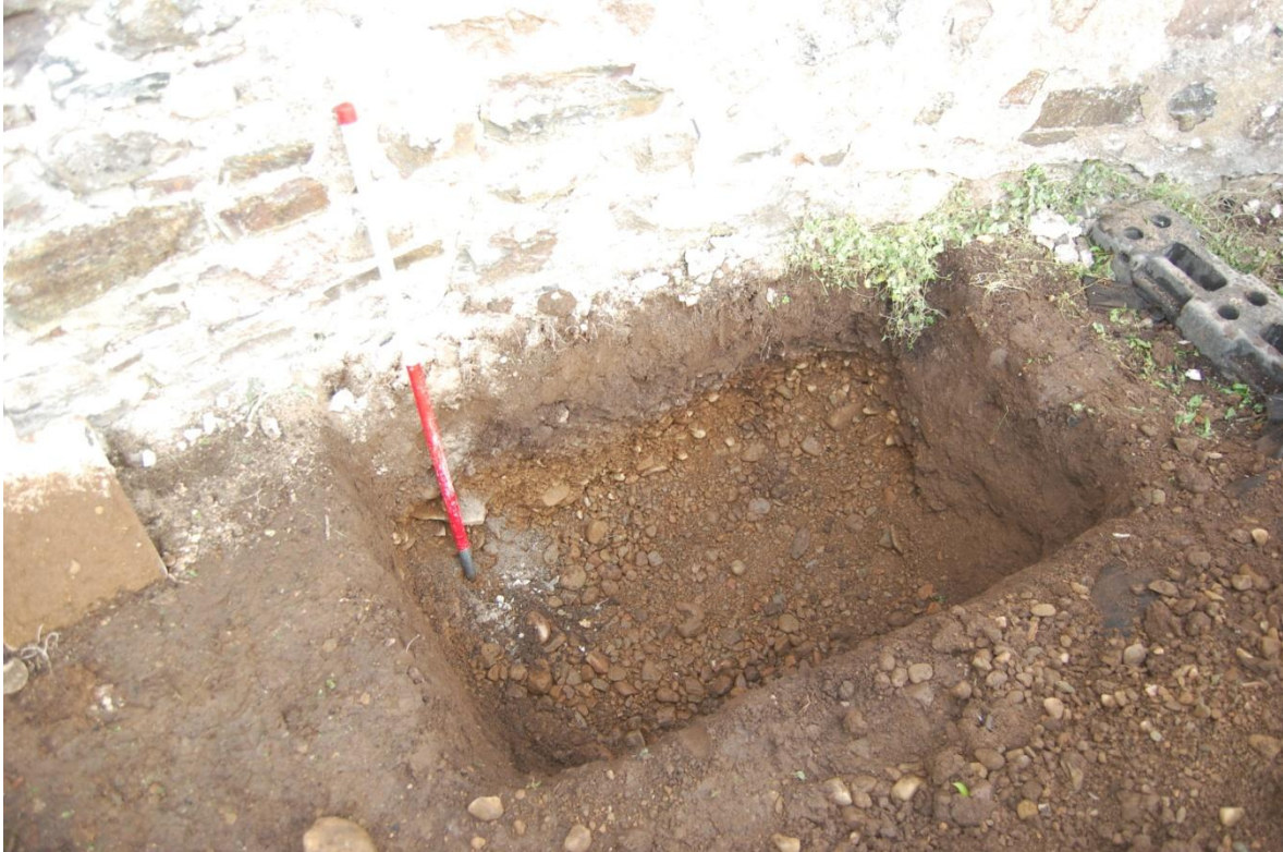
Illus 5 Trench for wall support, facing NW
