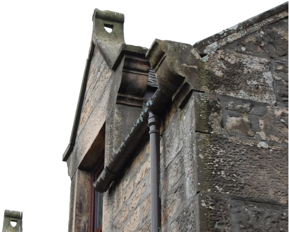
Illus 12 South facade Hattonhill House showing finials and roof detail
