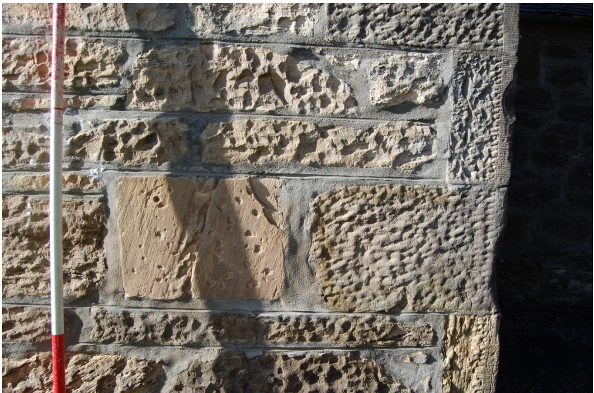
Illus 13 East gable showing tooling marks
