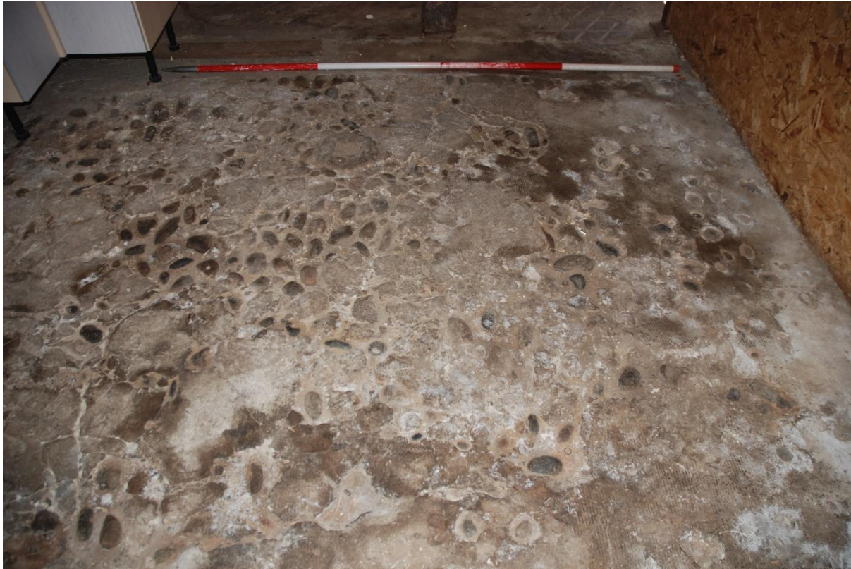
Illus 10 Floor of north room showing waterwashed pebble floor (grepe)
