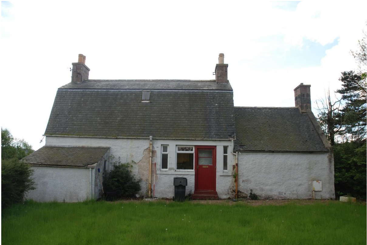
Illus 5 Building 1 the farmhouse; facing south
