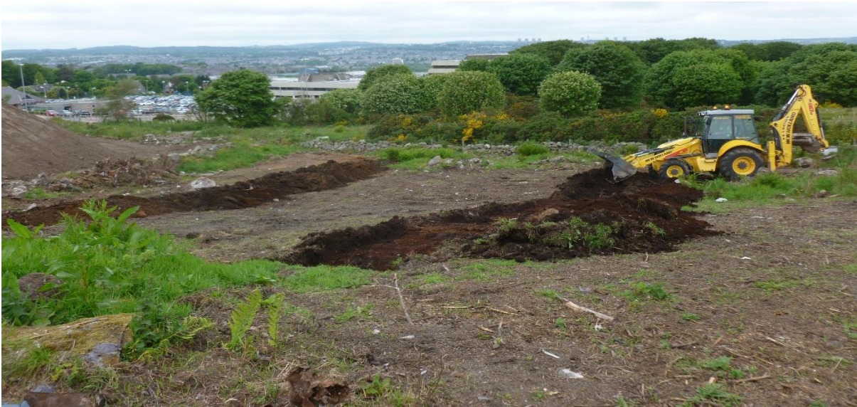
Illus 8 Trenches 8 (left) and 9 (right); facing WNW
