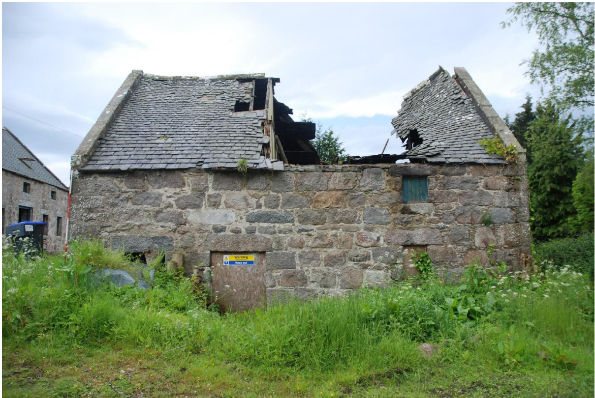
Illus 9 NE façade of mill Building 3; facing SW
