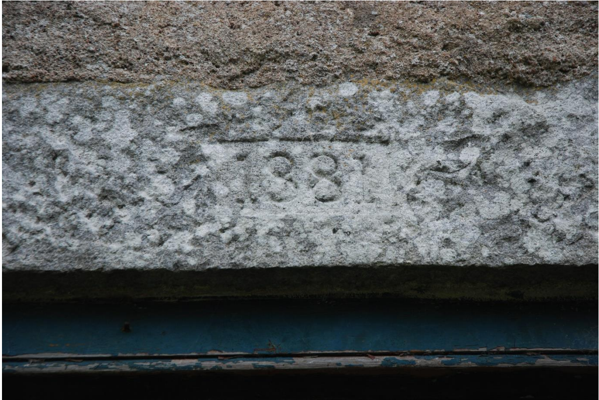
Illus 6 Building 2 lintel above door with '1881' incised
