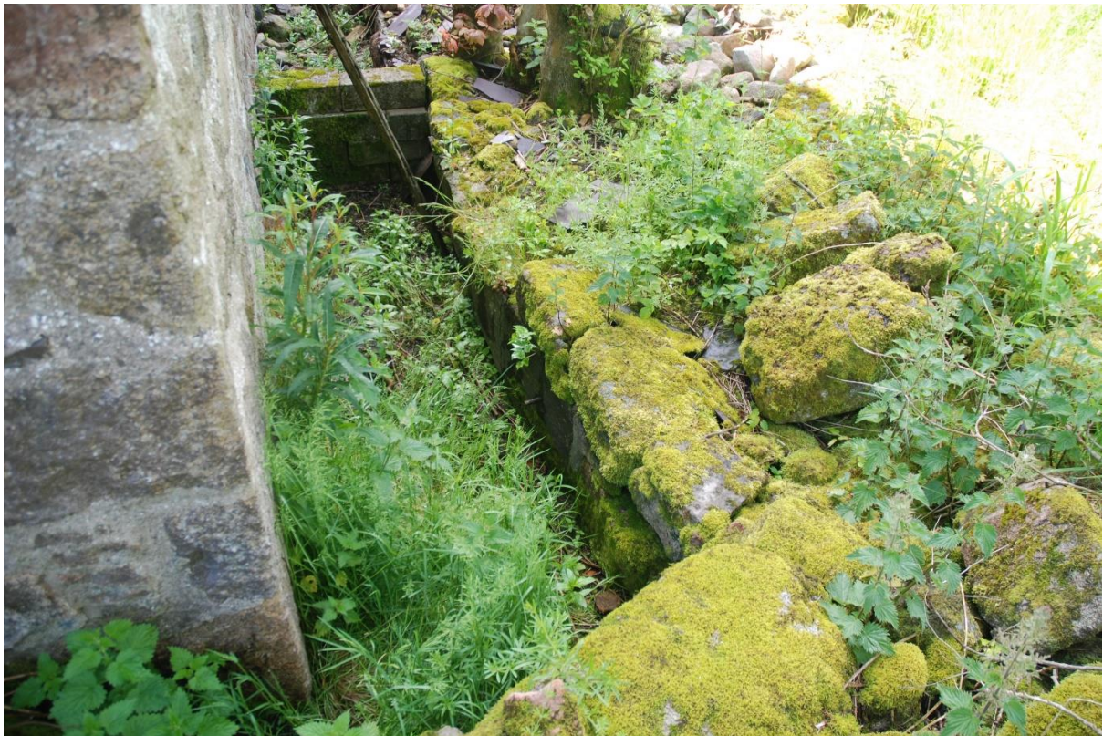
Illus 24 Partially re-excavated mill race on north end of west wall; facing S
