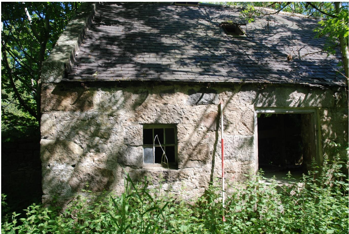
Illus 27 Building 7 south façade; facing N
