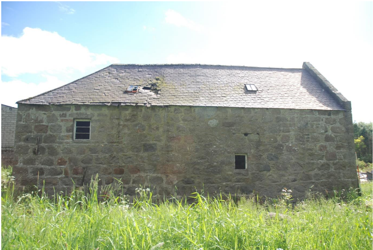
Illus 23 Exterior of west wall showing former location of millwheel (centre); facing E
