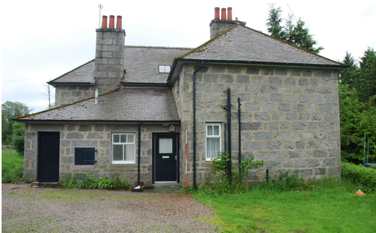
Illus 2 The mill house; facing SSW
