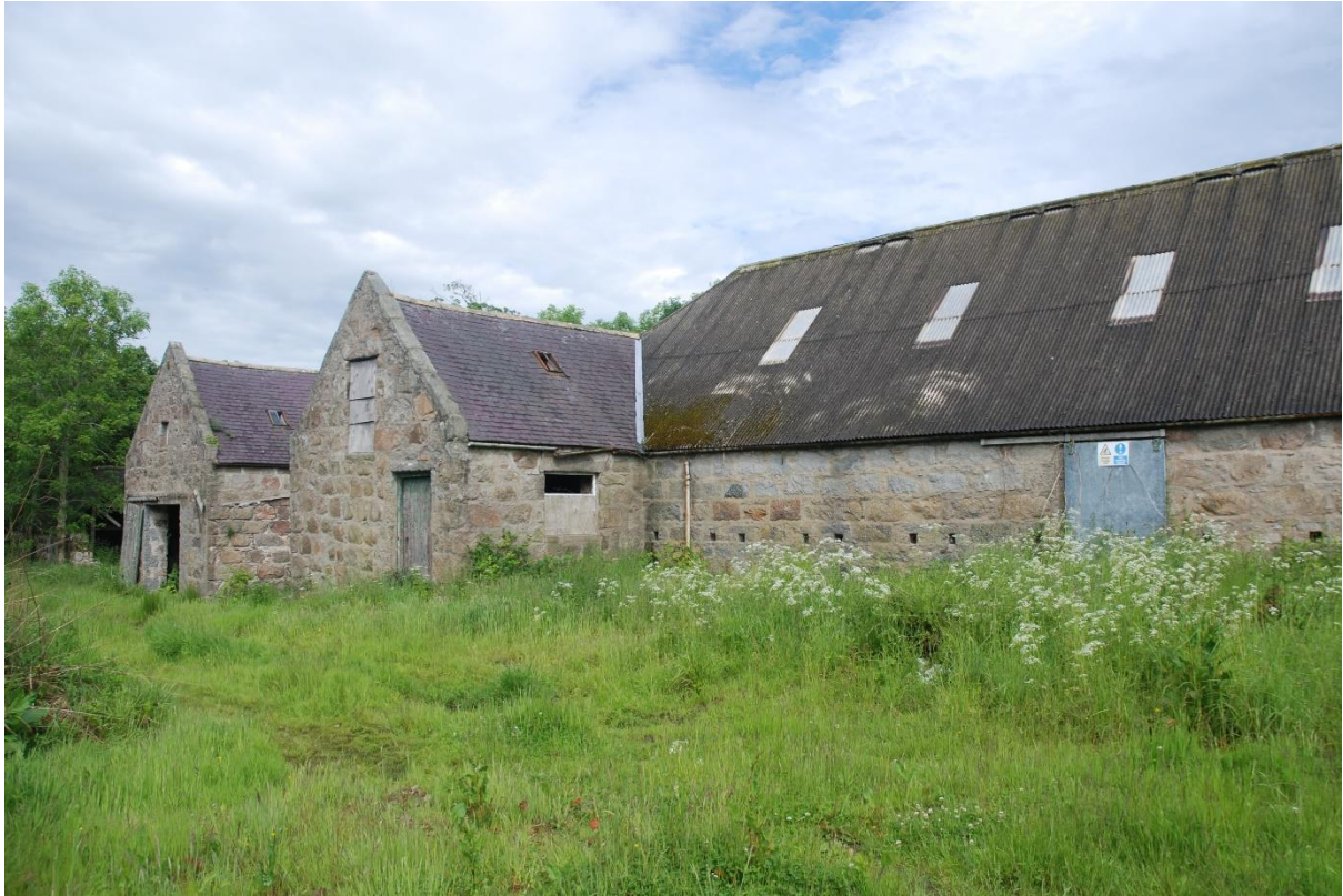
Illus 19 Building 6 from SE showing conversion to steadings; facing NW
