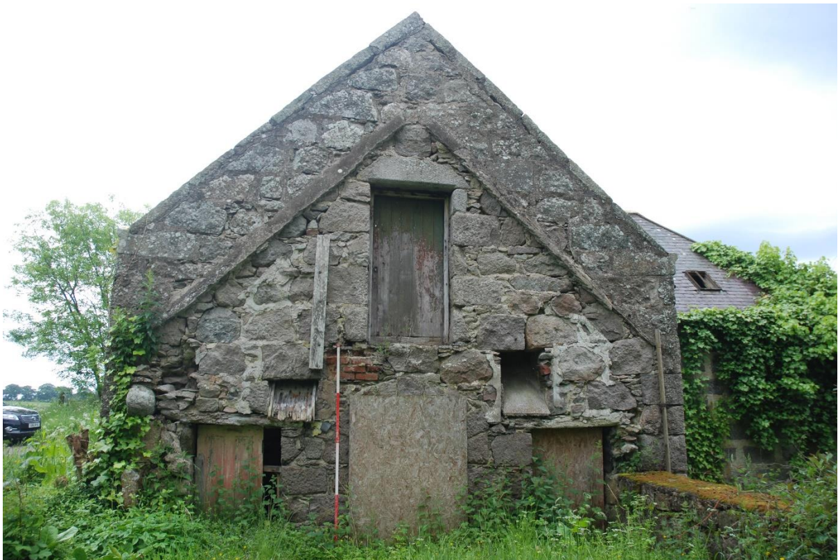
Illus 10 NW end of Building 3 showing central arched door, grain chutes, upper door and roof scar from extension now demolished; facing SE
