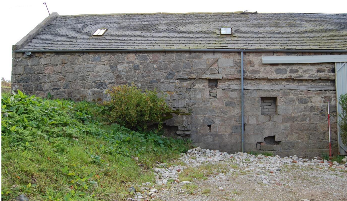
Illus 5 Exterior wall of the NW range, north end showing north extension of the building in Phase 2 (left of centre) and the apertures for the Phase 1 horse mill and Phase 2 water mill. The rubble from the recently demolished grain store can be seen bottom right; facing SE
