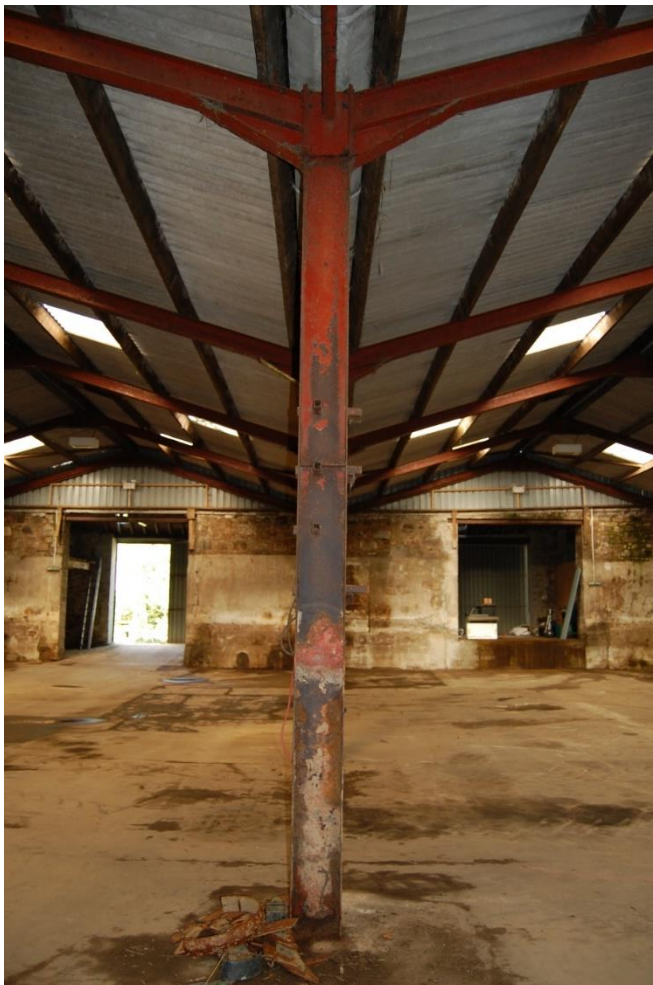
Illus 15 SE internal wall of courtyard showing cast iron beams supporting roof
