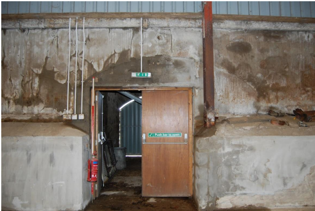
Illus 14 NE internal face Door D6 showing as a scar in the concrete infill created when the sheds were converted for cattle in the 1960s; the modern door (D7) dates to this phase
