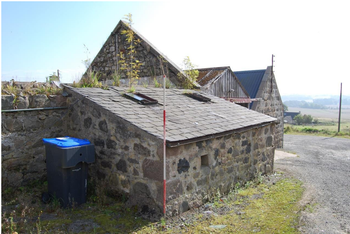
Illus 7 Lean-to shed Room 6; facing SE
