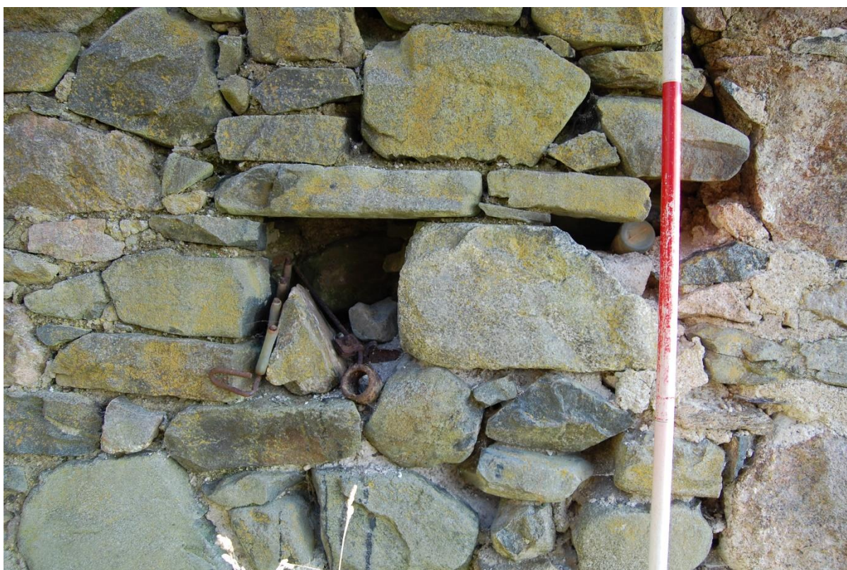
Illus 5 Stone alcove in NE wall Room 2
