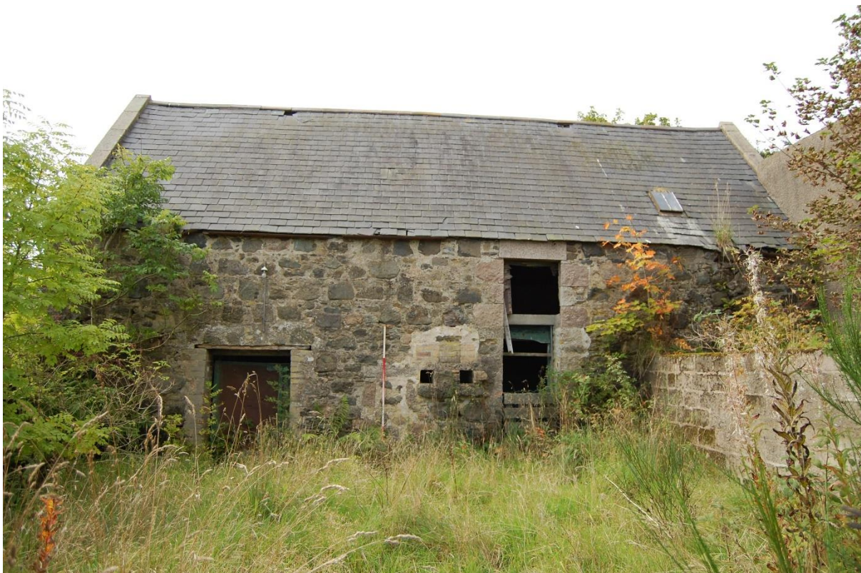
Illus 8 Mill building rooms 9 and 10; NE wall facing SW
