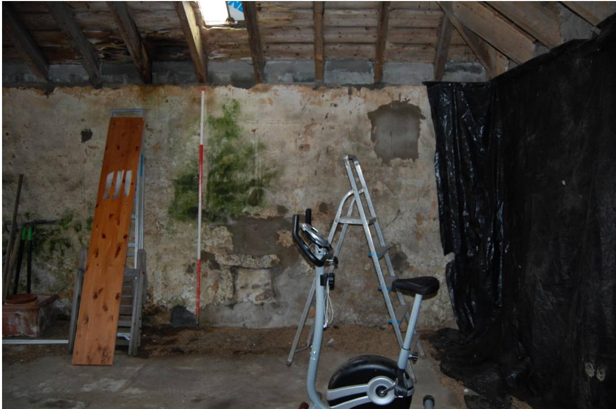
Illus 5 East end of north wall of steading showing Window W2 (top right blocked) and F4 and F5 (centre) the apertures for the horse mill driveshaft.
