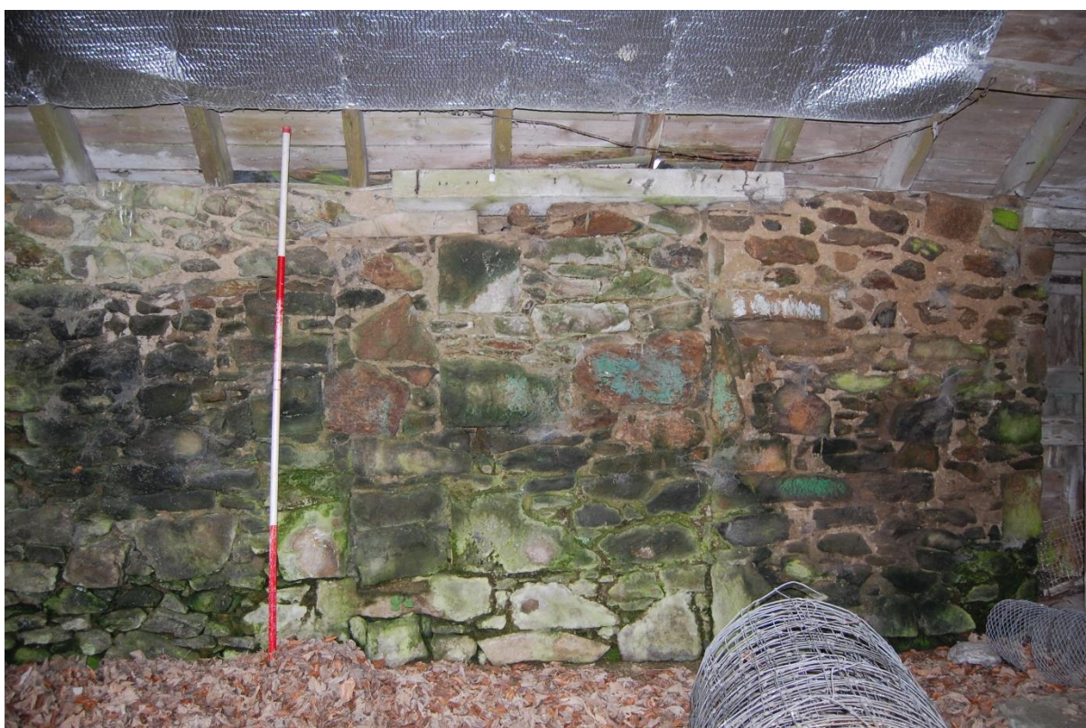
Illus 6 Building 1 interior west wall showing blocked door D4 (centre) and F1 (left) and F2 (right) apertures for driveshaft of horse mill
