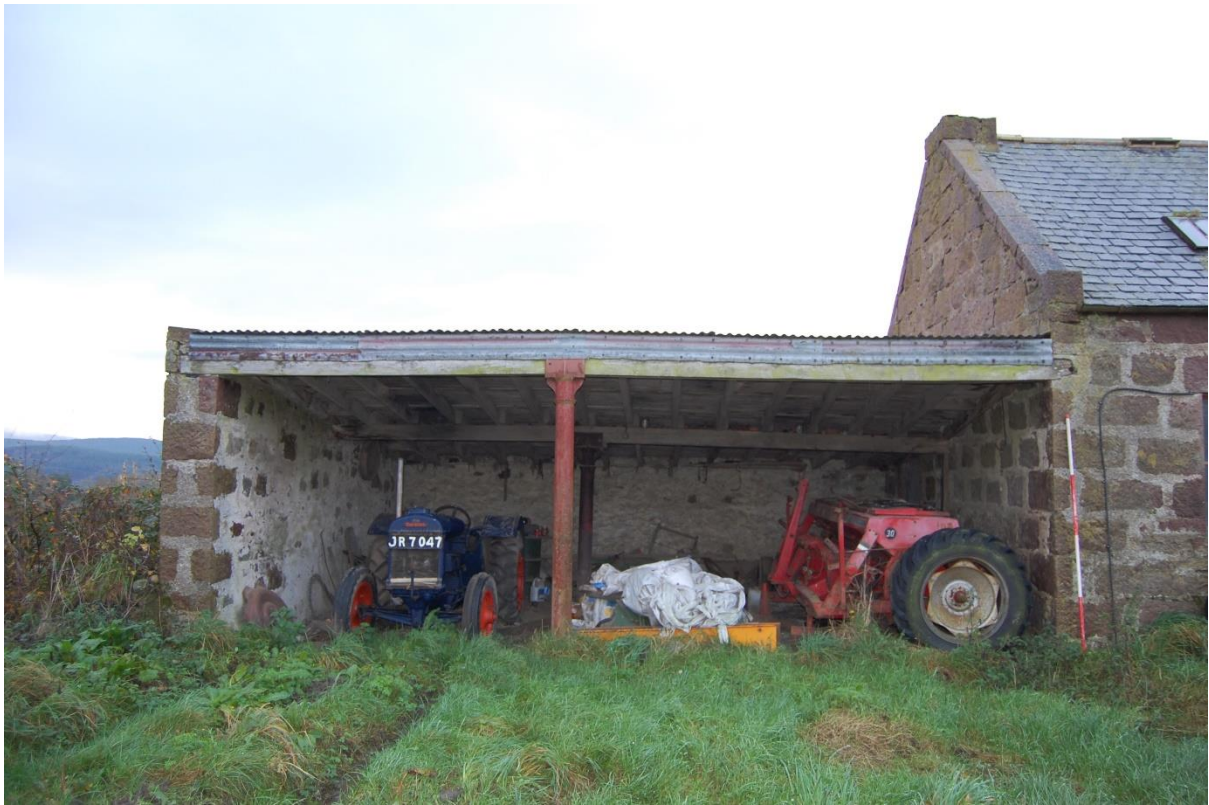
Illus 10 Building 1A with cast iron pillars; facing SW
