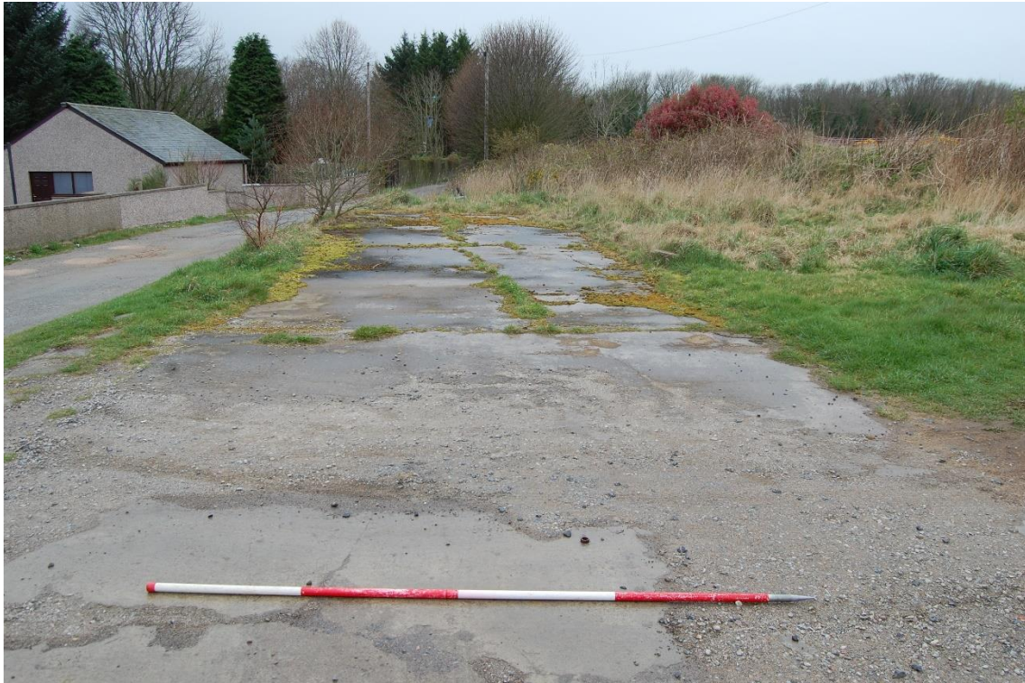
Illus 36 concrete base F10; facing SW
