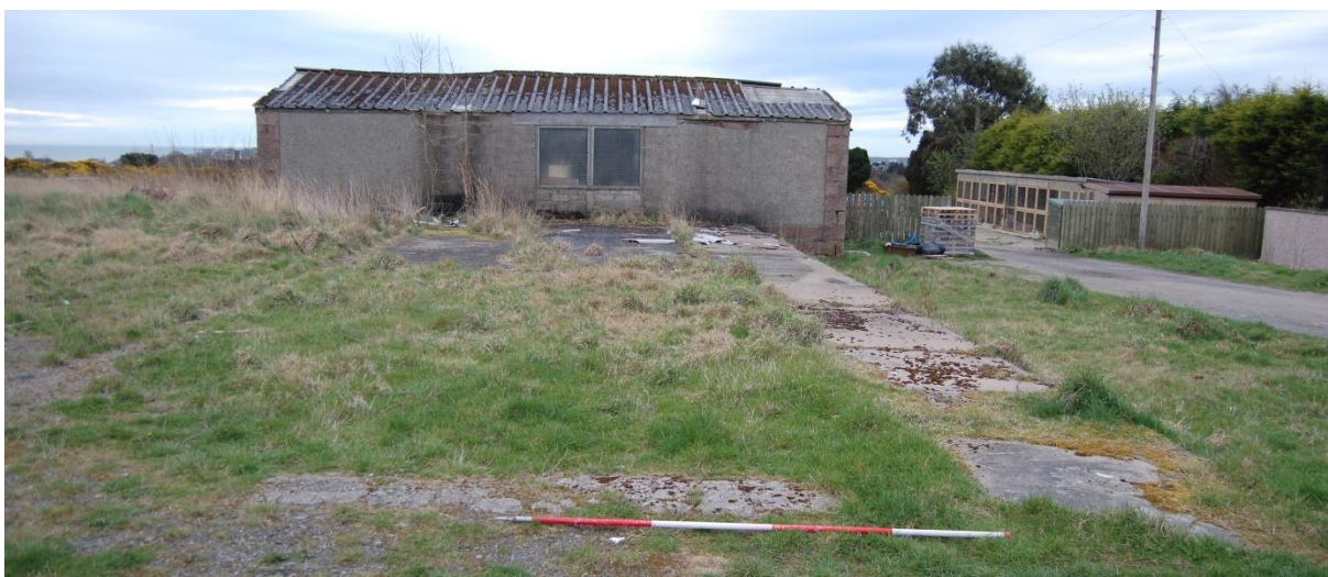
Illus 39 concrete base F13 with F14 (background); facing SE
