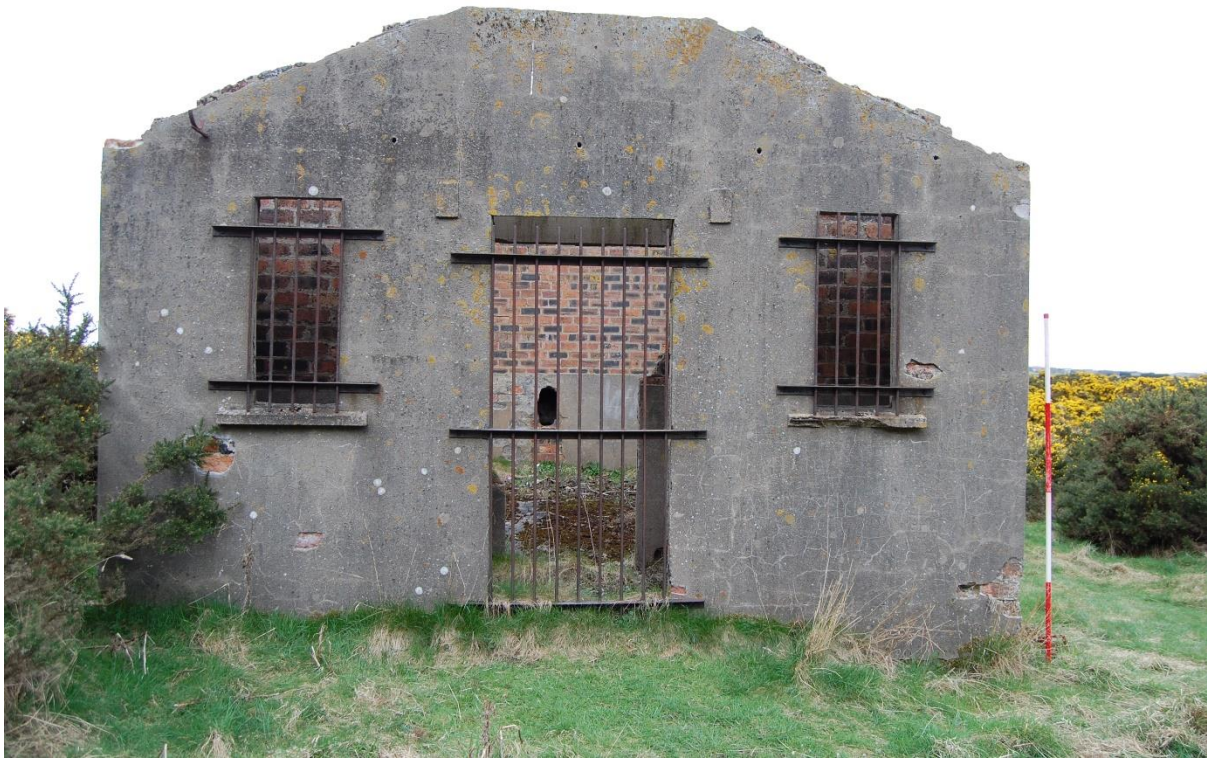
Illus 14 F7 south frontage; facing N
