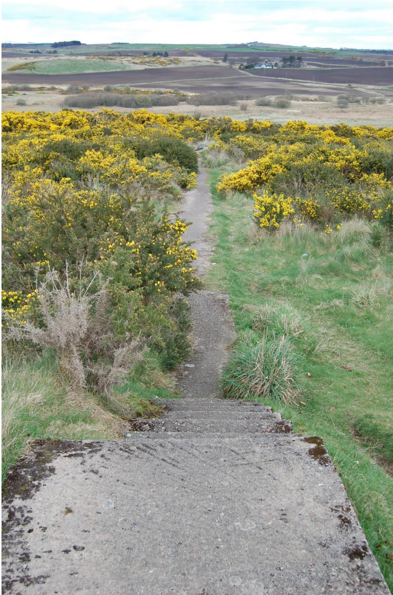
Illus 8 Path F4 with steps F22 (foreground); facing north
