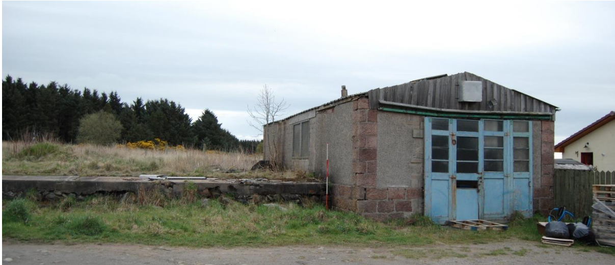
Illus 40 concrete base F13 (left) with F14 (right); facing ENE
