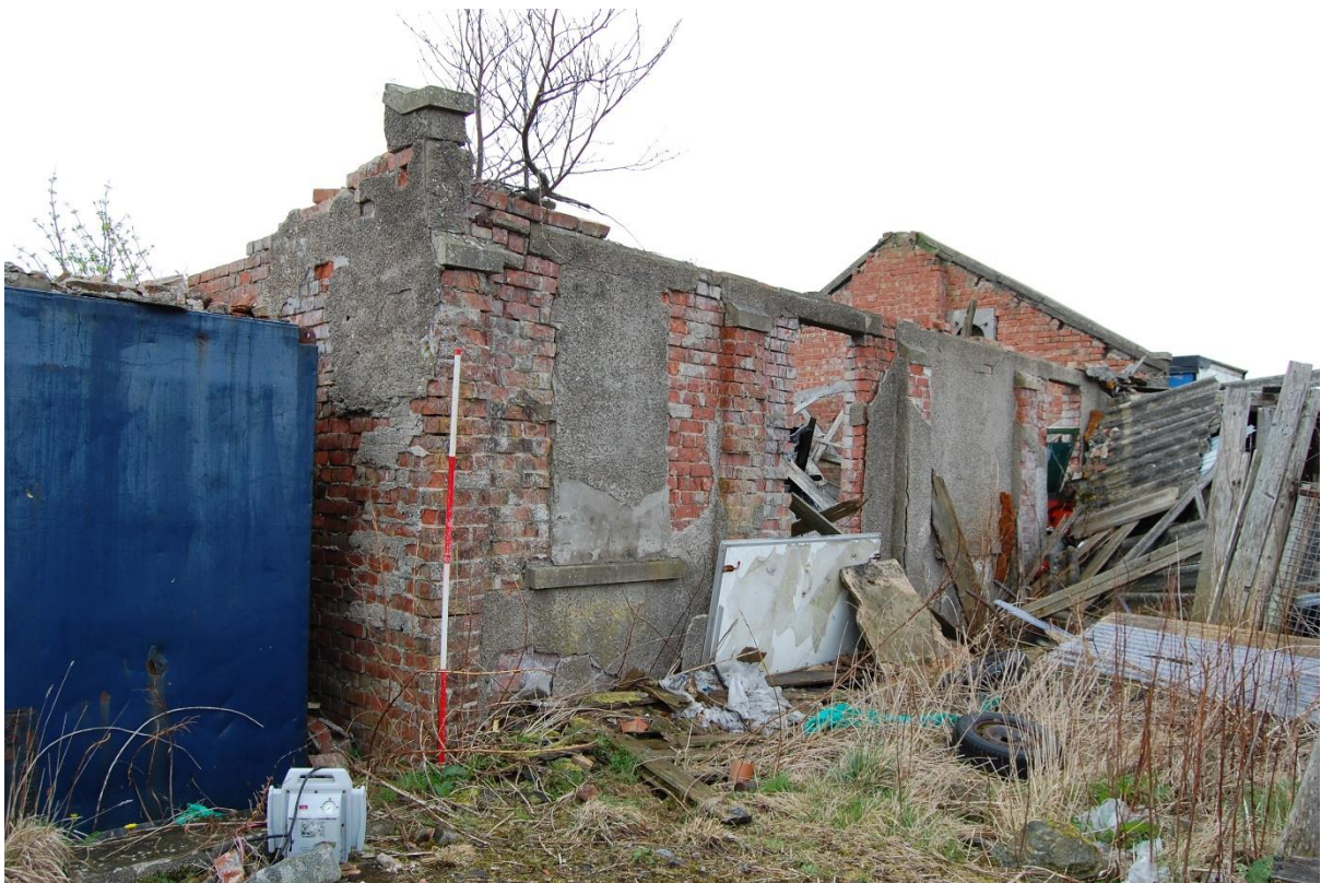
Illus 35 F9 NE wall; facing W
