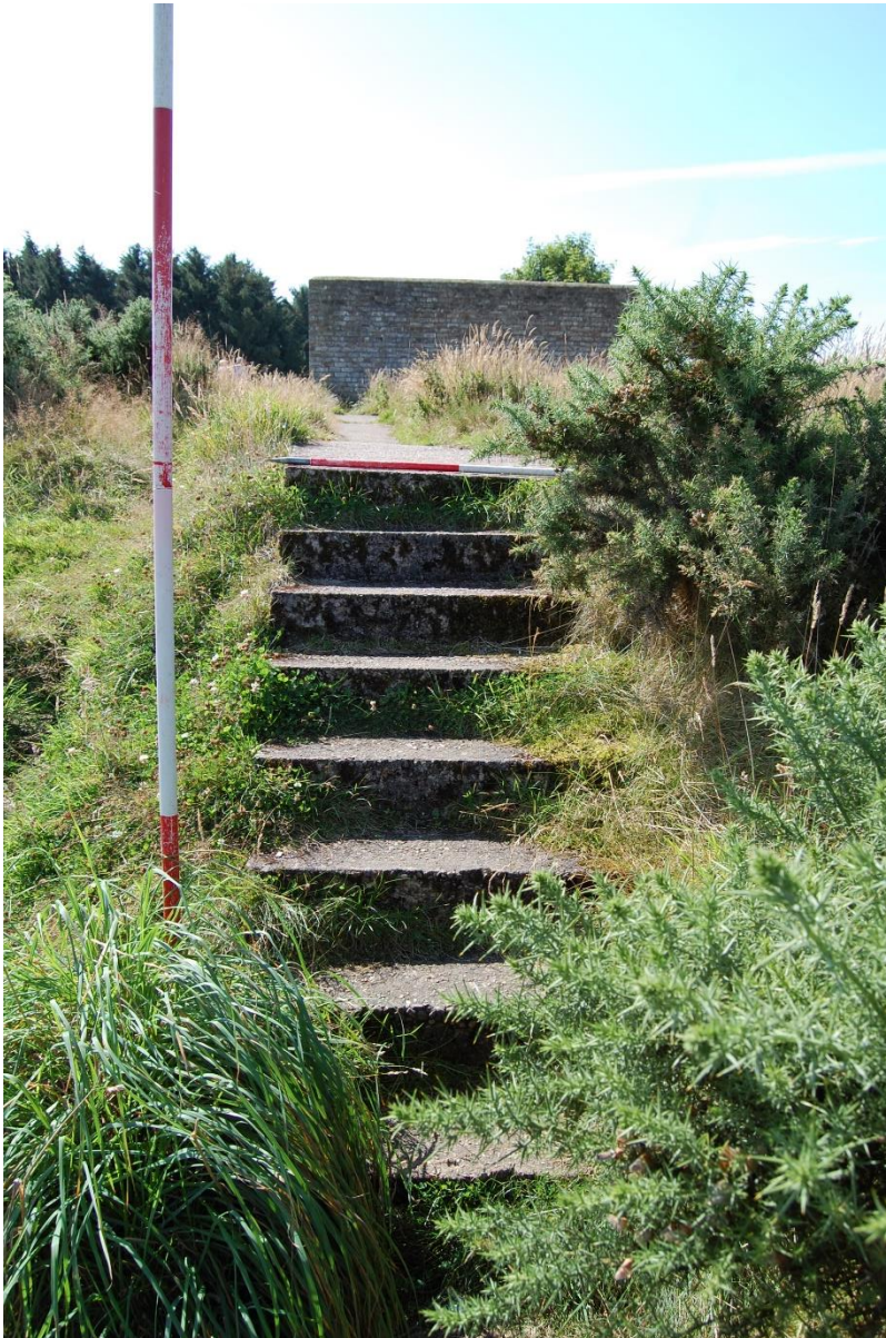
Illus 25 Concrete steps F22 with building F6 (top); facing S
