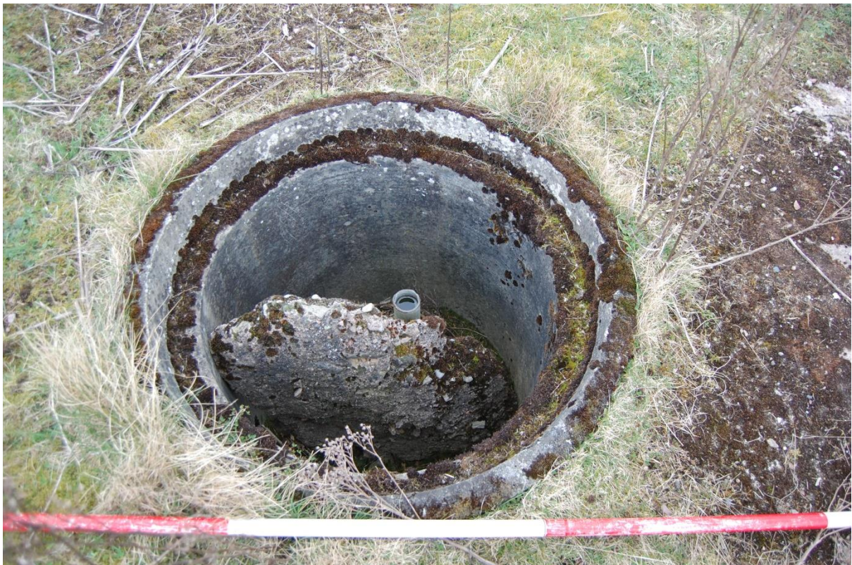
Illus 18 F7 central concrete pipe showing central cable fitting; facing E
