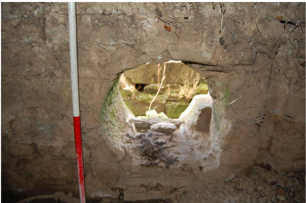
Illus 10 Detail of F1, mill wheel drive shaft aperture SW gable
