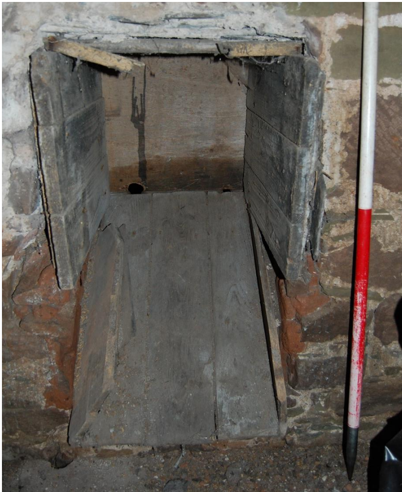
Illus 25 Wood-lined grain chute, F15 in first floor Room 2 NE gable; this chute would have carried grain from the upper Room 1 to the grinding floor; facing NE
