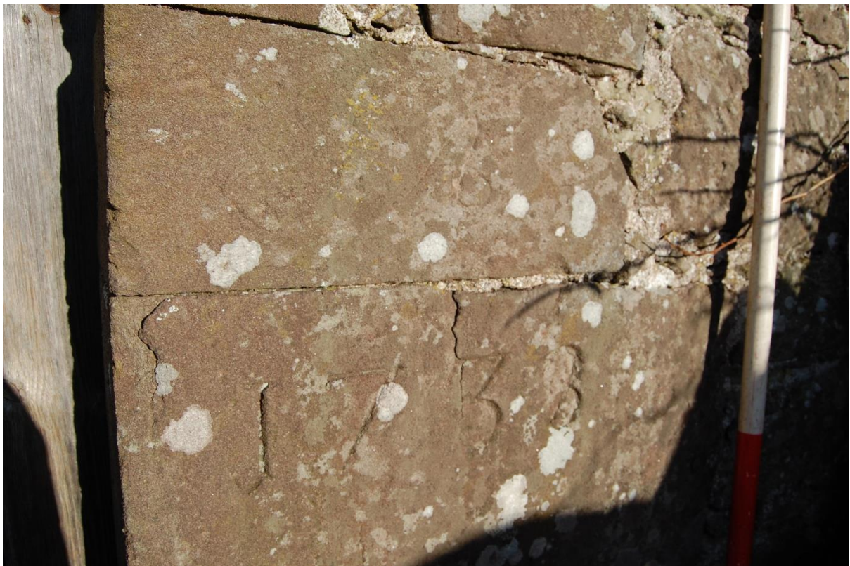
Illus 6 Door D17 date stone detail; facing NNW
