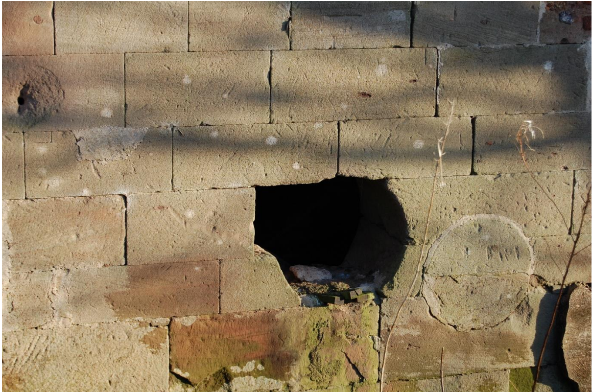
Illus 9 Wheel driveshaft F1 in Phase 1 room 2 SW gable; facing NE
