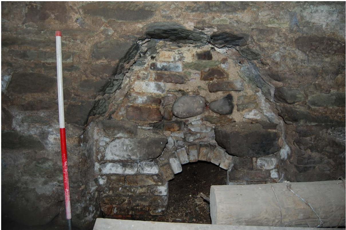
Illus 22 Brick flue F3 inserted into the stone NE gable Room 2
