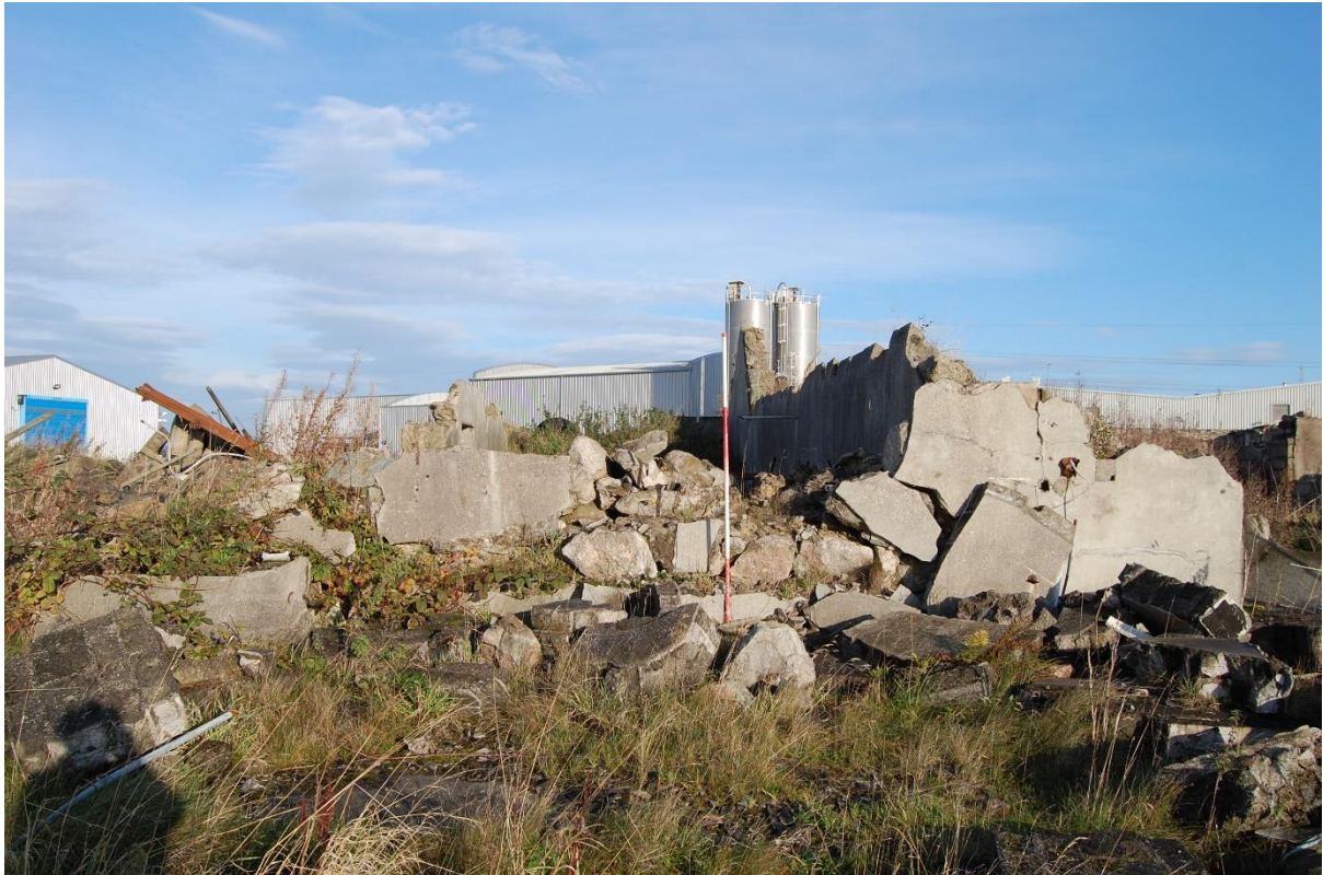
Illus 4 South wall Room 1 showing ruinous nature of buildings and concrete in exterior and interior; facing NW
