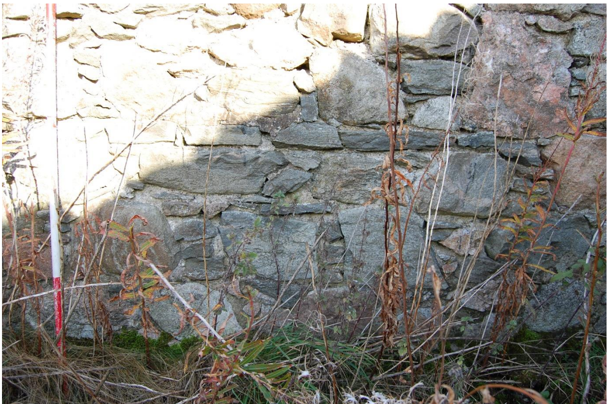
Illus 5 Blocked aperture F1 in north wall Room 4; facing NW
