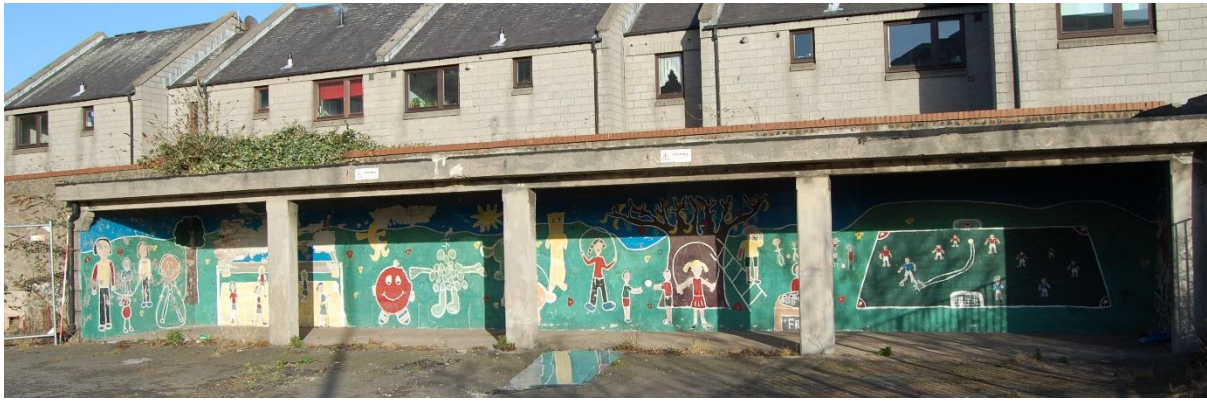
Illus 13 Building 5 open-sided shelter; facing NE
