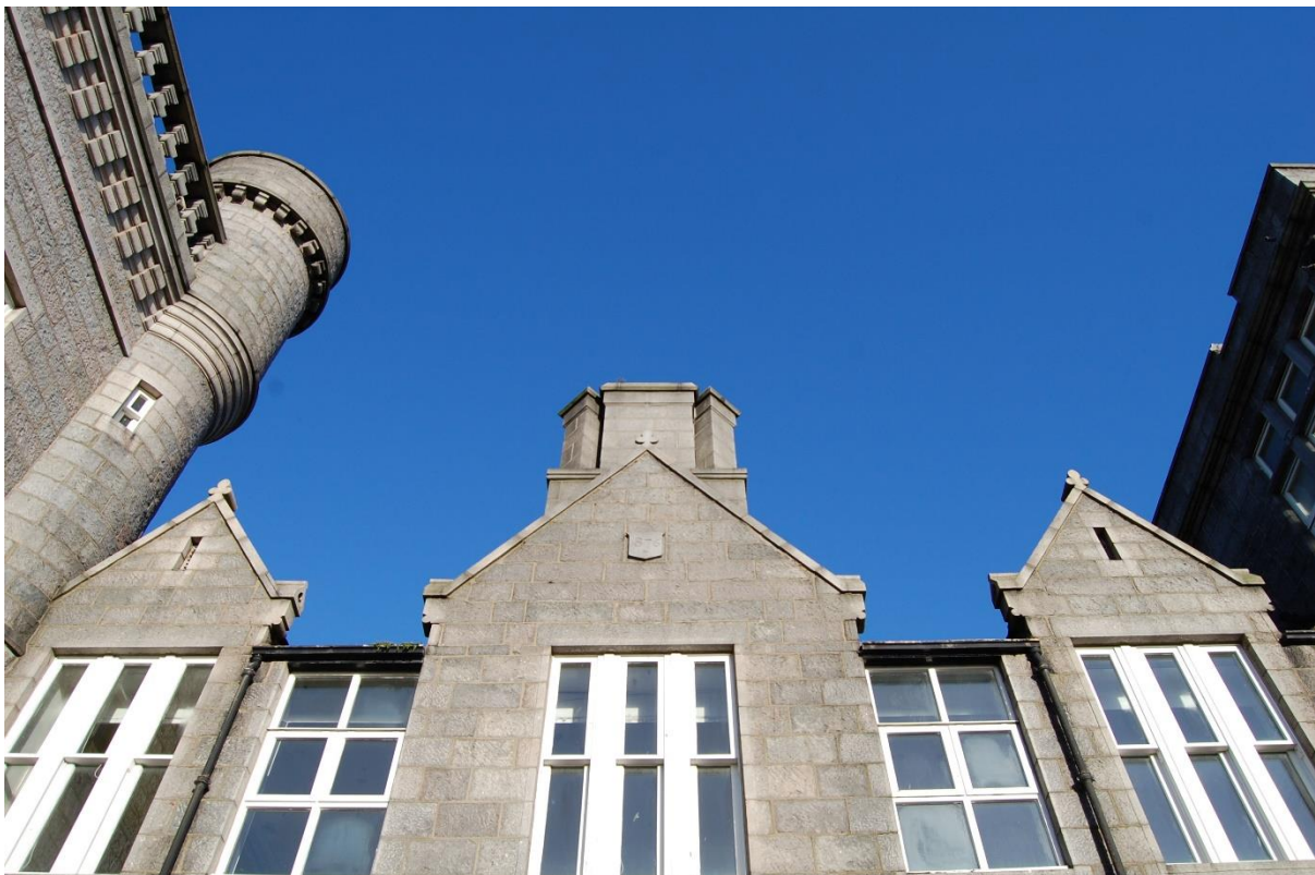
Illus 14 Building 6 SW façade with 1876 date plaque (centre); facing NE
