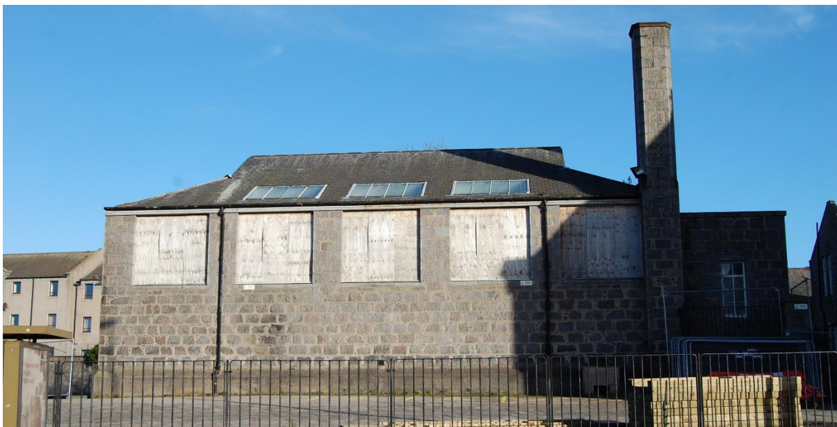
Illus 4 Building 2 the gym, SW façade; facing NE
