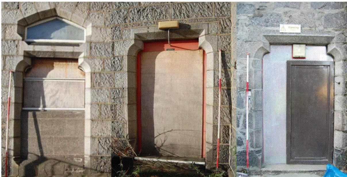
Illus 10 Building 6 Doors D2 (left) D3 (middle) and Building 4 D10 (right)
