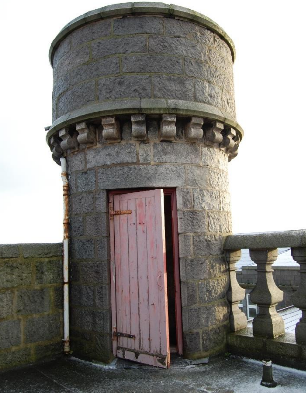
Illus 18 Stair turret F3 granite top; facing E
