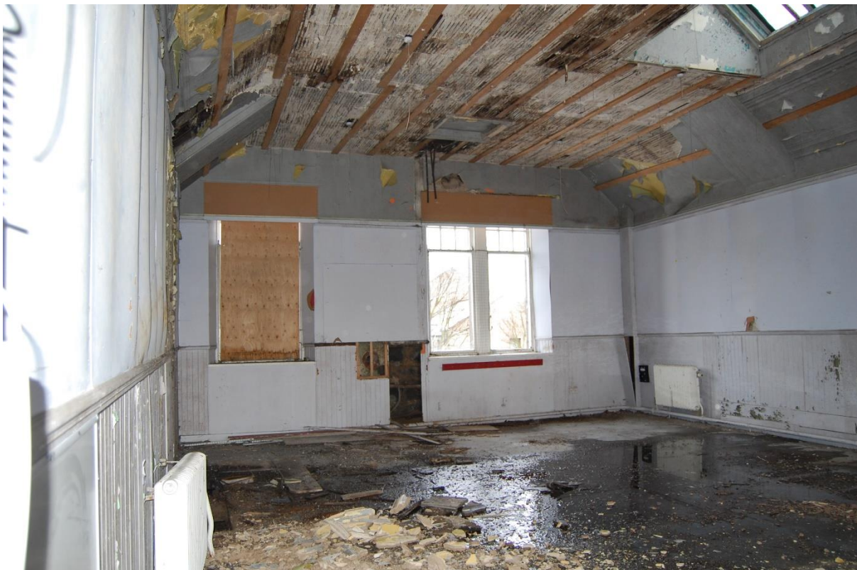
Illus 12 Building 4 the nursery first floor classroom; facing NNW
