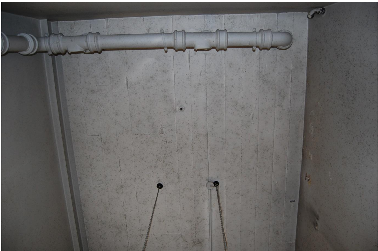
Illus 21 Building 6 tower ground floor room poured concrete ceiling; facing NW
