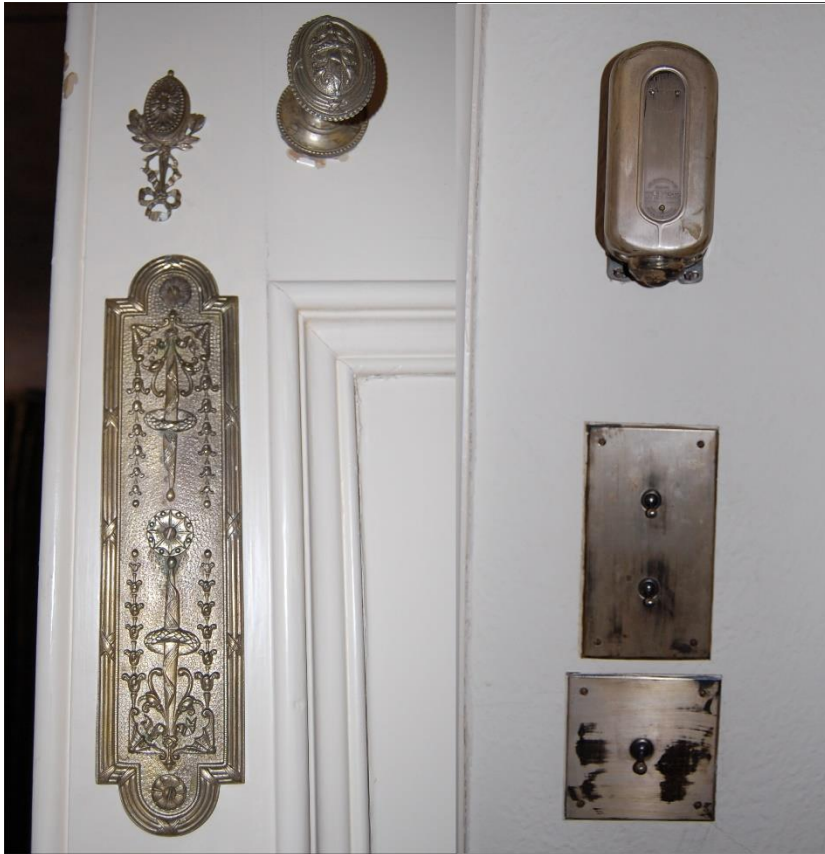
Illus 13 Room 2 door fittings (left) and light switches (bottom right) and Satchwell thermostat, The Rheostatic Co Ltd, Slough Type N No 10812 Automatic control for electric heaters, Patent 1948 in UK (top right); facing ENE.
