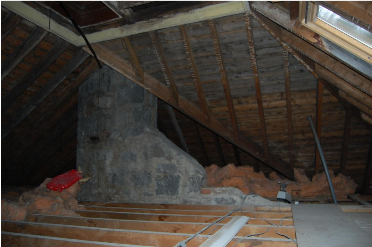
Illus 17 Gable chimney stack on NW end of Phase 4 (above fireplace F5) visible in attic; facing NW
