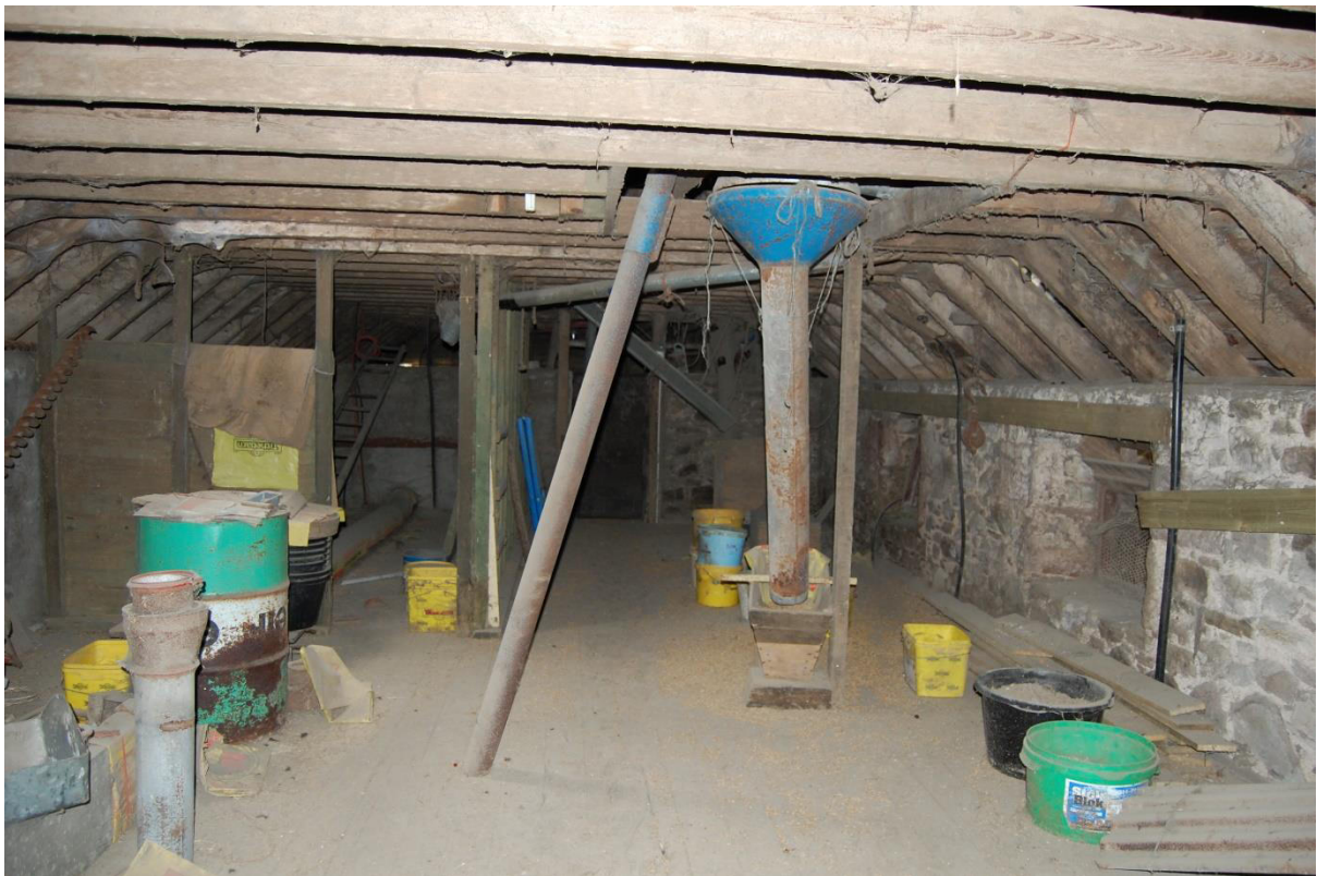
Illus 9 Phase 1 Room 13 (first floor above Room 10); facing SE
