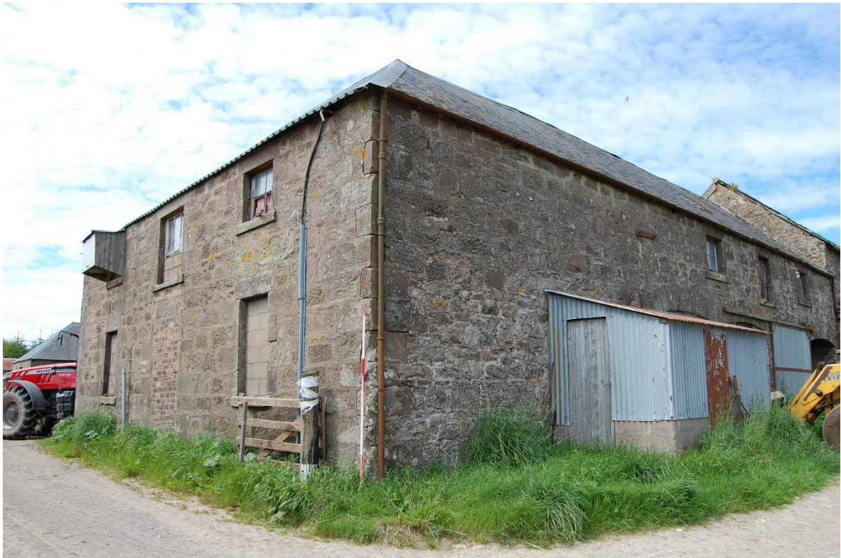
Illus 10 Phase 1 farmhouse Room 11 with blocked windows now used as a grain store; facing W
