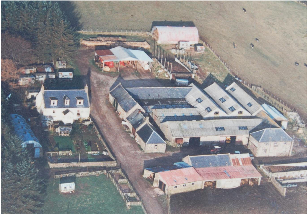
Illus 3 Copy of photograph of farm in 1980 showing buildings prior to collapse of roofs and dereliction of Rooms 4-8; facing N
