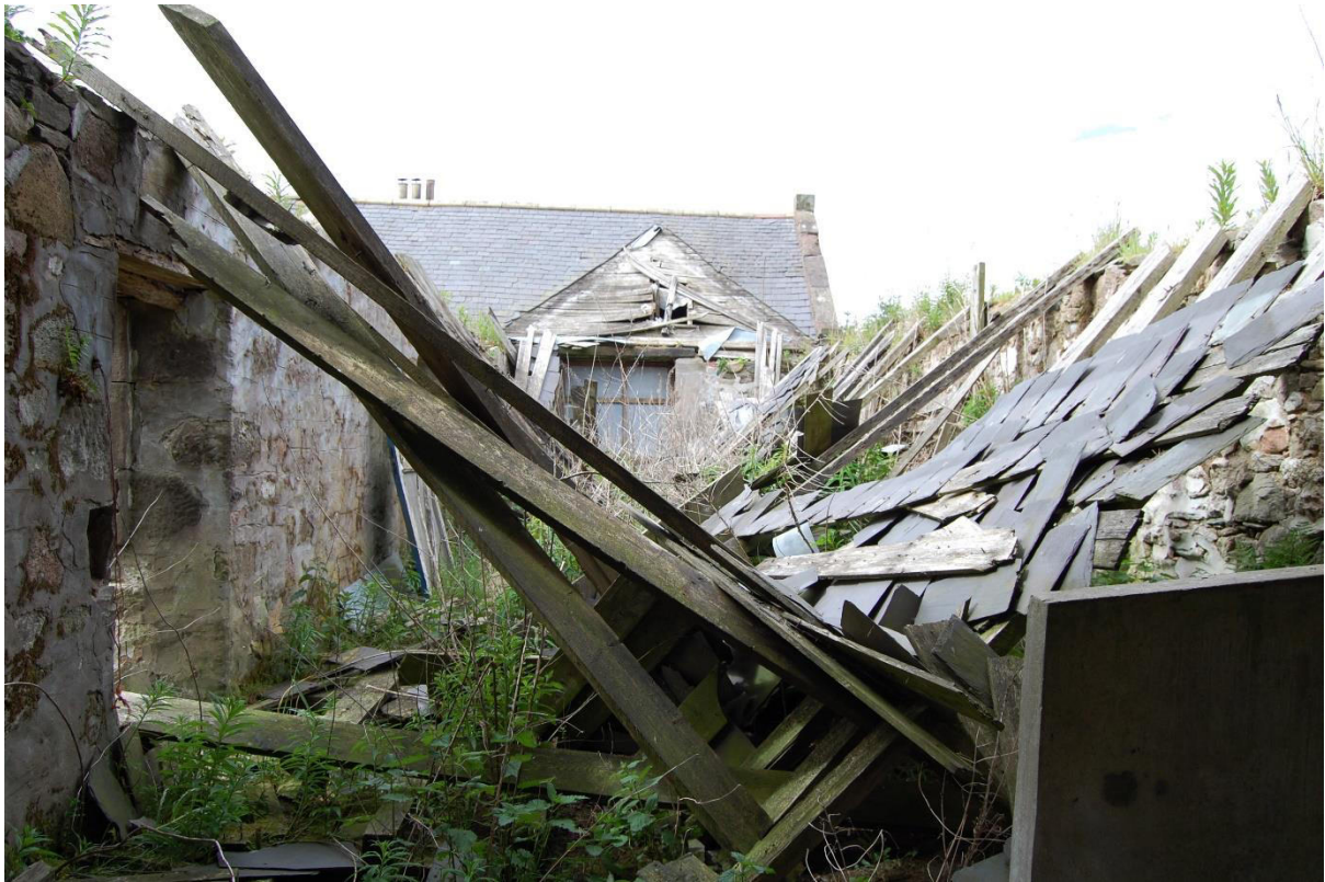
Illus 6 Phase 1 Room 4 SW end showing collapsed roofing and Phase 2 Room 3 (top centre); facing SW
