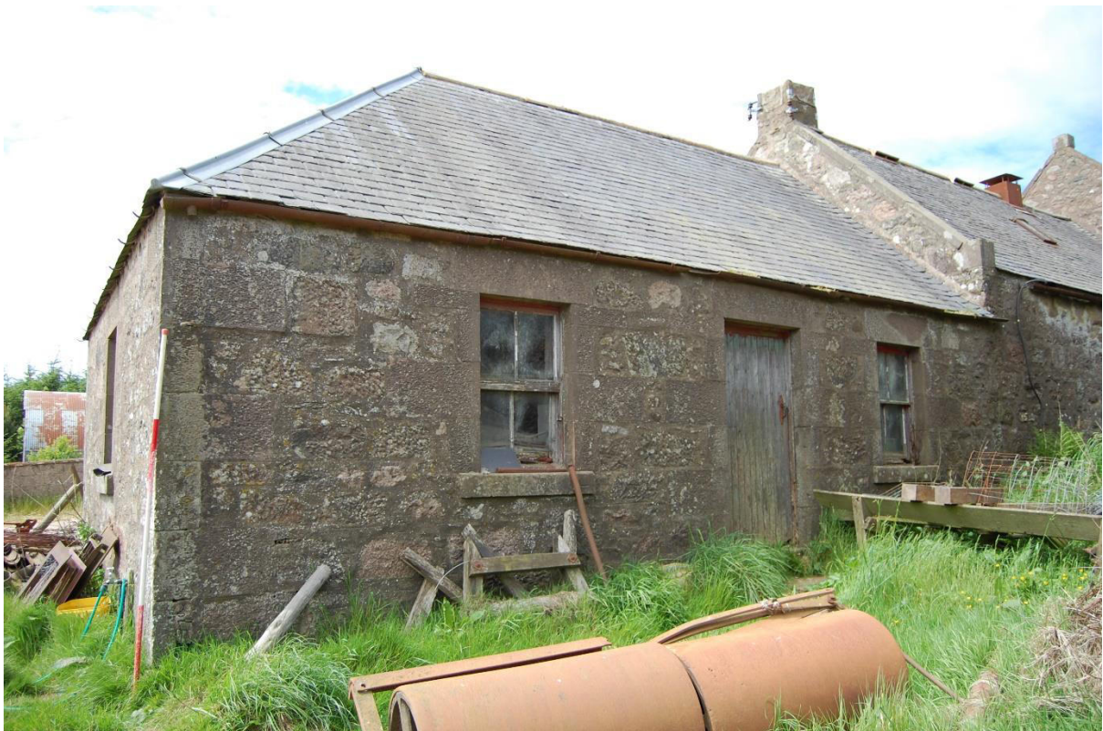
Illus 22 Phase 2 bothy Room 1; facing WSW
