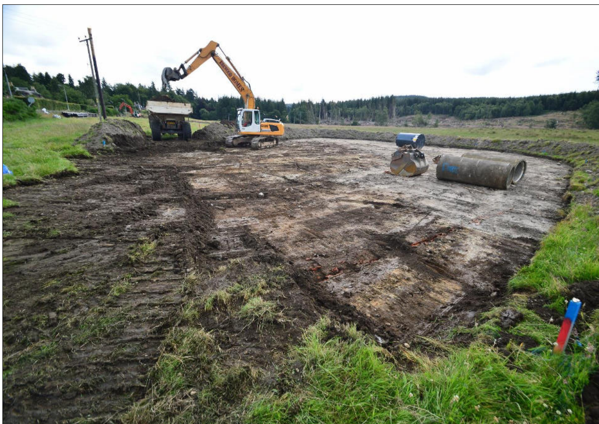
Illustration 3: View of SUDS area looking NE near completion of soil strip on 27 July.
