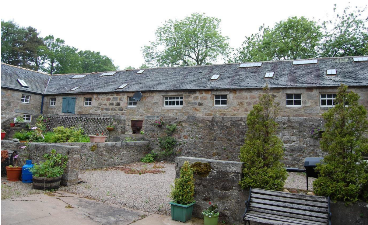
Illus 8 NW range SE wall within courtyard; facing WNW
