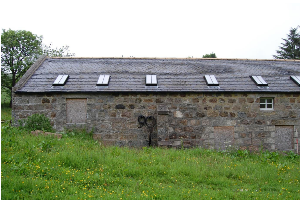
Illus 10 SW elevation with W13, F1, F2, W14, W15; facing NE
