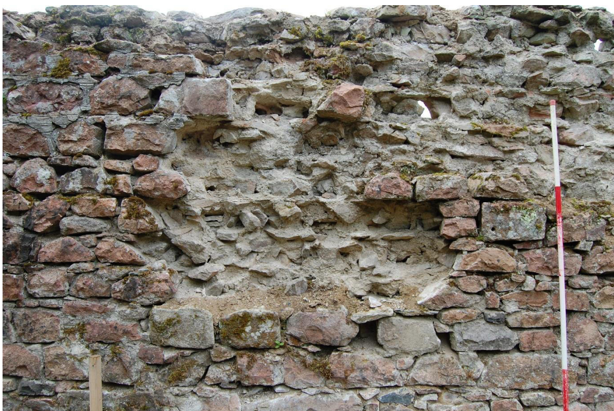
Illus 5 N face of wall F7 showing area of damage (left) and socket stone F5 (right)
