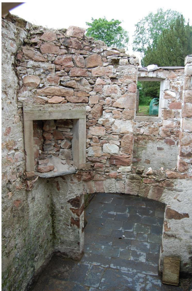
Illus 14 Structure 1 showing Phase 1 inserted wall with corner fireplace F9 showing stone rubble above, door D2 (below) and door D6 (above) with W1 in background; facing WSW
