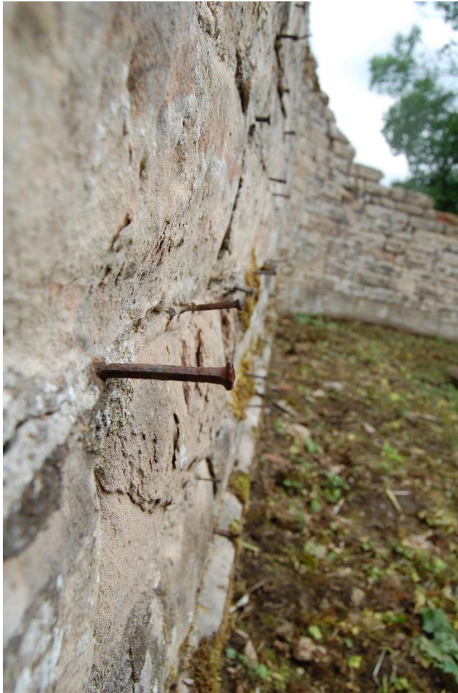
Illus 8 Iron nails concentrated on the S facing inner face of the wall for espalier; many overgrown fruit trees were cleared from this area by the present owners; facing ENE
