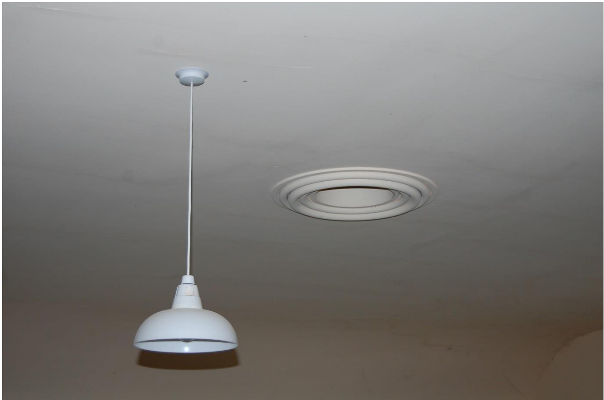
Illus 15 Detail of older light fittings (?gas; right) and modern light fittings
