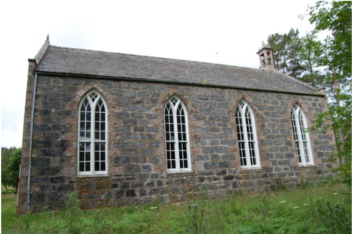
Illus 9 ENE wall with windows W4 (right), W5, W6 and W7
