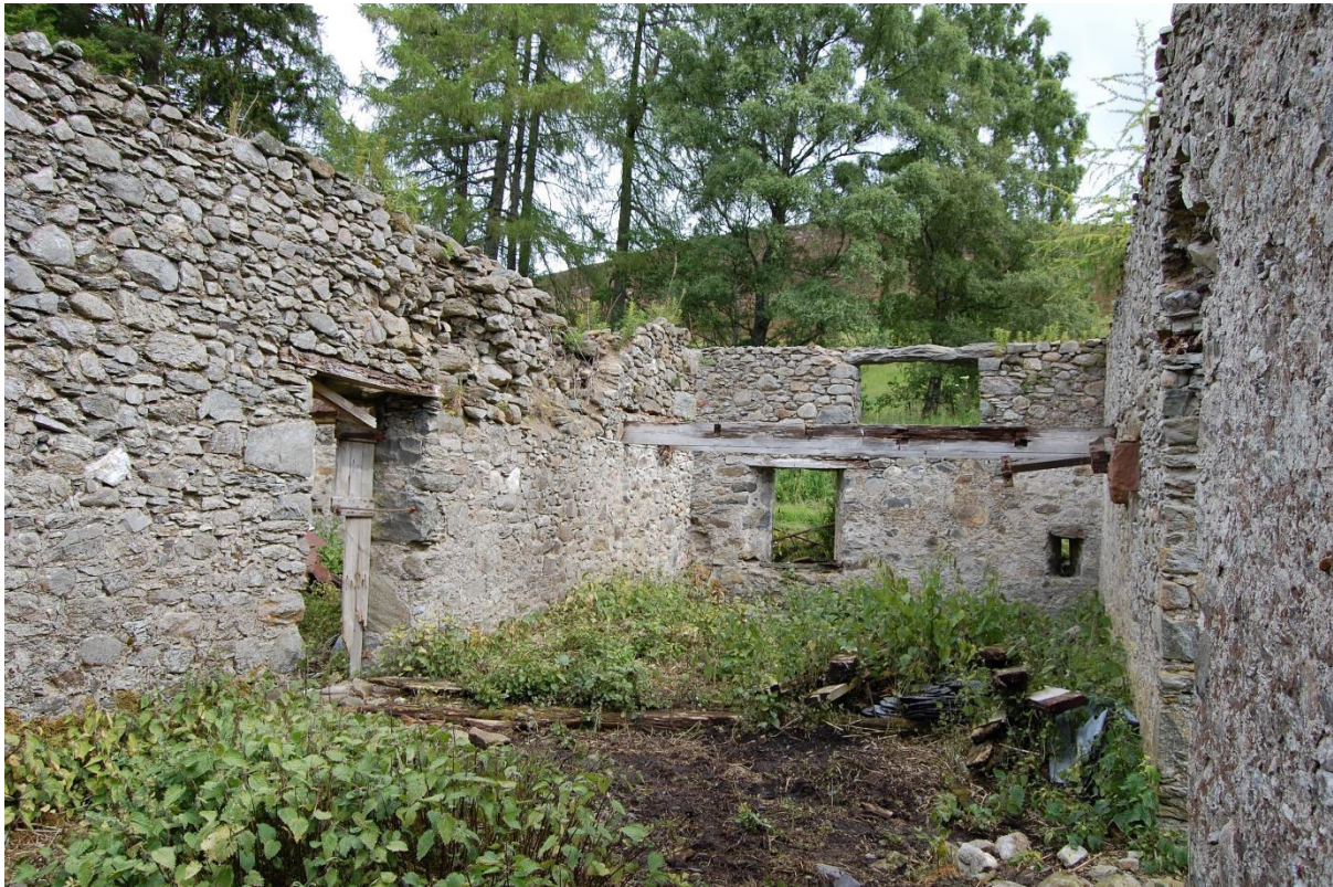
Illus 8 Interior Room 2; facing NE
