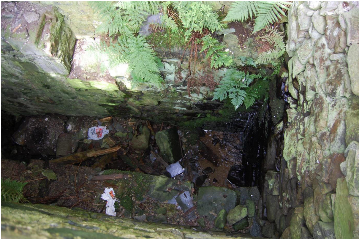
Illus 6 Wheel pit F1 (not accessible) photographed through roof of Room 3; facing NW
