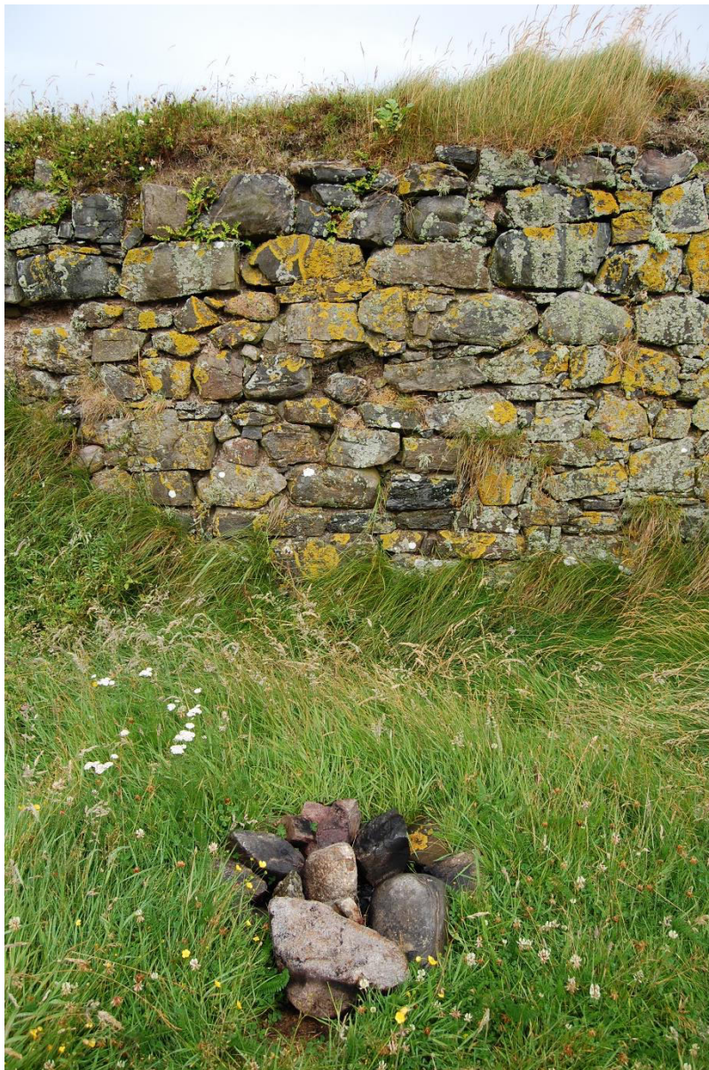
Illus 4 Interior W elevation showing stones missing and recent fire setting (foreground)
