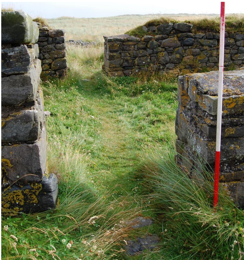
Illus 8 S door (foreground) and N door showing little repair needed, mortar along jambs and well-used access route
