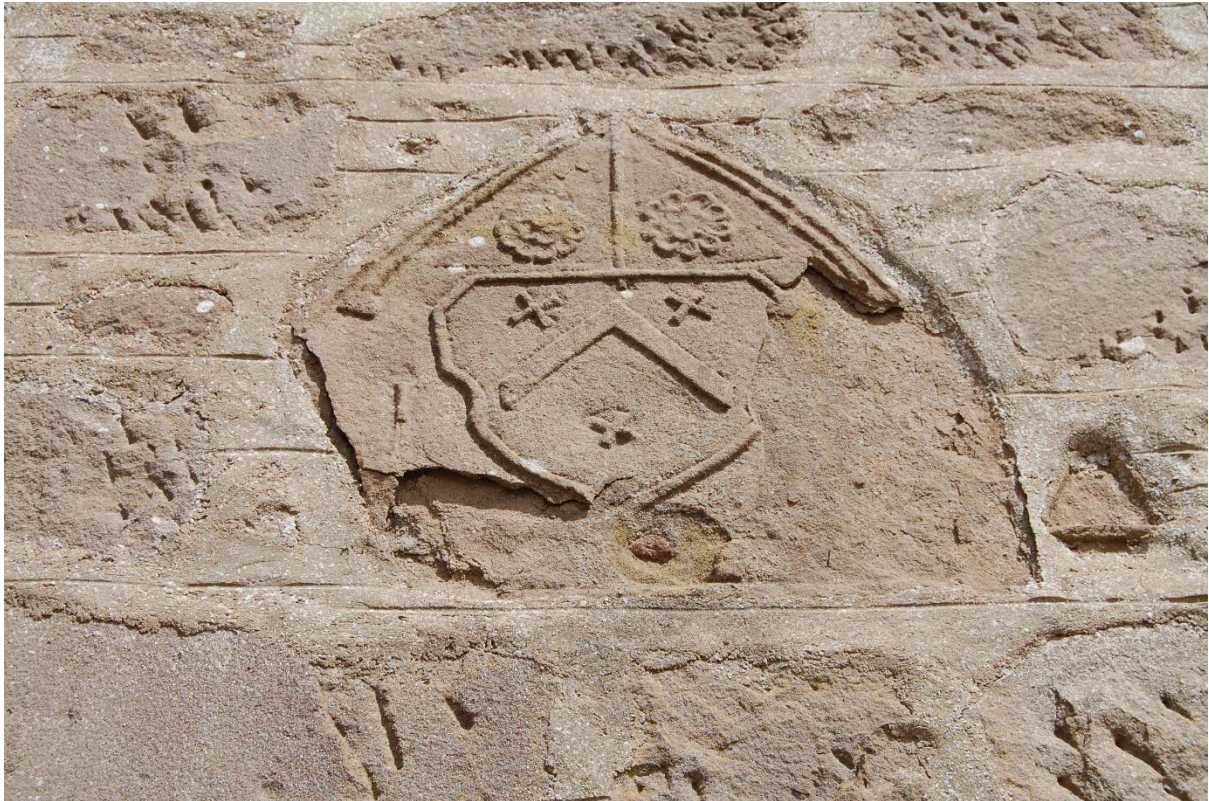
Illus 13 Armorial panel F7 the Barclay arms; the initial I (part of IB which together with the figures '7 1' at bottom right and a '1 6' at the bottom left, have been lost due to delamination of the stone); facing NE
