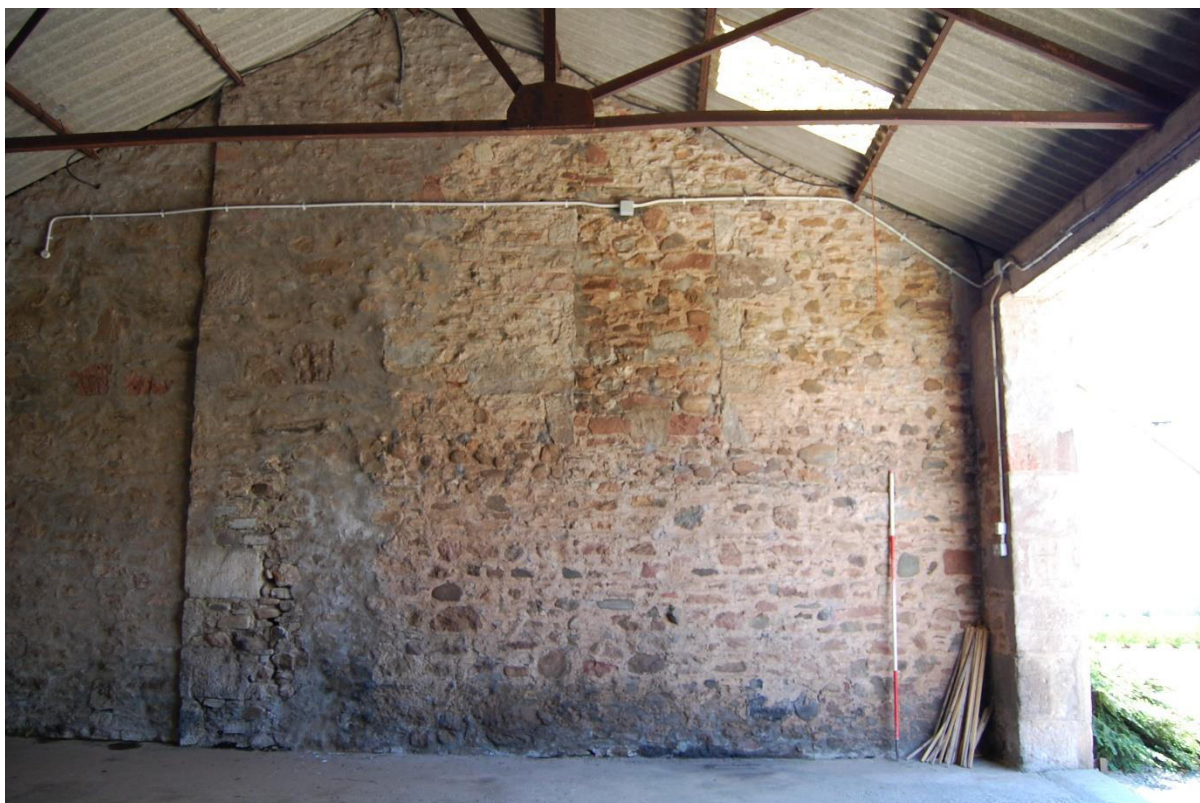
Illus 15 SE internal wall Room 6 with stonework F15 (left) and upper door D23 (centre); and the extension in Phase 3 to form larger Room 6a (left); facing SE
