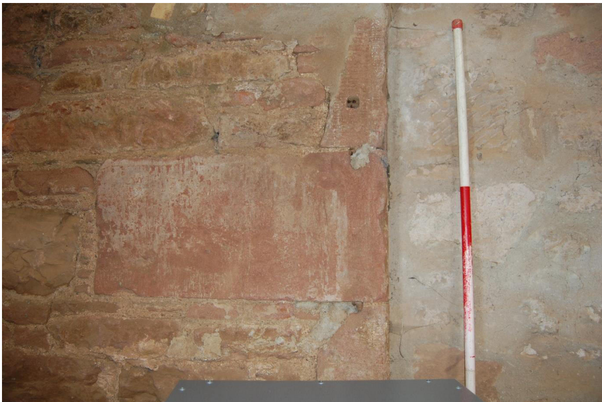
Illus 7 Room 5 exterior SE wall showing Phase 1 red sandstone blocks (left) and Phase 2 grey sandstone extension (right); facing NW
