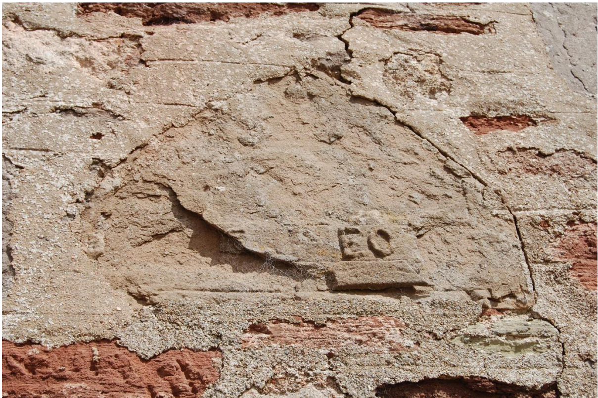
Illus 14 Armorial panel F8 is very delaminated but has lettering 'E O?'; facing NE
