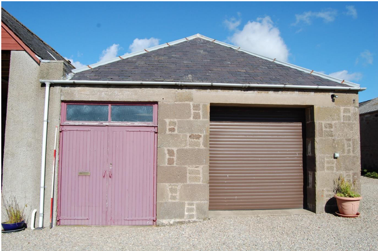
Illus 16 Room 2 SE façade showing large cart doors D1 (left) D2 (right) showing early 20 th century stonework; facing NW
