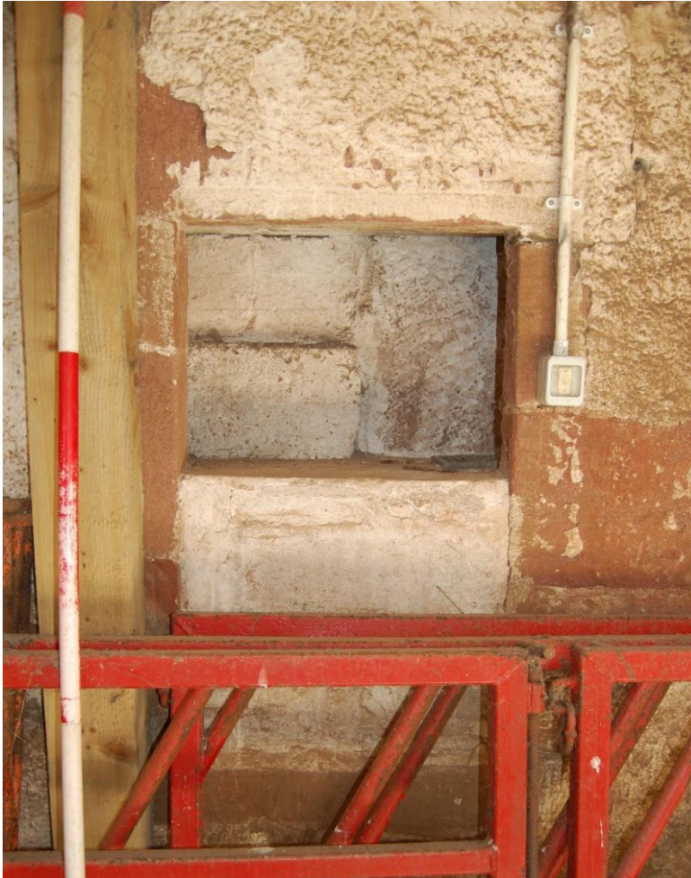
Illus 5 Room 5 SW wall; window W7 with Phase 1 red sandstone showing difficulties of access to some features and heavy whitewash on some walls (top right); facing NW
