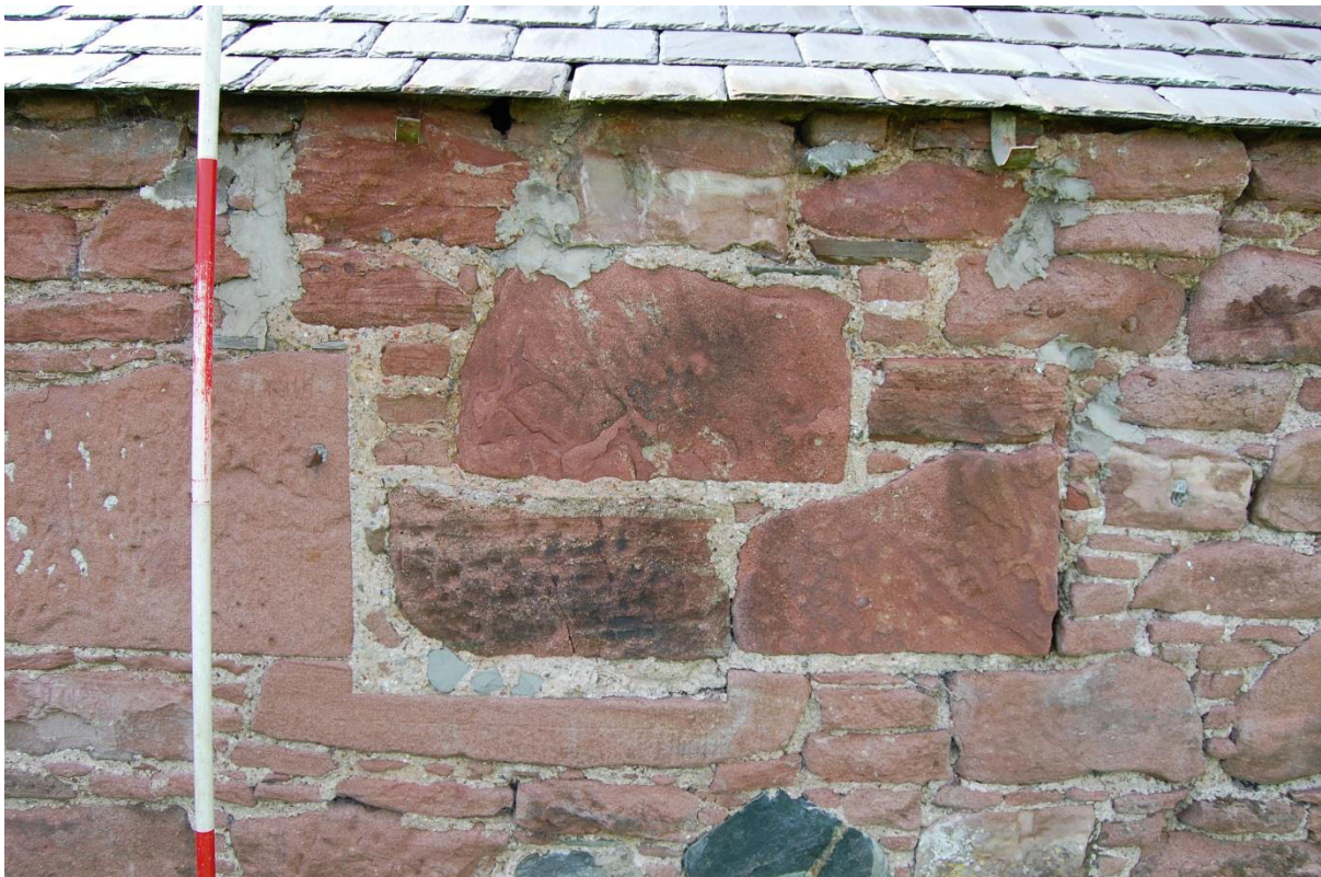
Illus 4 Red sandstone sill and jamb Phase 1 window W12; facing SW
