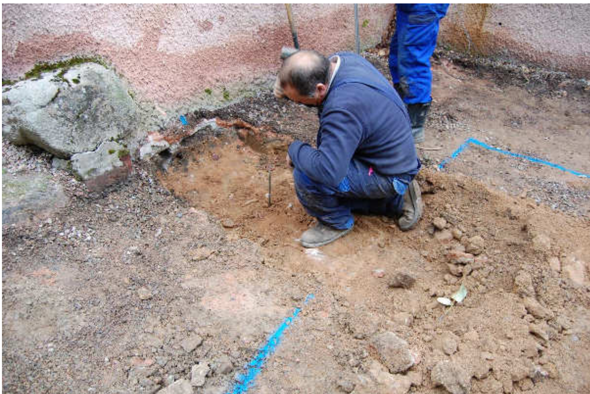
Illus 29 Shallow foundation trenches for the new extension; facing NW
