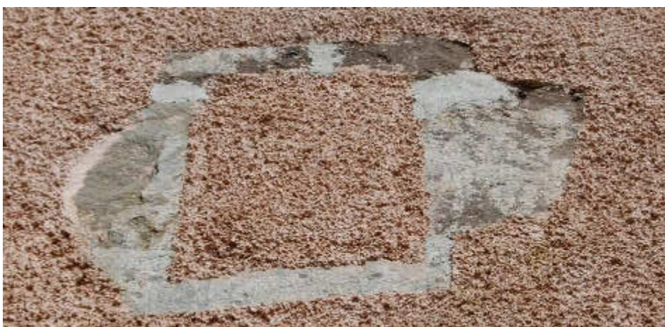
Illus 18 Blocked window W27 on first floor WSW façade; facing ENE
