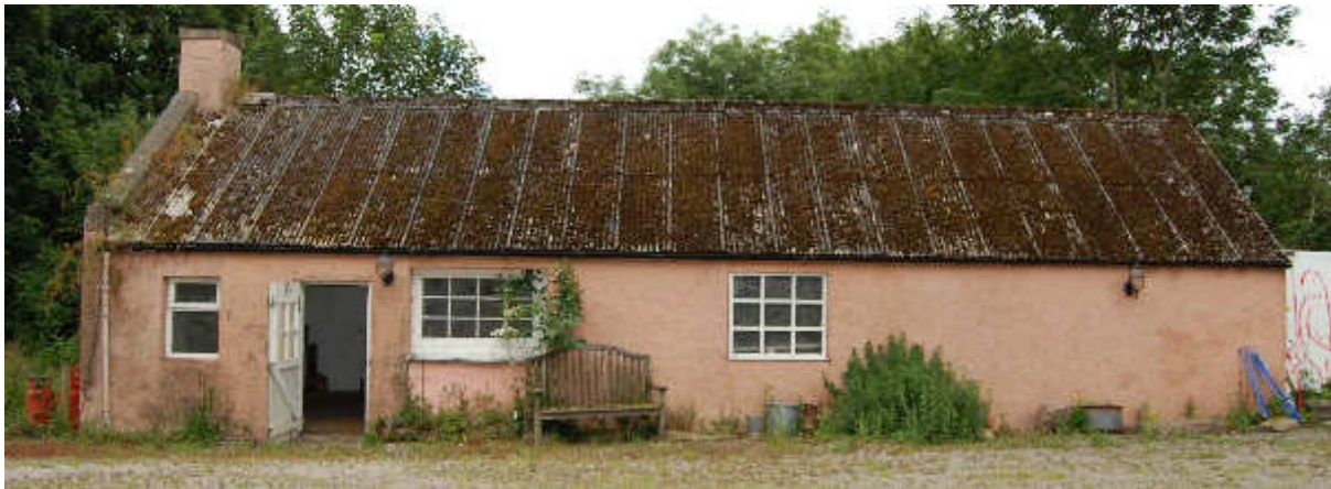
Illus 21 Building 2 WSW façade; facing ENE
