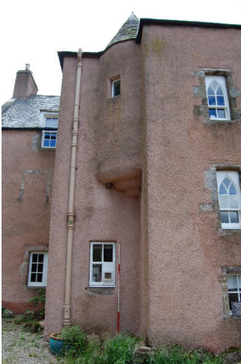
Illus 17 ENE façade showing original house (left), 19 th -century extension with windows with narrow granite sills (centre) and entrance stair probably added 19 th century (right)
