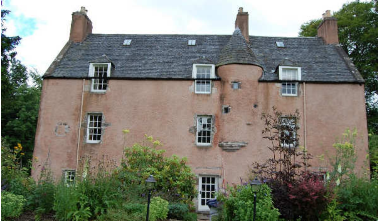
Illus 5 WSW façade with turret stair Room 10 with three small windows or shot holes (W28, 29, 30); facing ENE
