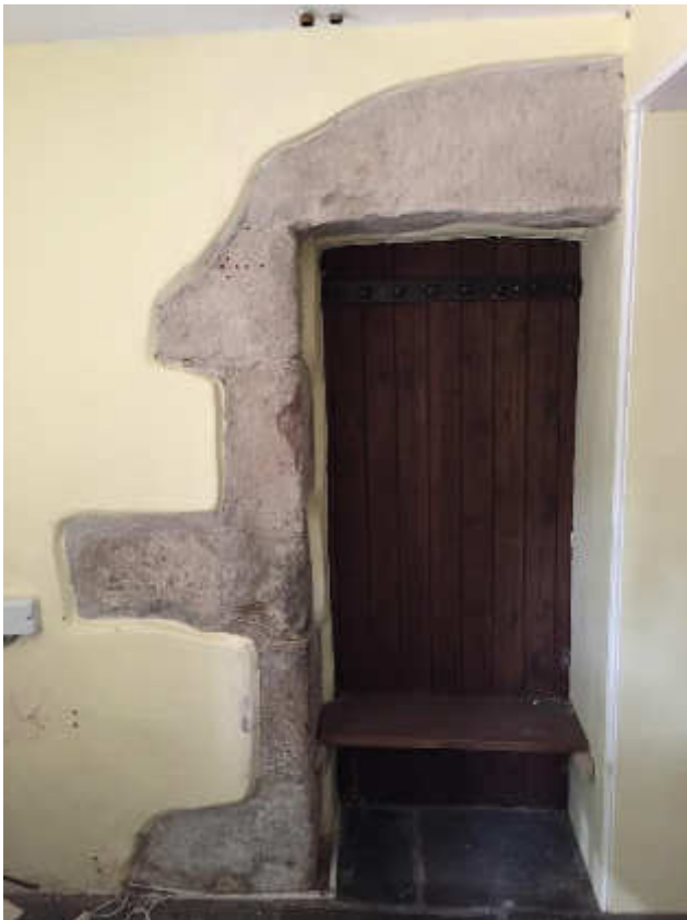
Illus 12 Door D5 the original exterior door on ENE façade with grey sandstone mouldings; facing WSW
