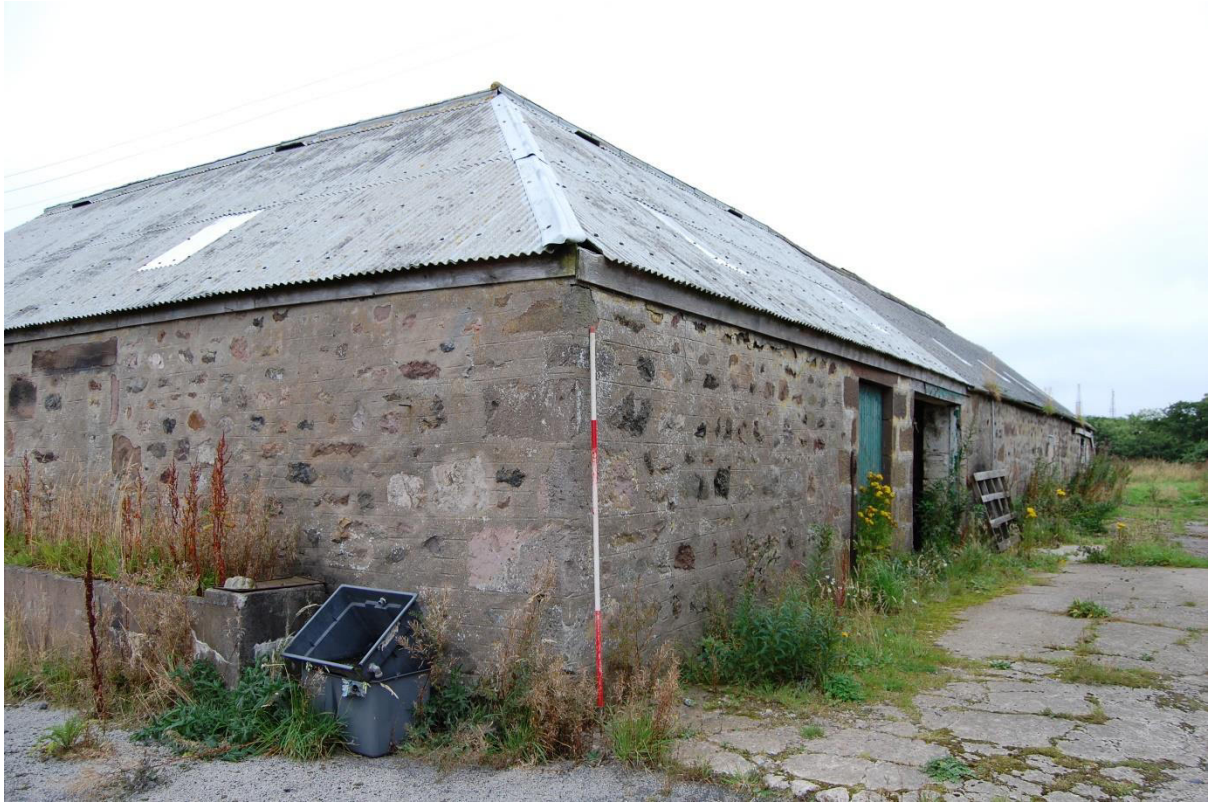
Illus 5 Building 1 E corner; facing W
