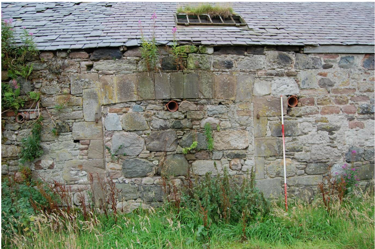
Illus 8 D14 cart door in NW wall Building 1; facing SE
