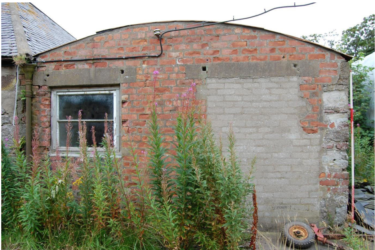
Illus 11 Building 3 W4 (left) and door D23 (right); facing NE
