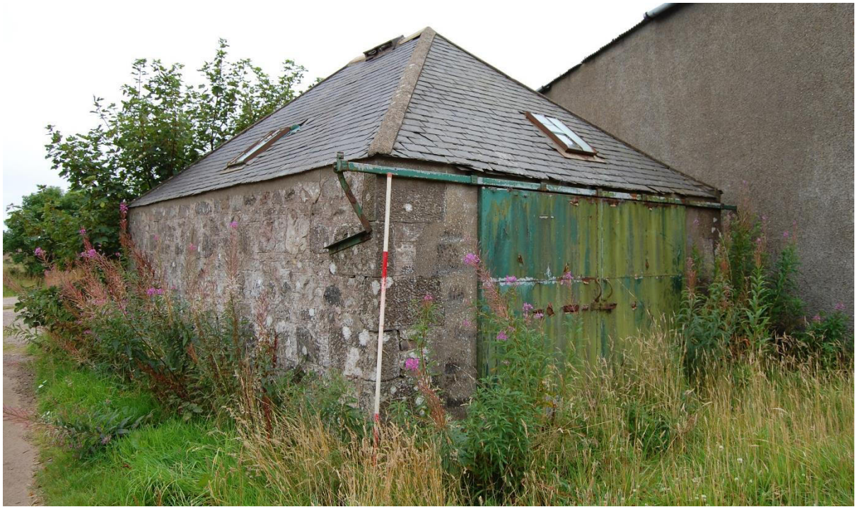
Illus 17 Building 6; facing W
