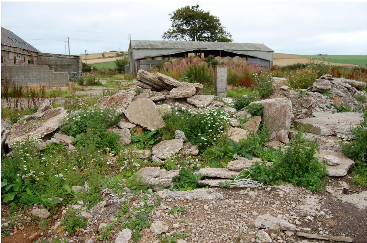
Illus 18 Building 7 (centre background) with demolished concrete structures (foreground); facing SE
