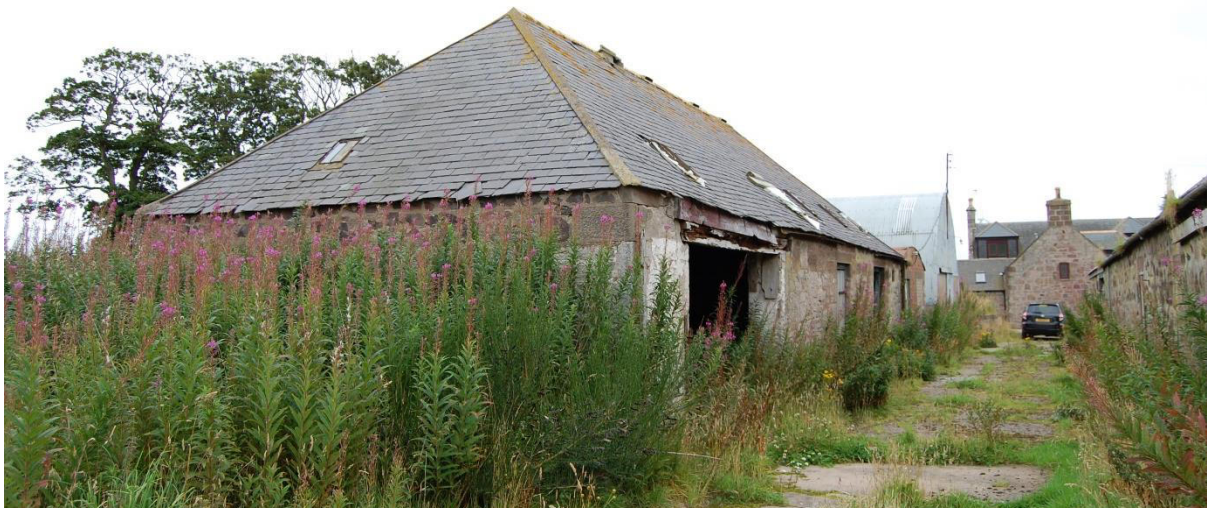
Illus 13 Building 4; facing SE
