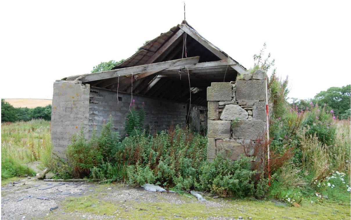
Illus 15 Building 5 SE gable with D29 showing SW wall rebuilt; facing NW
