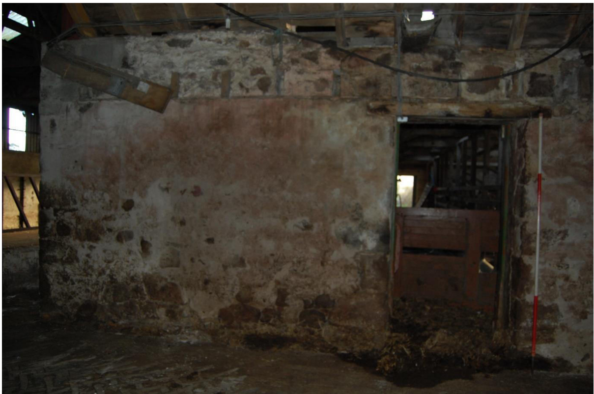
Illus 14 Shed 3 ENE wall with D3; facing ENE
