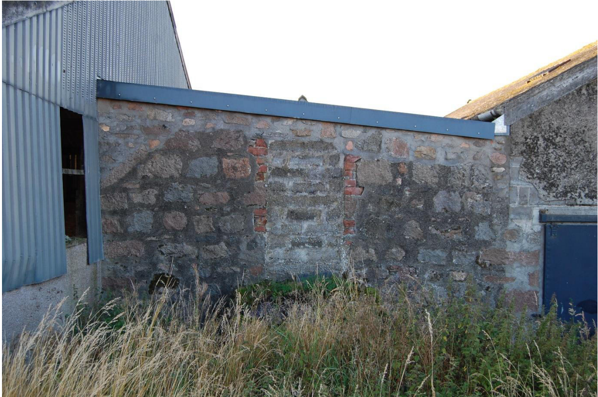
Illus 17 Shed 4 NNW wall exterior with D6; facing SSE
