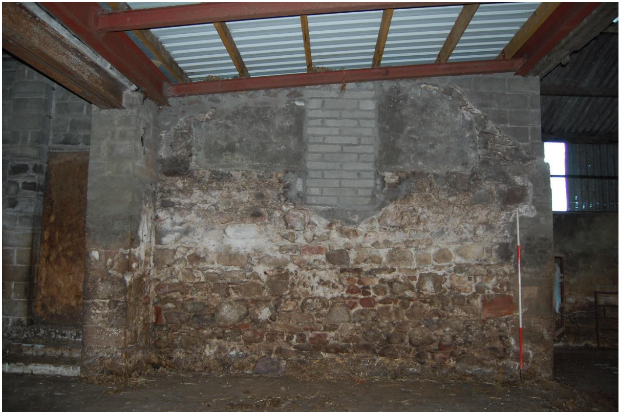
Illus 15 Shed 3 NNW wall with D6; facing NNW
