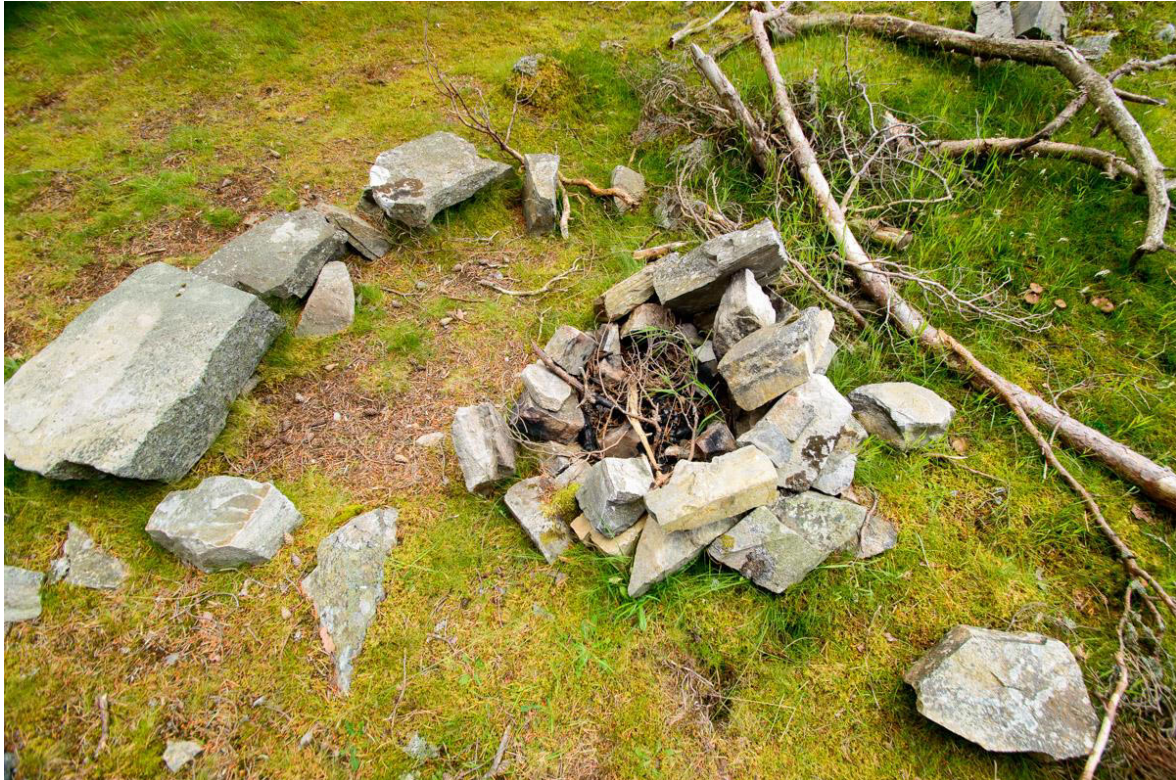
Illustration 14: Stone possibly removed from a nearby section of drystone walling for use as a makeshift hearth. Brush fires pose a threat to the estate, especially during the summer near conifer stands and plantations.
