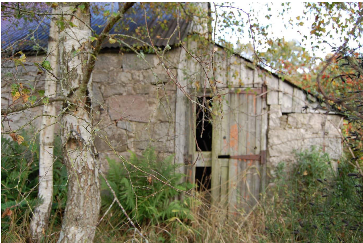
Illus 5 S façade with Room 3 lean-to (right); facing N
