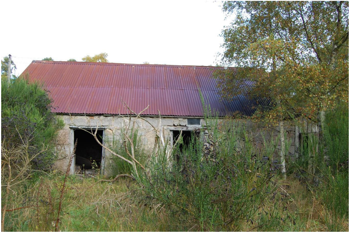
Illus 3 S façade of Rooms 1 and 2; facing N
