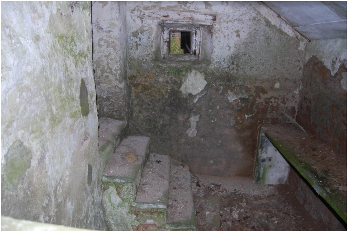
Illus 7 Room 1 interior through window W8; facing WSW
