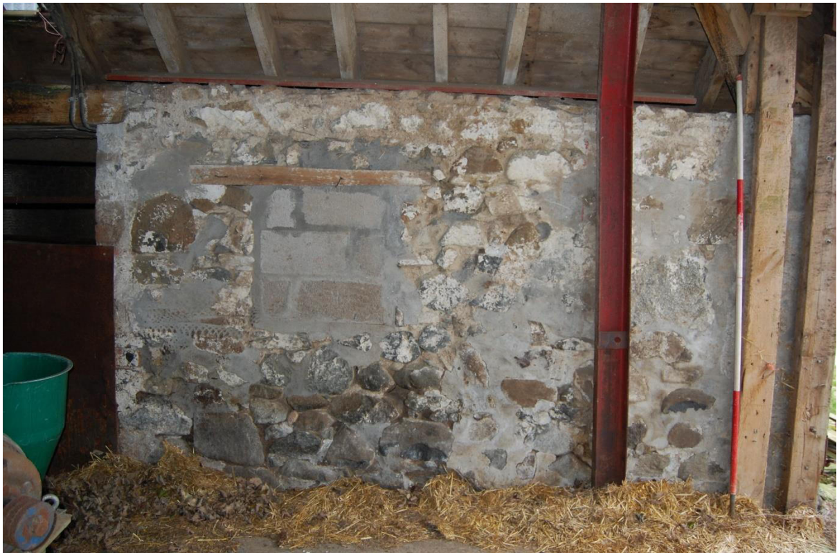
Illus 8 Room 7 W wall blocked window W13; facing WSW
