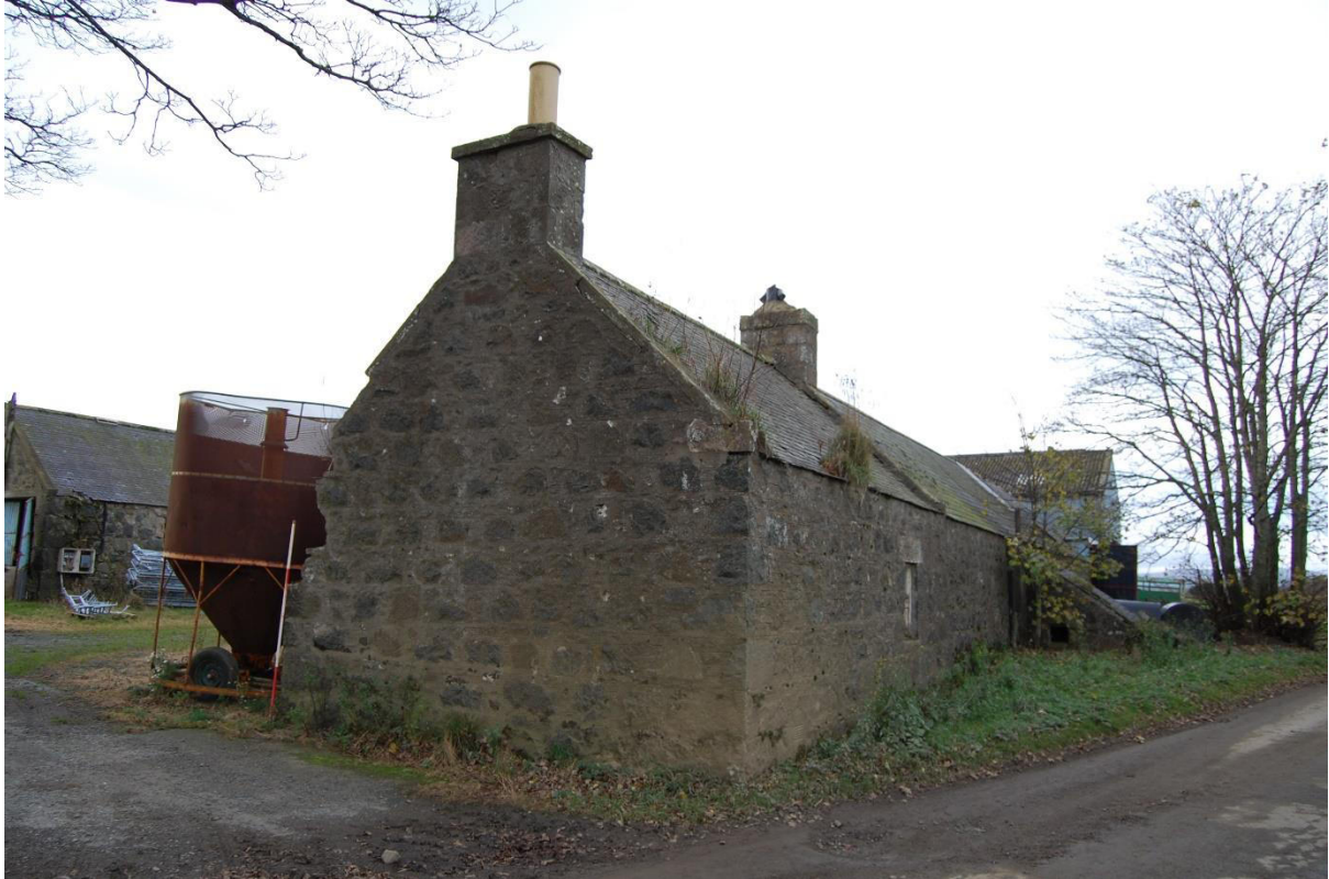
Illus 15 Phase 2 gable Room 5; facing SW
