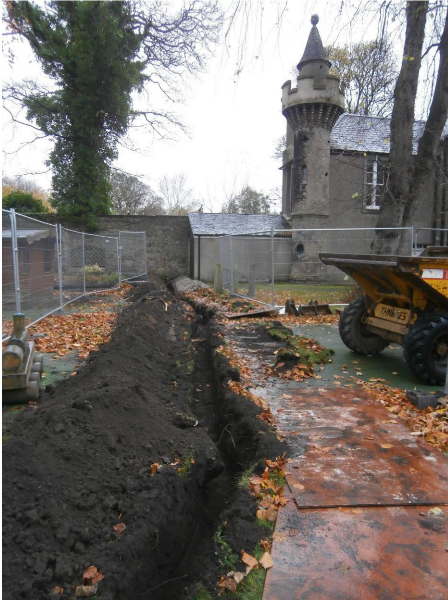
Illus 3 Trench 1 showing garden soil with 51 College Bounds (right); facing N
