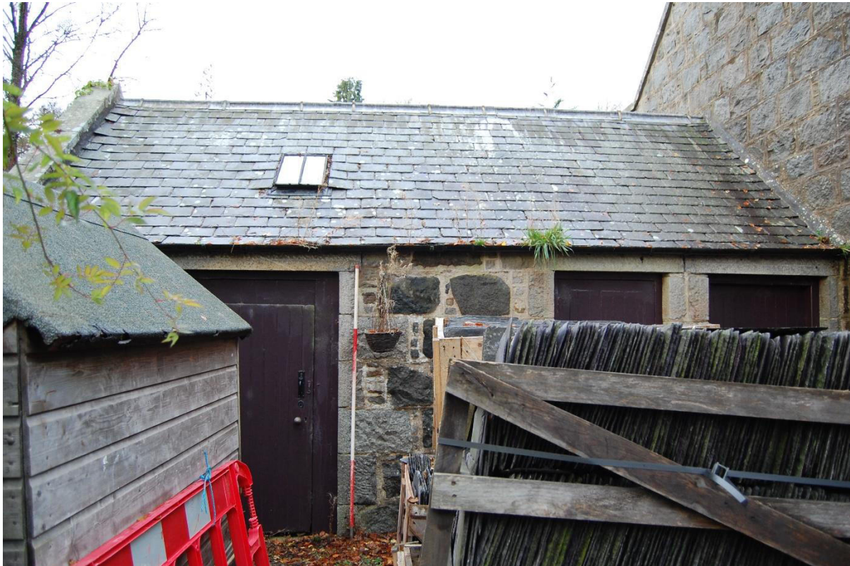
Illus 12 Room 7 E wall with D4, D5, D6; facing WSW
