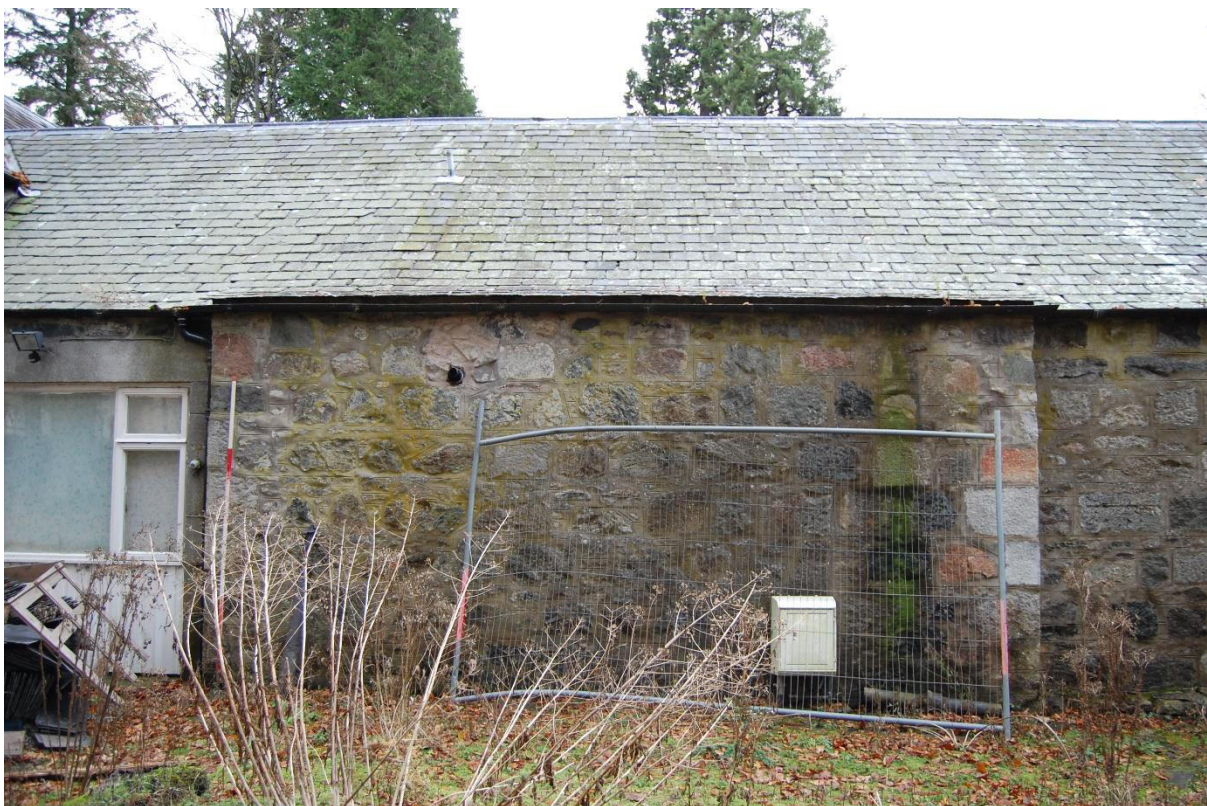
Illus 9 Room 4 N wall showing scar where building had been attached; facing SSE
