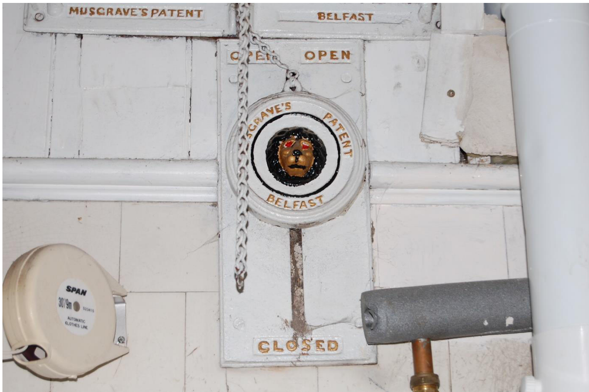
Illus 10 Room 4 N wall ventilation control 'Musgrave's patent, Belfast', facing NNW
