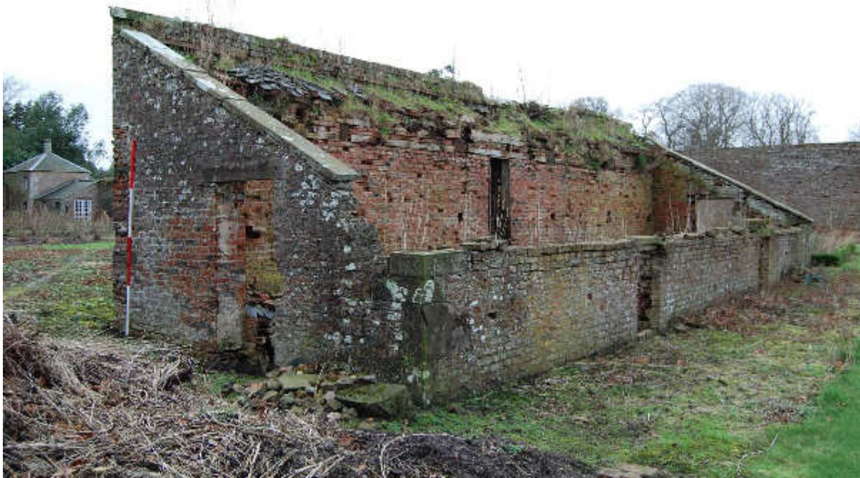
Illus 29 Building 5 from NE
