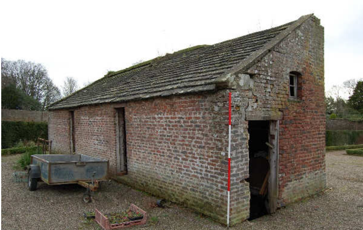
Illus 23 Building 4 from NW
