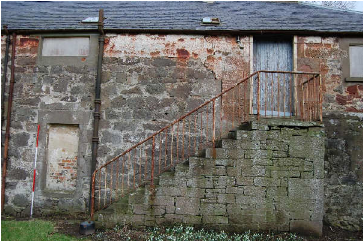
Illus 7 Phase 1 grey sandstone structure (bottom left) and Phase 2 red sandstone walls, door D4 and windows W10 (top left) and W12 (right) and sandstone steps F10 which were built in Phase 2 and reduced in length by Phase 3; facing N
