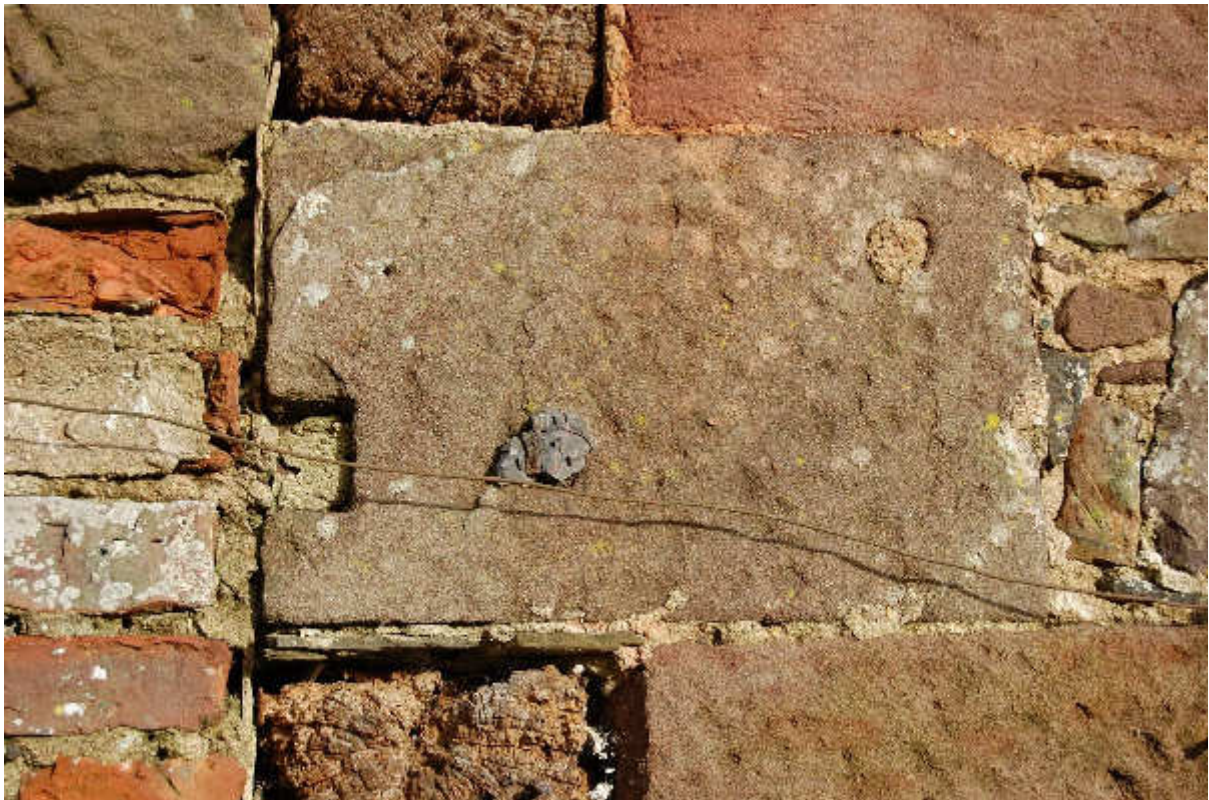
Illus 22 Building 3 reused sandstone block with notch, F27; facing N
