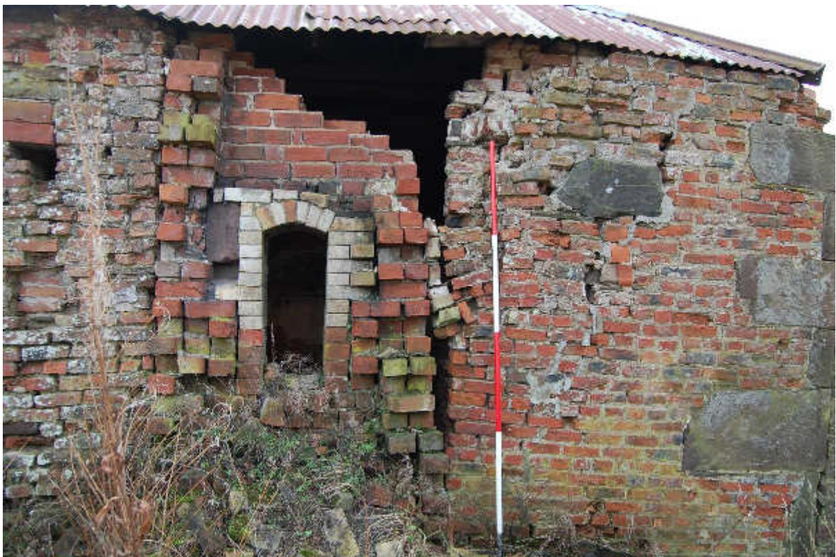
Illus 15 Building 2 Room 2 N wall with fireclay flue F16 (centre) and sandstone block quoins (right); facing S
