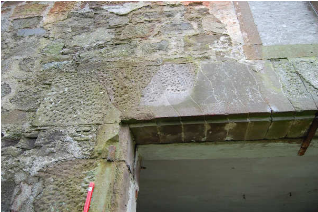
Illus 4 Building 1 N wall D2 detail of E jamb of pecked sandstone and joggle jointed lintel; facing S
