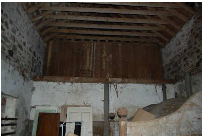
Illus 11 Building 1 Room 3 showing wooden partition wall to create a double height room and domestic accommodation on first floor on other side of partition; facing W
