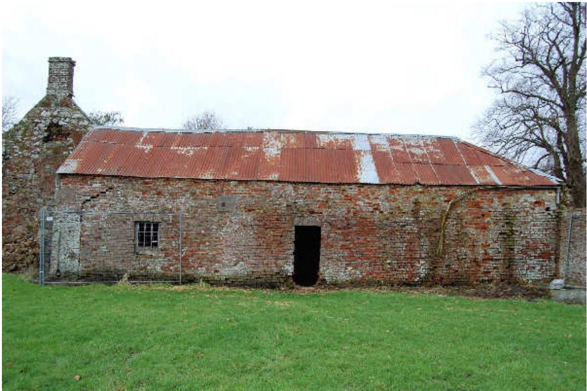
Illus 14 Building 2 E wall; facing W
