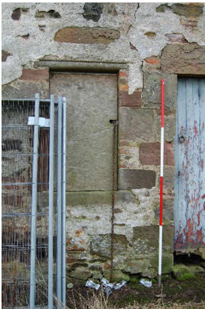
Illus 3 Building 1 S wall W9 with sandstone roll moulding reused for lintel; facing N
