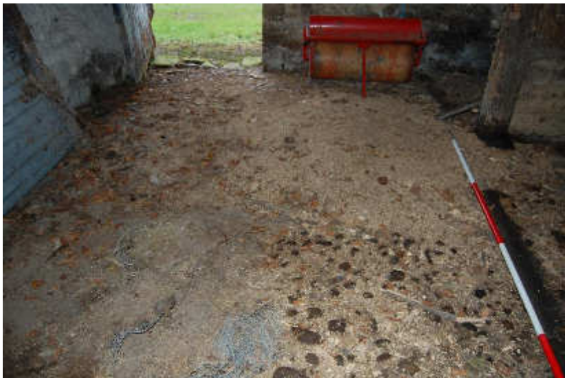
Illus 10 Building 1 Room 1 cobbled waterwashed stone floor; facing N
