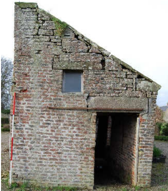
Illus 26 Building 4 E wall with D10 and W29; facing W
