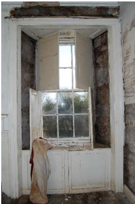
Illus 38 Room 28 W15 showing stonework around the window and original window seat and cupboard and wooden shutters in situ; facing E
