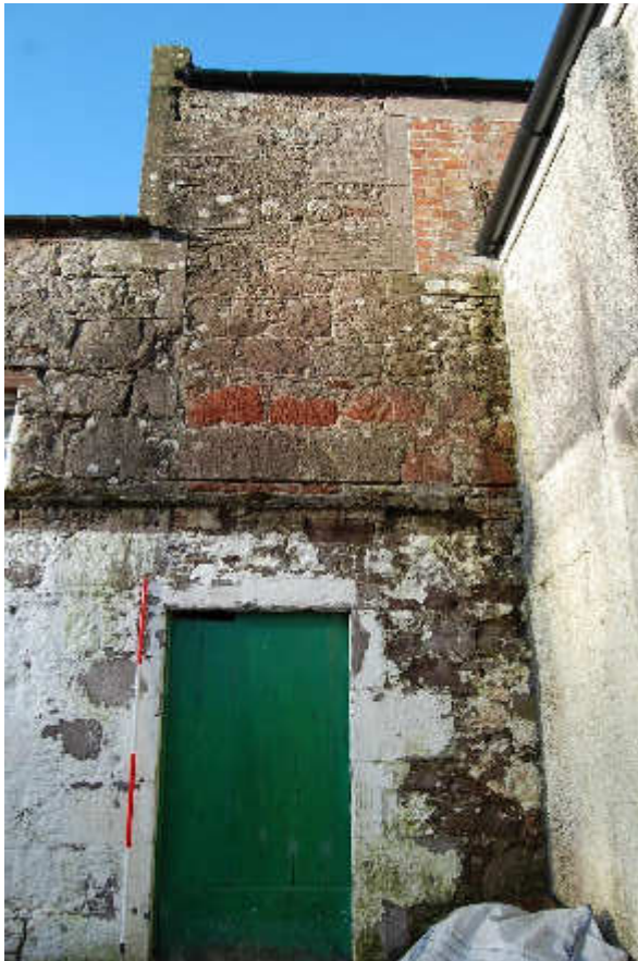
Illus 28 Room 21 door D8 with blocked window W37 (top right) showing junction between Phase 2 E wing (left) and Phase 3 (right); facing W
