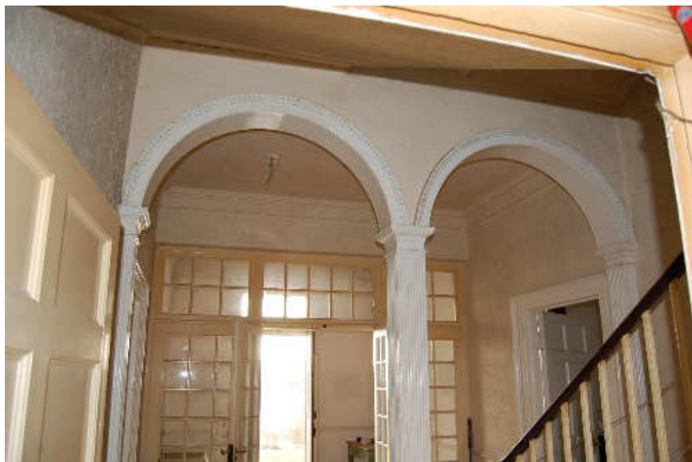
Illus 17 Arches on N side Room 10 between hallway and stairs; facing SSW
