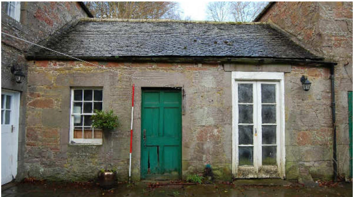
Illus 36 Room 27 S wall W61, D15 showing tooled sandstone lintels and mouldings with D16 (right) with newer sandstone lintel inserted when door inserted; facing N
