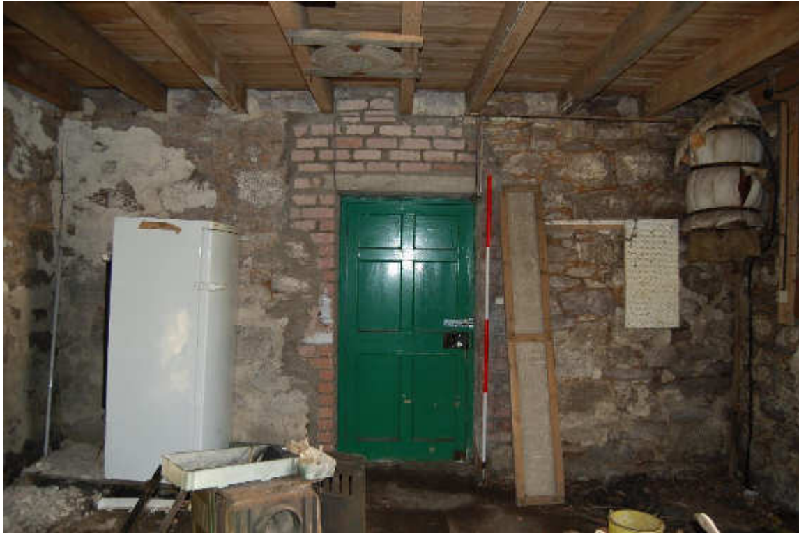
Illus 25 Room 19 E wall showing D7 with rebuilt surround in brick' facing E
