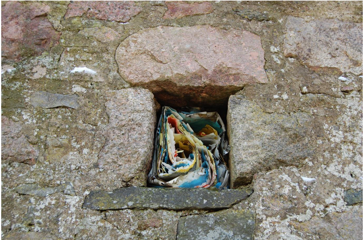
Illus 10 Room 3 exterior aperture F12; facing E
