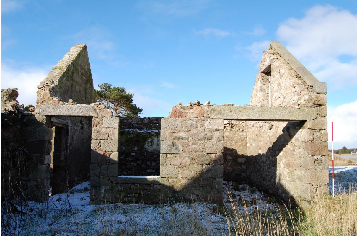
Illus 7 Rooms 1 and 2 E wall D7, W7, D8; facing W
