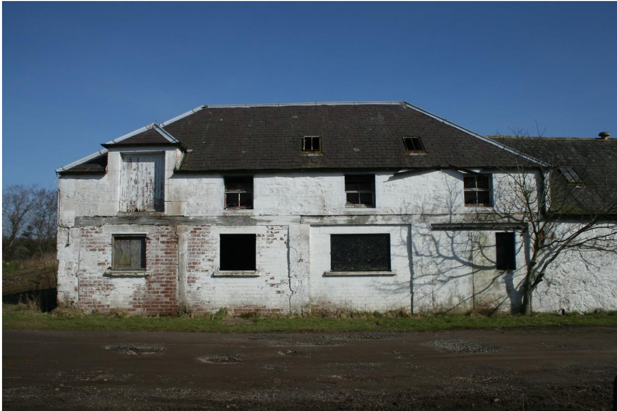
Illus 6 Building 1 W wall N end four cart doors D16-D19 infilled and with smaller apertures opened; facing E
