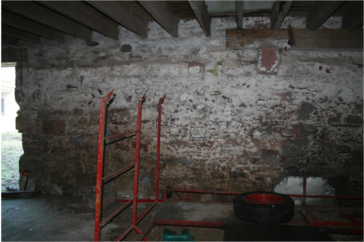
Illus 8 Building 1 Room 7 N wall showing smaller corbels (left) and larger corbel supporting current roof timbers (right)
