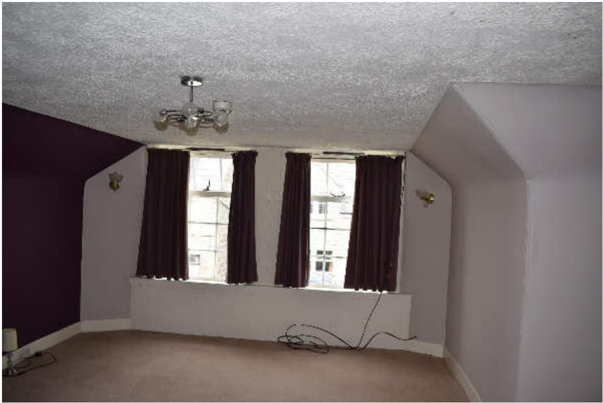
Illus 6 Phase 1 NW wall W25 and W26
