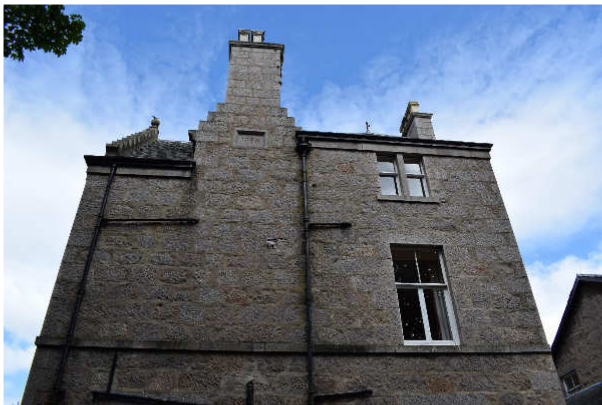
Illus 8 Phase 2 hotel SE façade with 1874 date stone; facing
