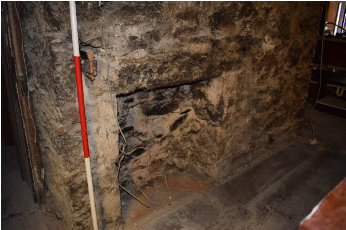
Illus 4 Fireplace F19 in Phase 1 room 27; facing N
