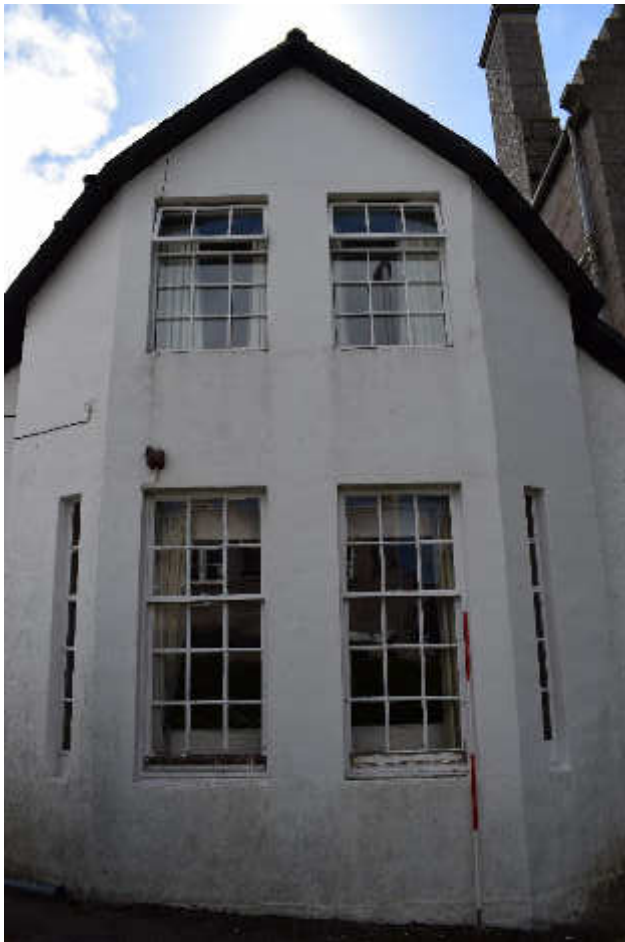
Illus 2 Phase 1 NW façade with windows W25-W30; facing SE
