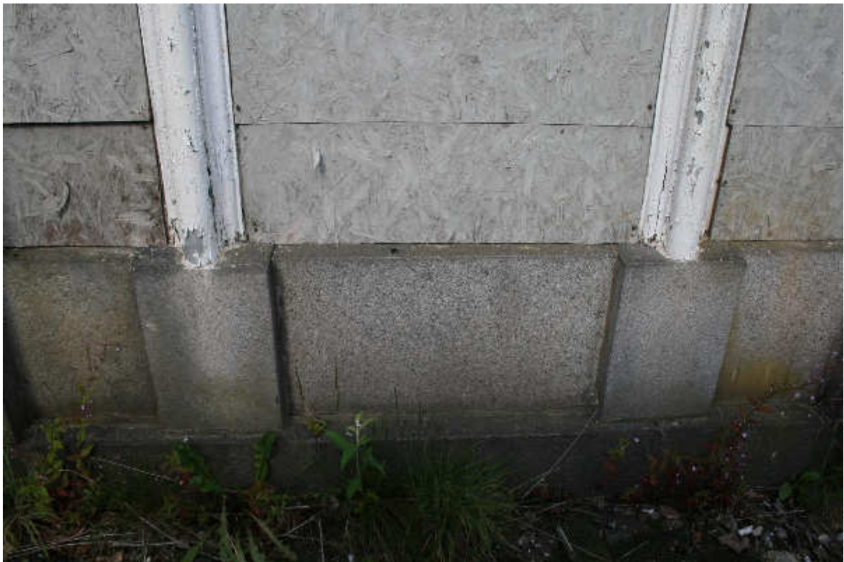
Illus 9 Granite base course under W33; facing W
