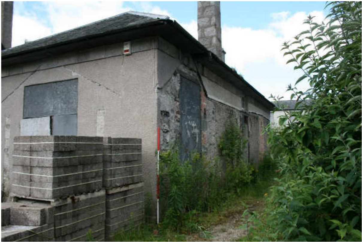
Illus 16 Building 1 NE corner; the 3 rd Edition OS map shows an extension to this façade which has since been removed; facing WSW
