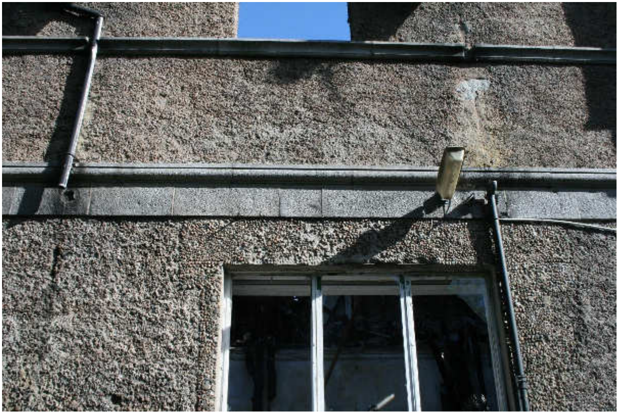
Illus 10 Granite dividing band course with W24 below and W20 above; facing N
