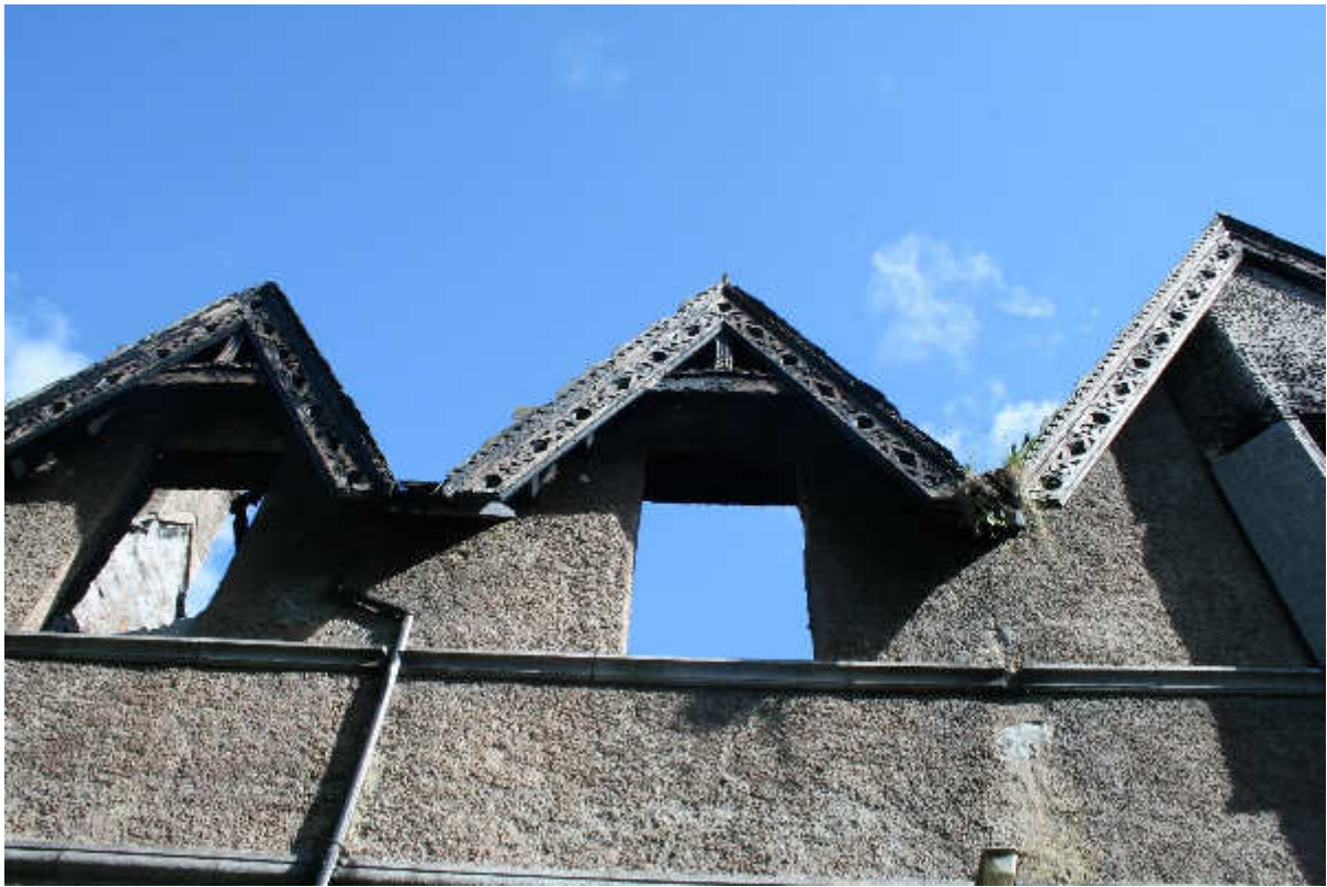
Illus 8 Building 1 S façade with decorative pierced timber bargeboards above gablets; facing N
