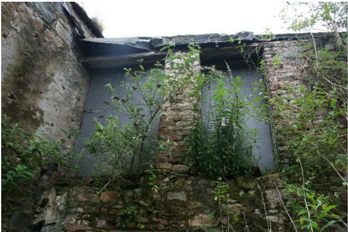
Illus 21 Building 2 Room 5 E wall D7 (left) D9 (right); facing W
