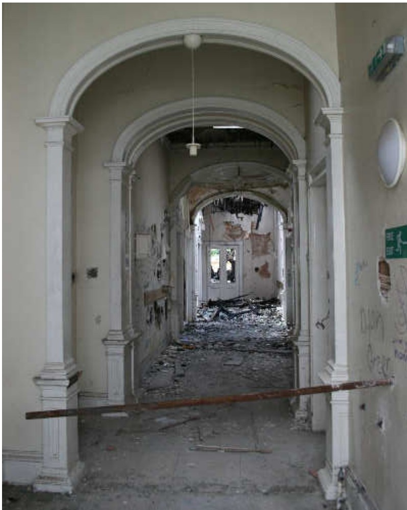
Illus 15 View into building through D5; facing S
