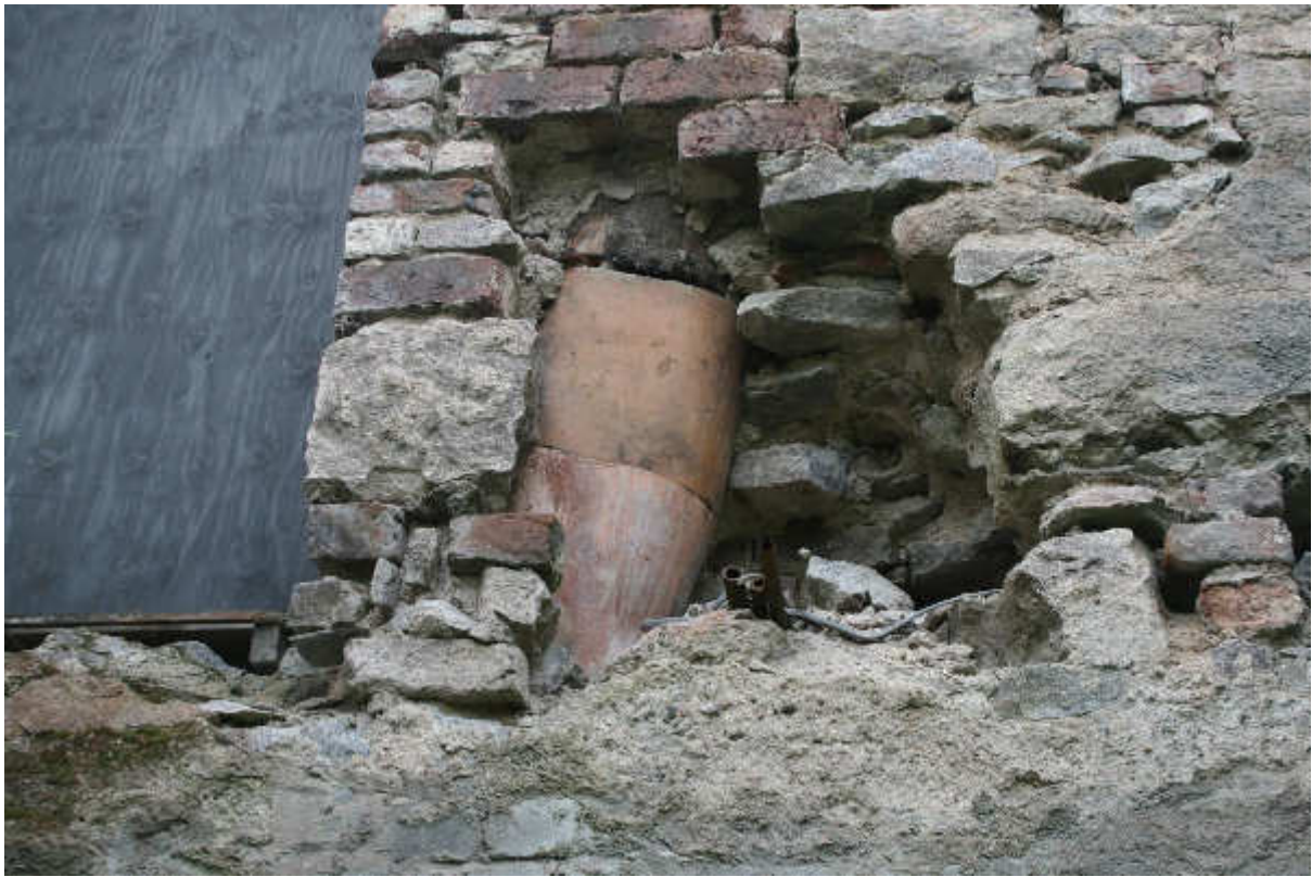
Illus 20 Building 2 N wall Room 8 ceramic flue F17; facing S
