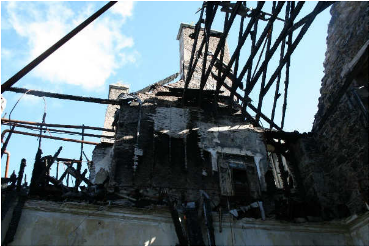
Illus 14 Interior through W24 showing fireplace F7 with chimney F1 above and burnt roof timbers; facing NNE
