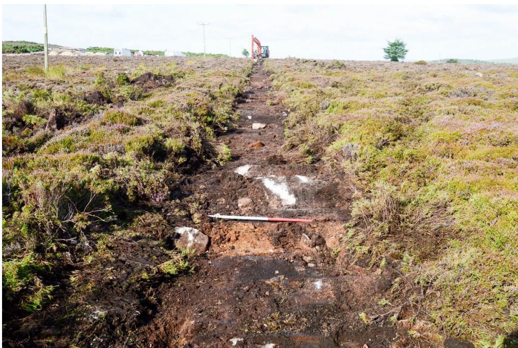
Illus 5 West facing view of corridor during topsoil removal.
