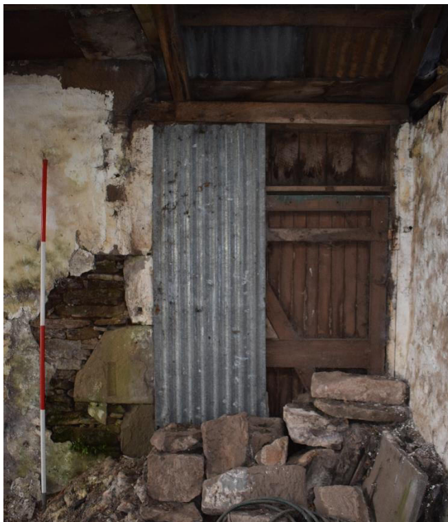
Illus 23 Sandstone quoins forming NW corner Room 6 (left) and E wall Room 2 (right); this wood door was inserted in the void and the room enclosed and roofed in Phase 2 forming Room 13; facing SSE
