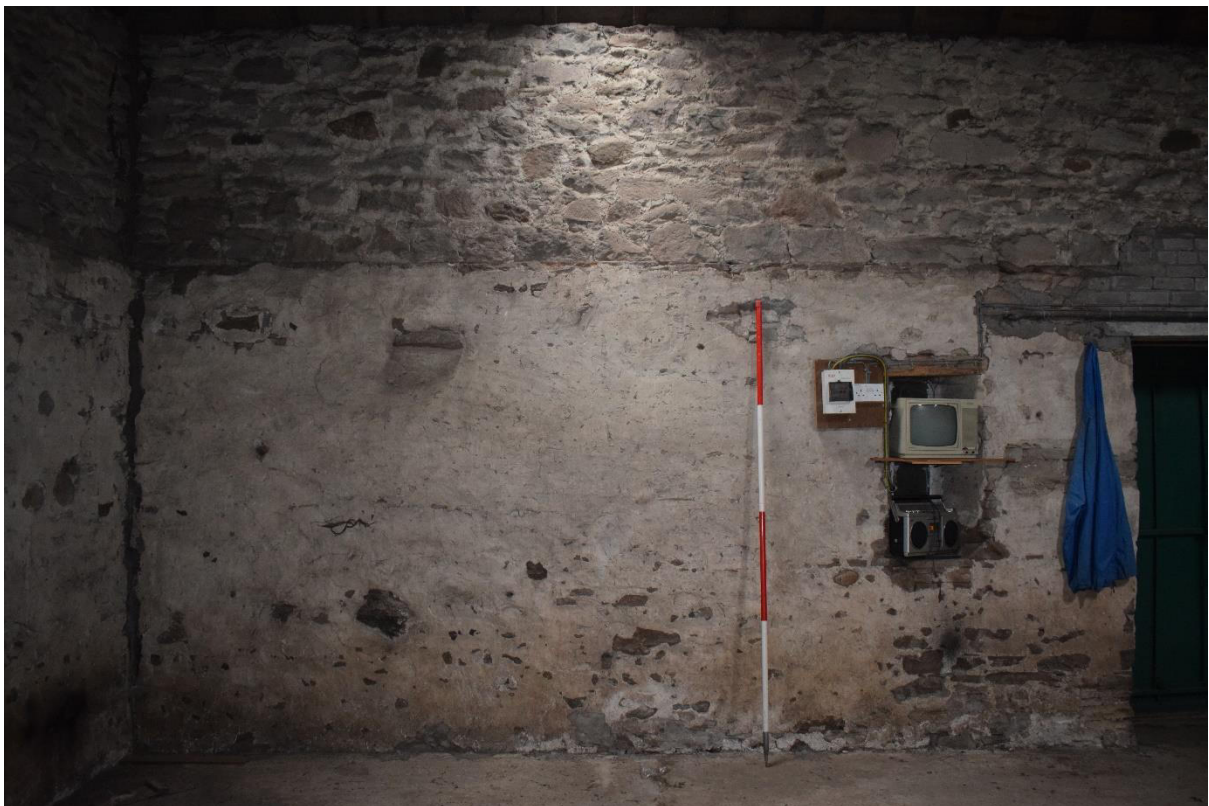
Illus 25 Phase 1 Room 9 W wall showing original height of walls, corbels F6 (centre), window W8 and D18 (right). The stone at the top has been added when the roof height was raised and new roof added; facing W
