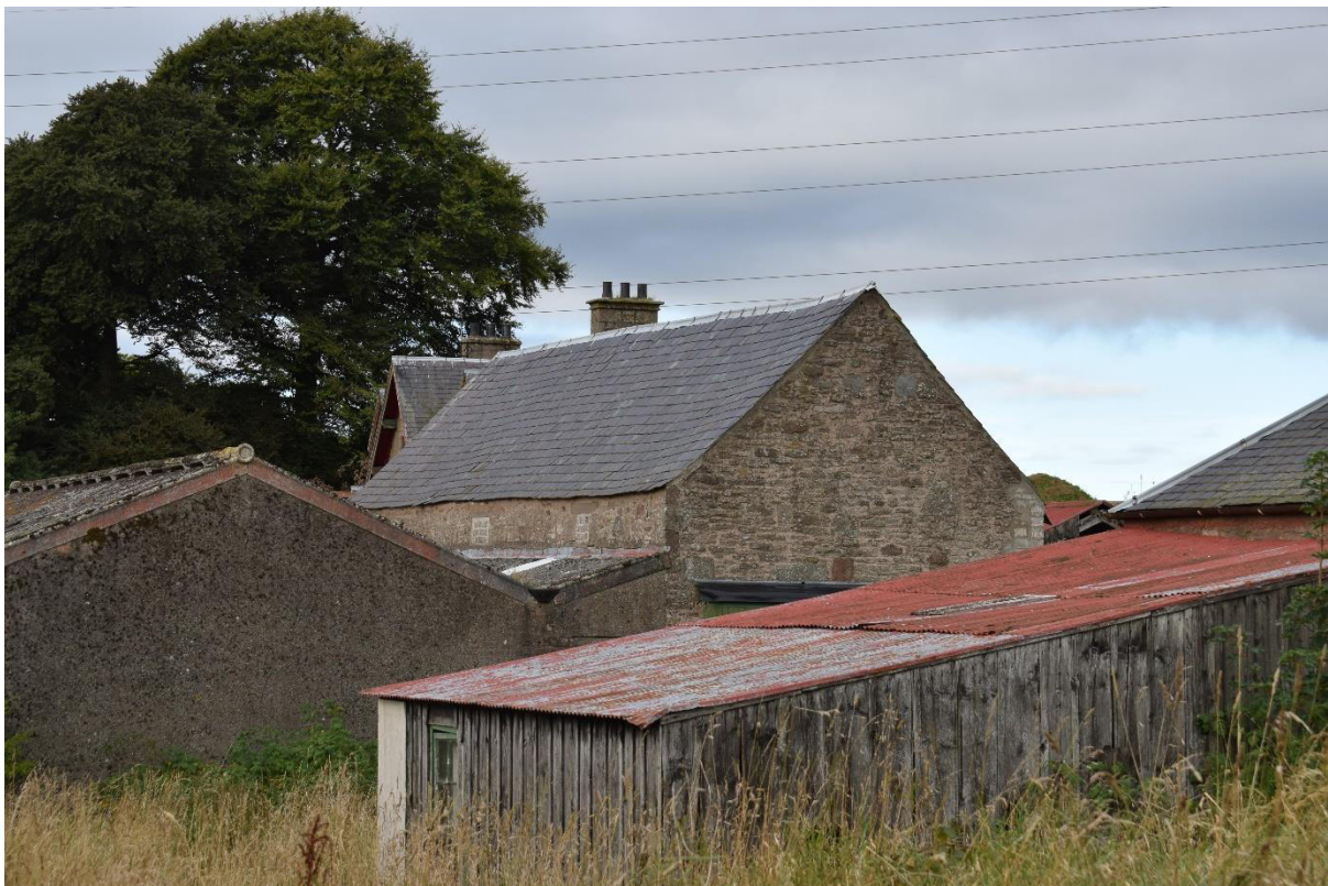
Illus 19 Room 6 (centre) view of S wall (left) with upper windows W11, W12, W13 (l-r) and E gable (right); facing WNW
