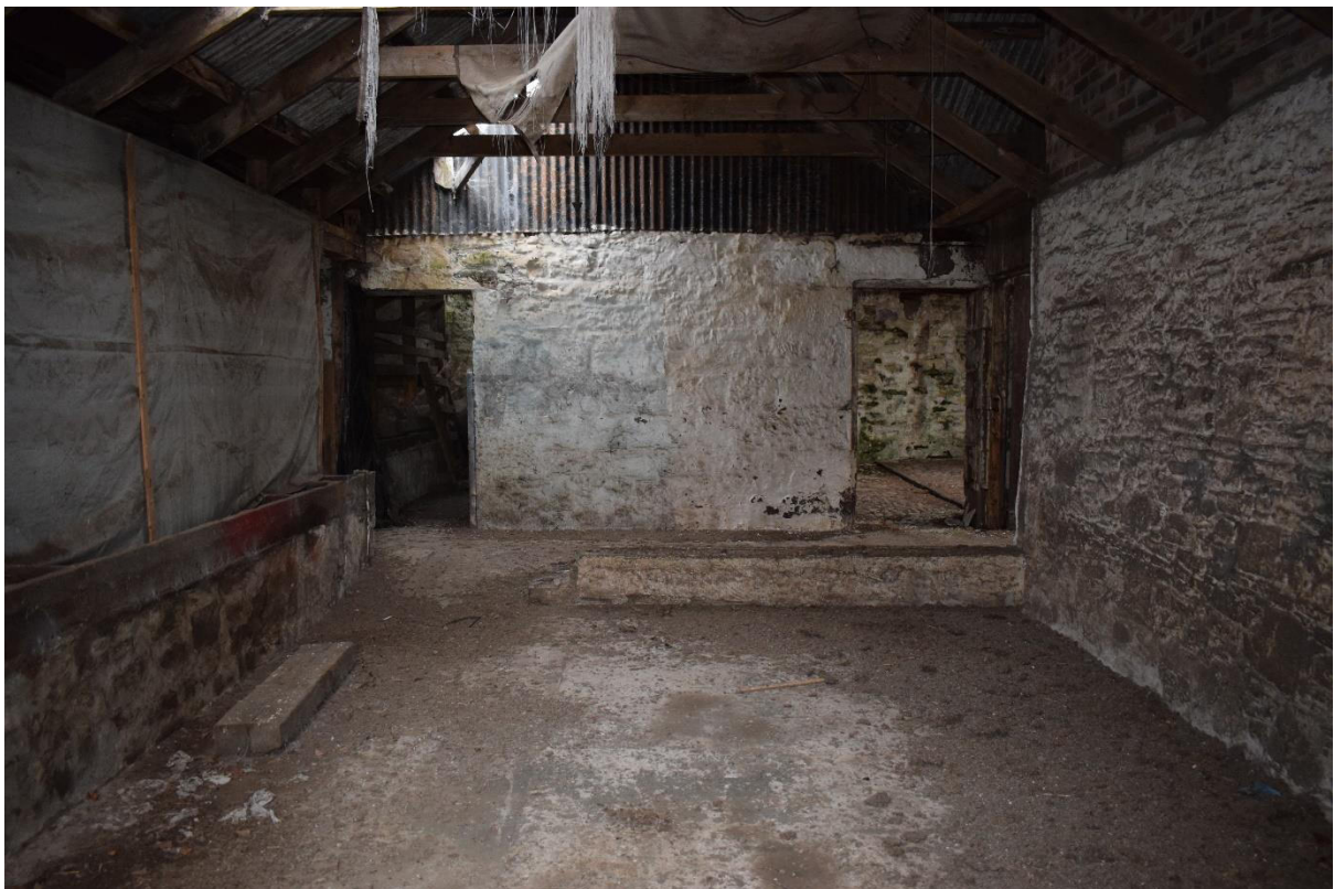
Illus 11 Phase 1 S wall Room 4 (centre, D2 left, D3 right) and courtyard Room 1 later enclosed in Phase 2. The low wall on the left is the slighted W wall of Room 2; facing NNW
