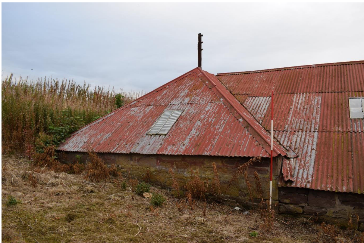
Illus 9 West wall Phase 1 Room 1 showing Phase 2 Room 1 butted on; facing ENE
