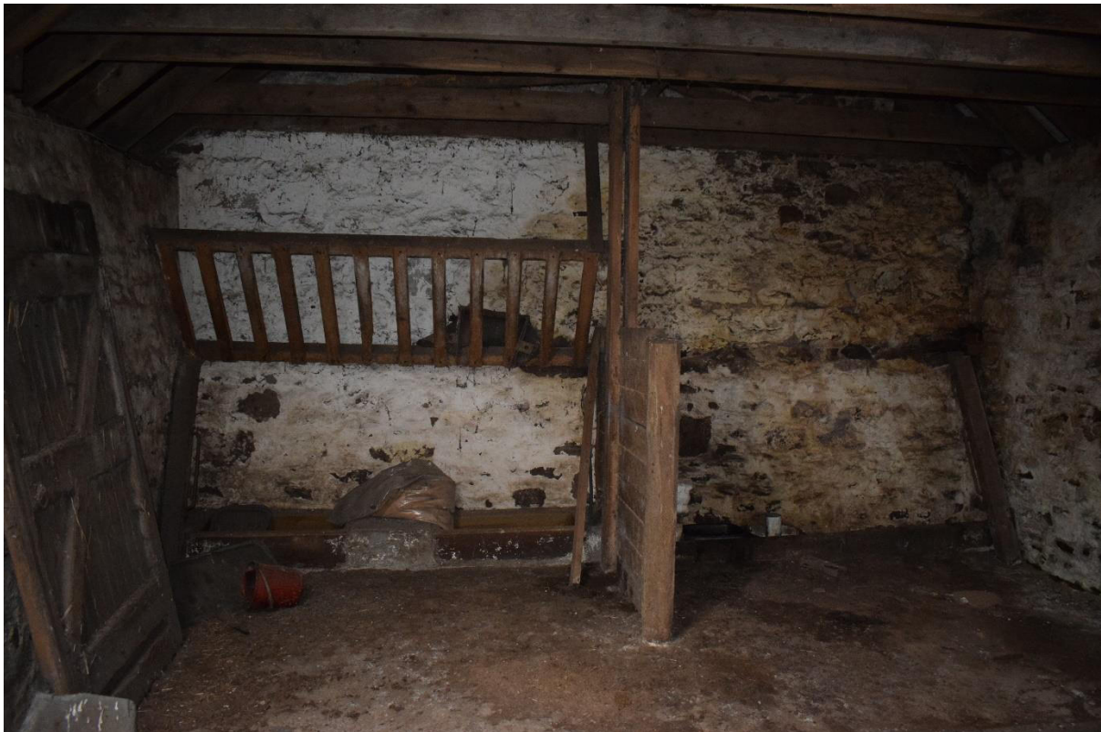
Illus 15 Phase 1 Room 4 wooden stall partitions, F11 and base for stoneware troughs F12 below; facing W
