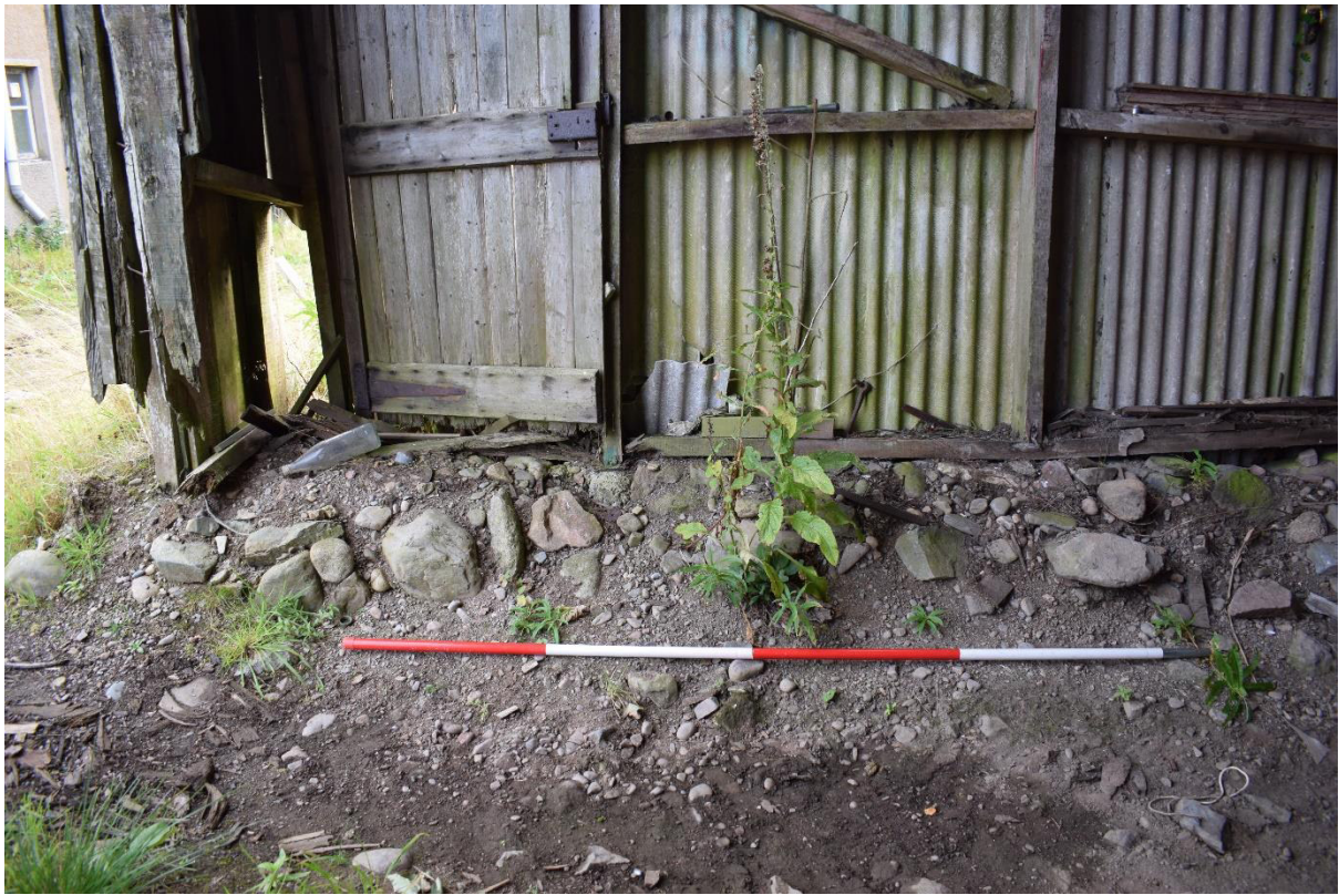
Illus 17 Building 2 stone foundation F2 under E wall; facing E
