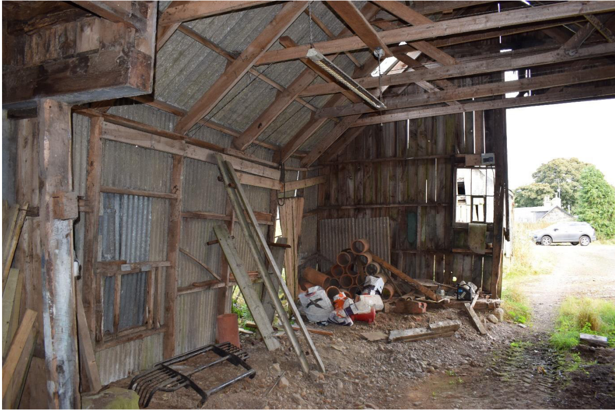
Illus 19 Building 2 extension constructed from asbestos cement roofing panels; facing NNW
