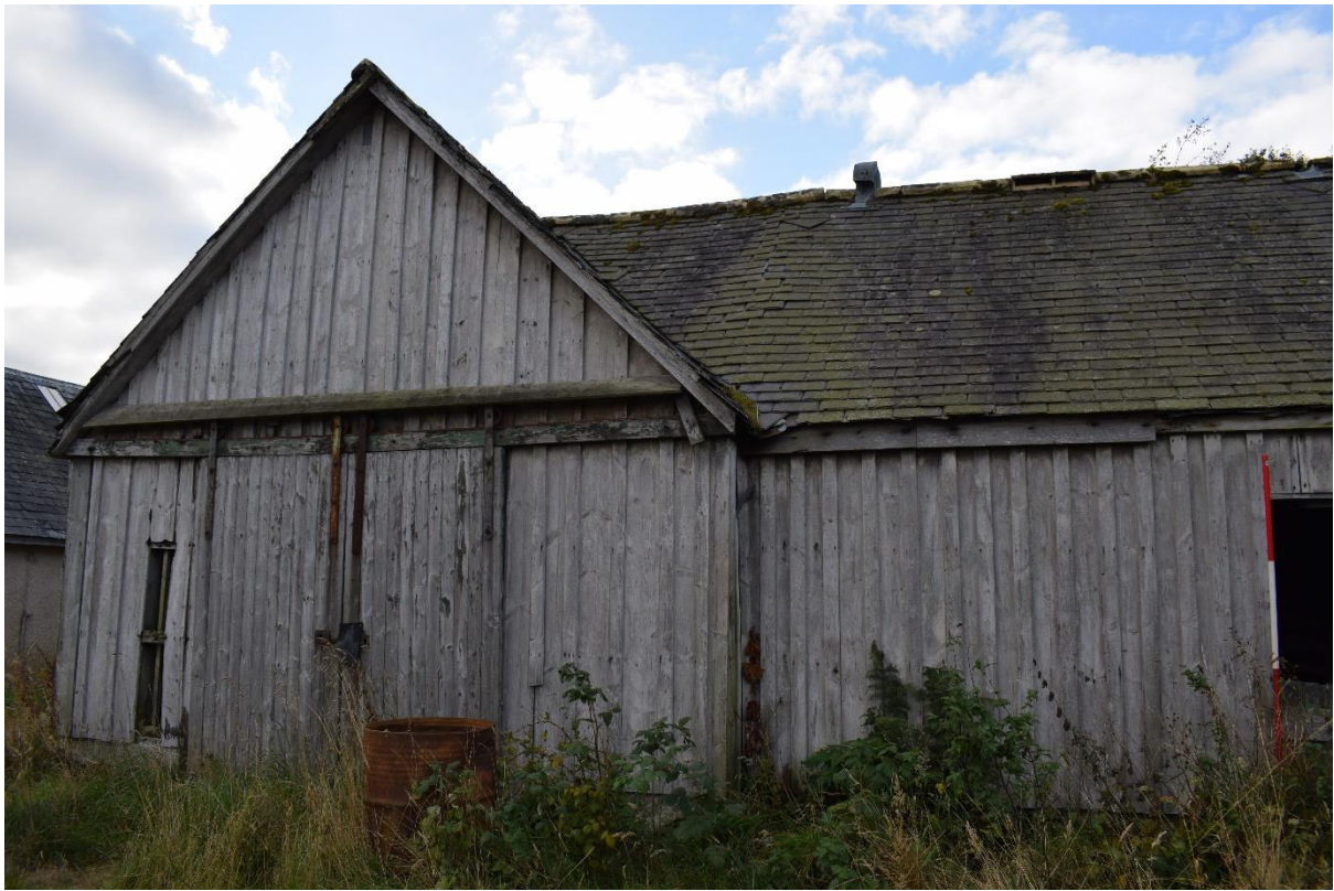
Illus 5 Building 1 N wall showing wood plank construction; facing SSE
