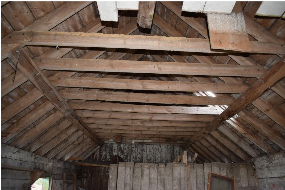
Illus 10 Building 1 wooden roof timbers from D7; facing E
