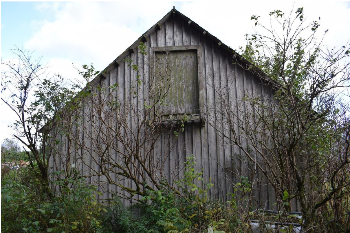
Illus 14 Building 2 S gable with first floor D9; facing N
