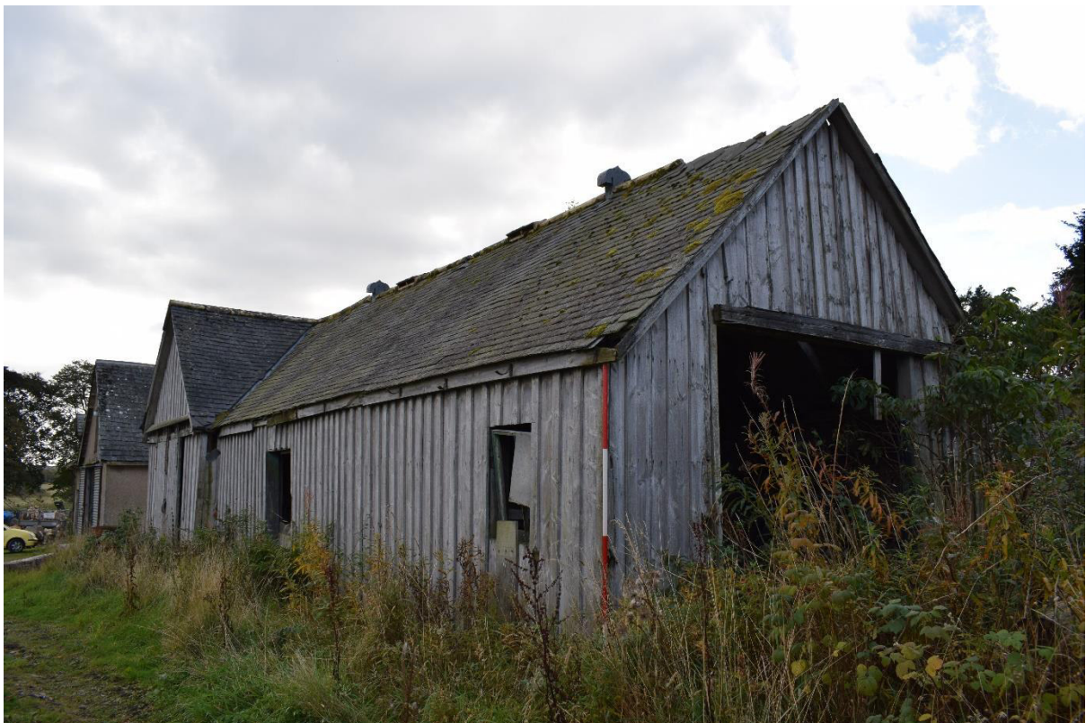
Illus 6 Building 1 from NW showing D7 (right); facing ESE
