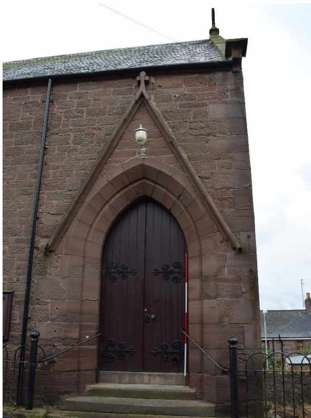
Illus 7 Principal doorway in N wall (D1) showing a recessed pointed arch doorway with decorative pediment above; facing SSE
