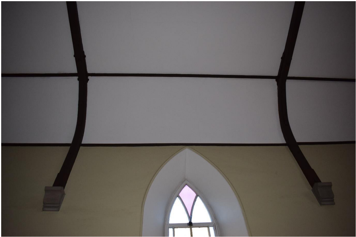
Illus 11 W2 (below) with mock wooden beams and corbels (F5, left; F6, right); facing NNW
