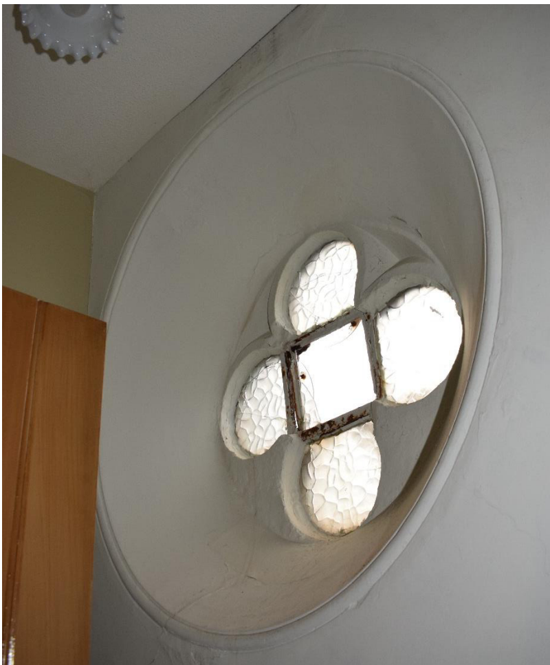
Illus 12 Phase 1 quatrefoil window W9 built into Phase 2 toilet; facing SE.
